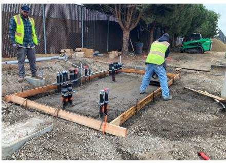
**Electrical Conduit Stub-ups at Electrical Pad**
