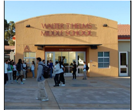
Helms Middle School $53 million Reconstruction completed with Measure D funds.
