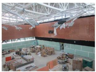
Building B - Gym: Perforated wood panels at gym walls
