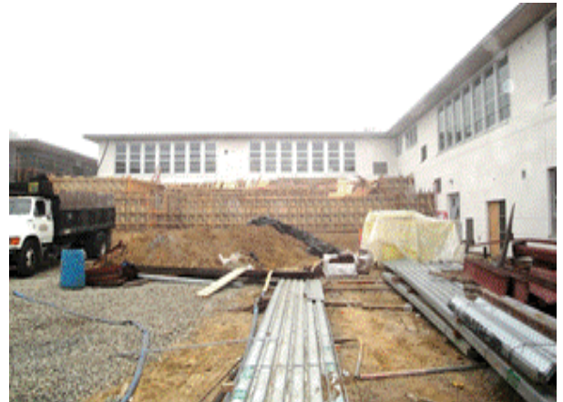
Building A - Complete forms for planter walls and seat benches
