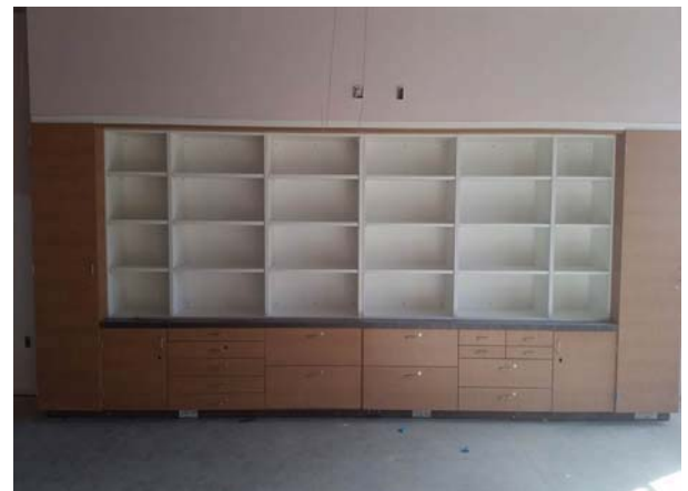
Building Classroom Casework Installation
