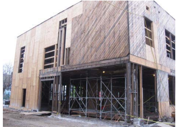
North Building - Replacement Diagonal Sheathing
