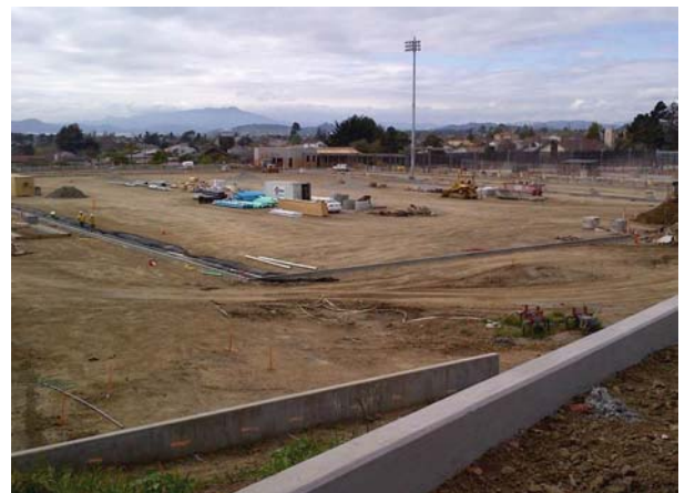
Field Drain Installation
