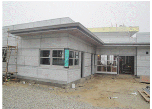
Building B - Storefront and window installation
