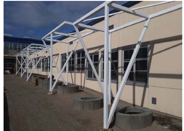
Building C - Exterior Classroom Shade Structure Painting
