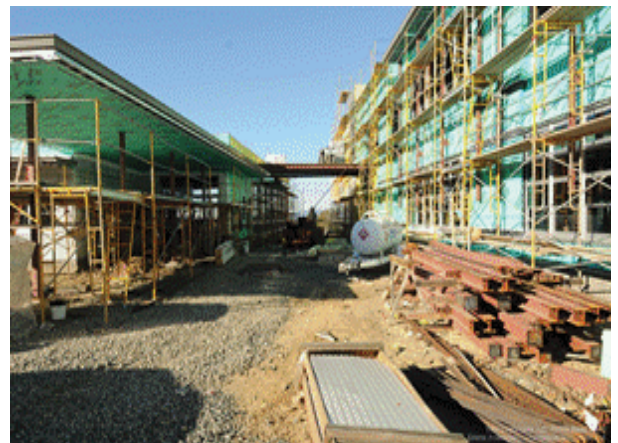
Building B & C - Sheetrock
