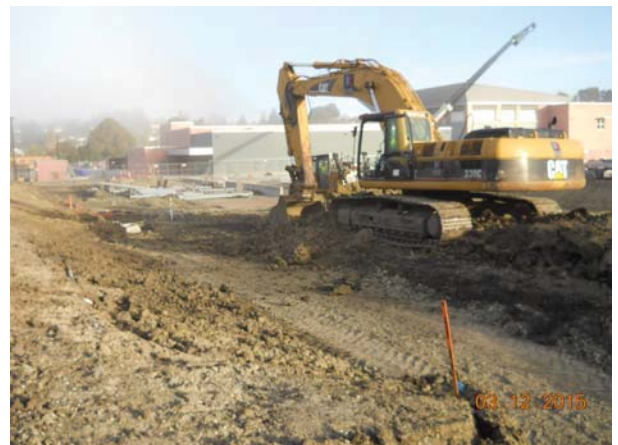
Grading Parking Lot
