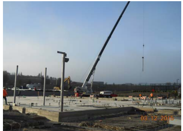
Structural Steel Erection
