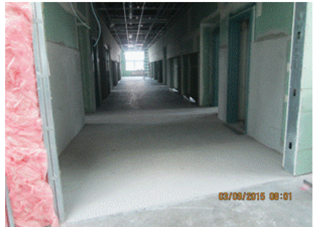
Building C - SGA: Moisture treatment at second floor corridor
