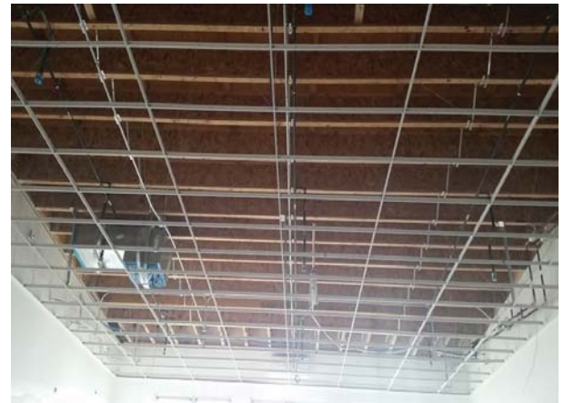
Building K - Classroom T-Bar Ceiling Grid Installation
