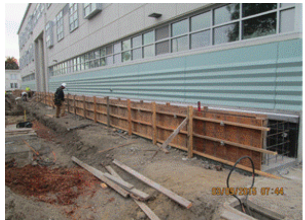
Site: Rebar and form work for planter boxes at north side
