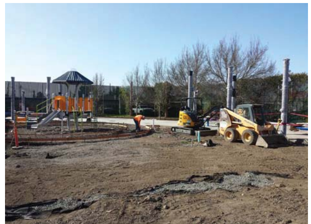
Forming & Grading of Court Yard
