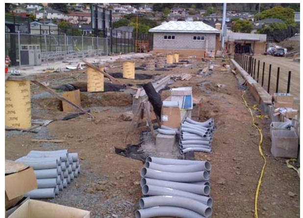
Visitor Bleacher Foundations
