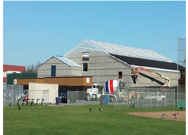
Building B - Roof Deck and Trusses
