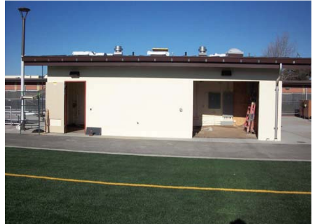
Restroom/Storage building painted
