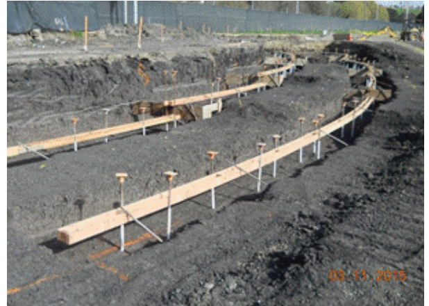
Ramp formwork
