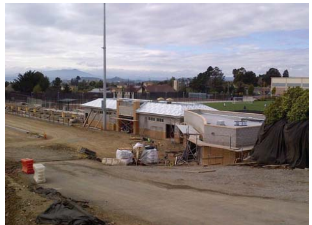
Building A & B - Roof
