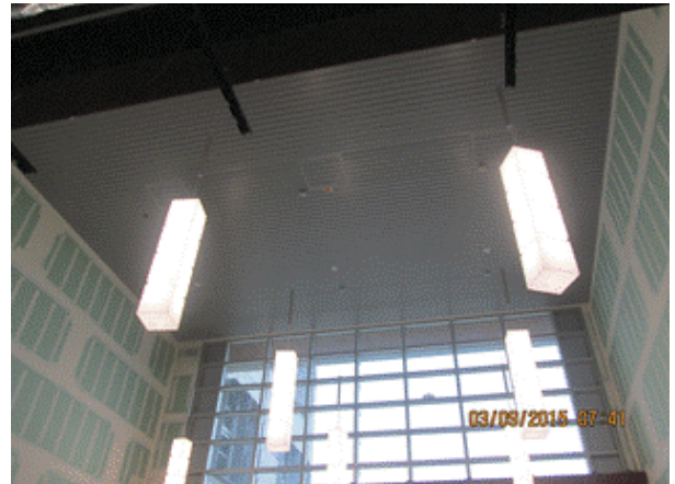
Building A - LPS: Metal ceiling and hanging light at lobby
