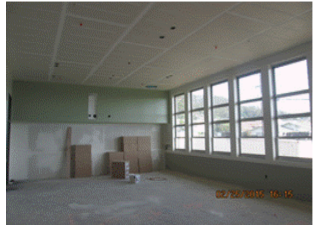
Building A - Prime and Paint interior walls on first floor
