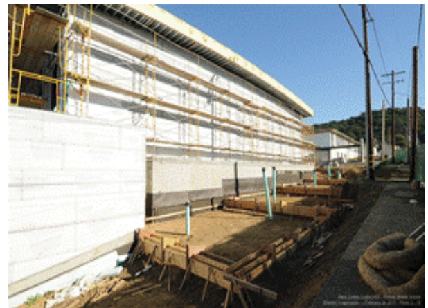
Site Level 2 - Planter Walls @ Stair 2
