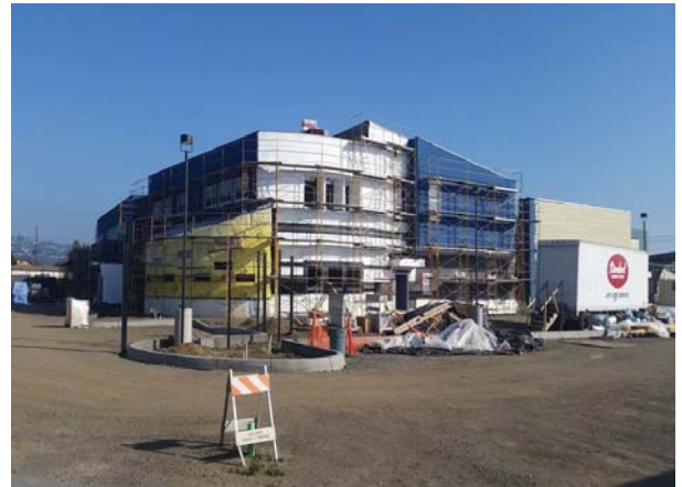
Building A - Wrap Northwest Section
