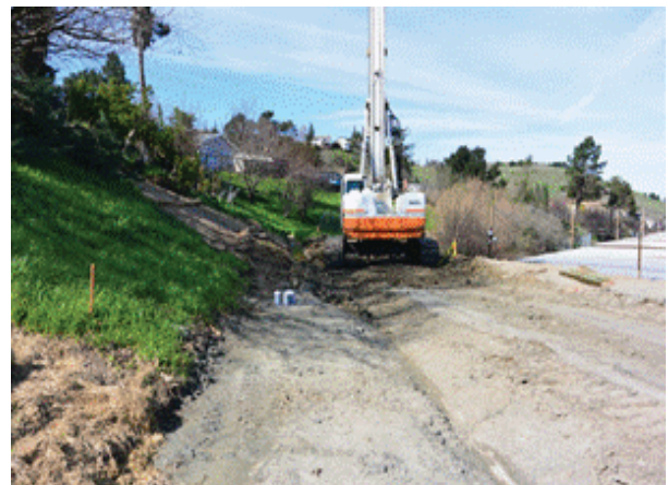
Drill and Set Piers
