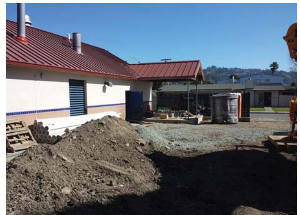
Storage Tank Canopy
