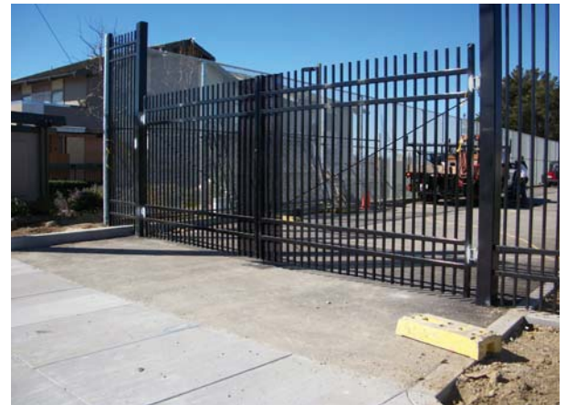
Fire Lane Entry Gate
