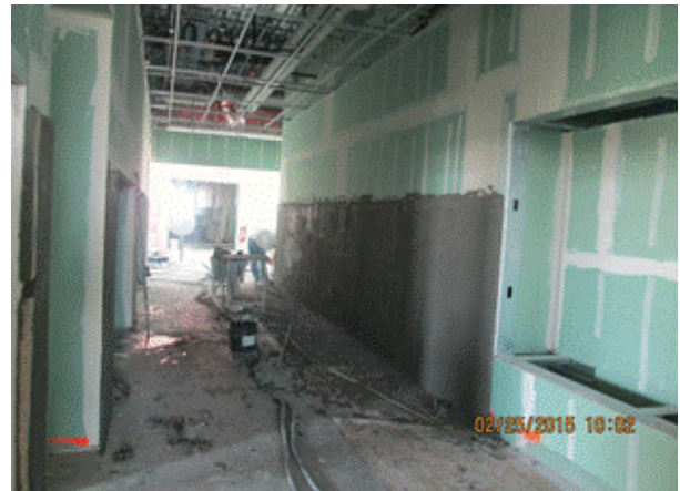
Building C - Mortar for tile at second floor corridor
