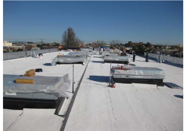
Roof Cap Sheet
