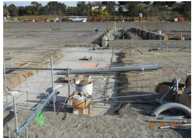
Concrete pour at building footings
