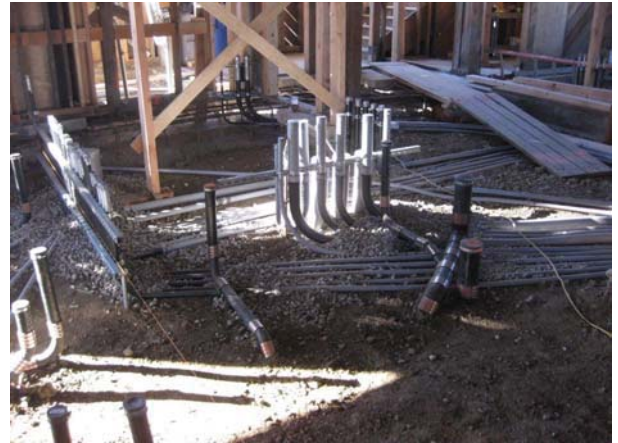
Plumbing and Electrical Under Slab
