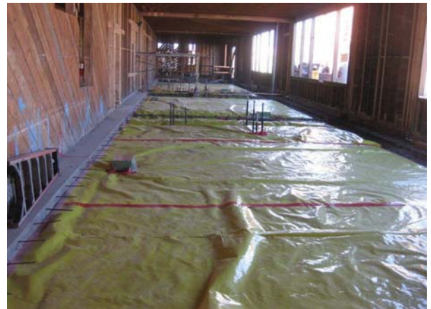
Under Slab Vapor Barrier
