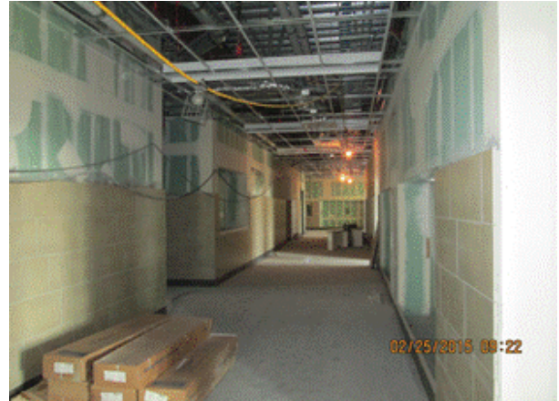
Building A - LPS: Tile corridor walls at second floor
