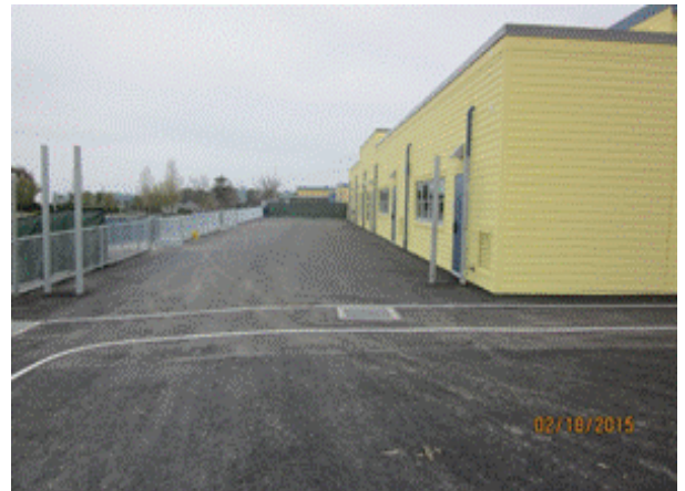
Exterior North elevation
