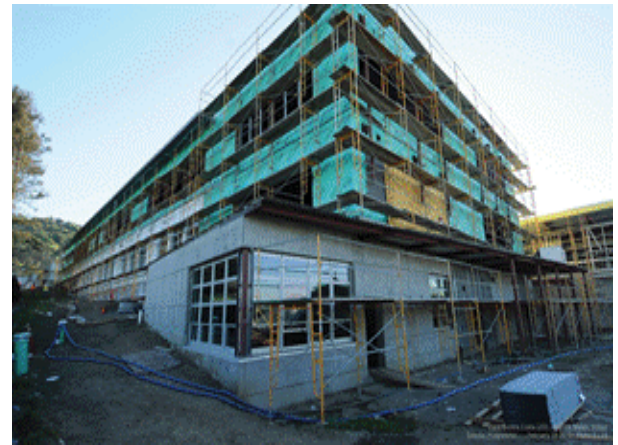
Building B - Storefront and curtain walls installation
