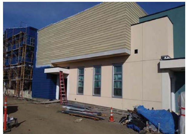
Building M - Fiber Siding Painting
