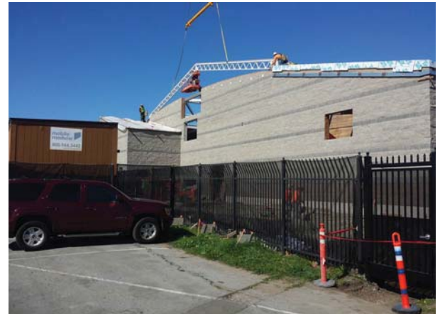
Erect Aluminum Trusses
