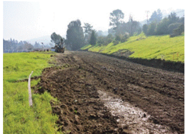
Grading for Crane Pad
