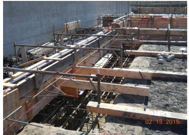
Formwork and rebar at building footings
