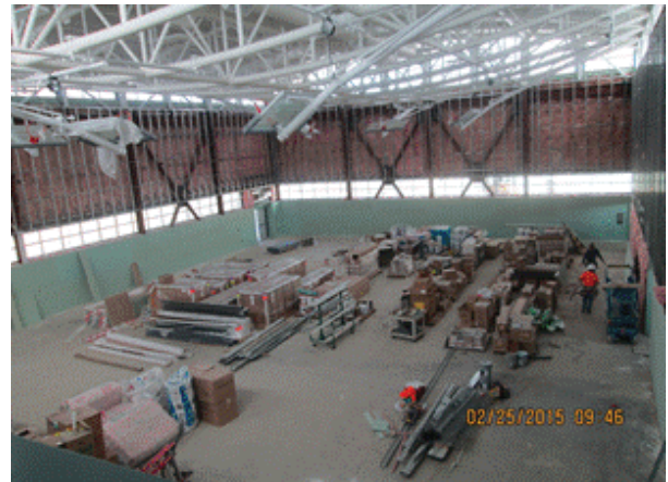
Building B - Gym: Insulation and gyp board at gym walls
