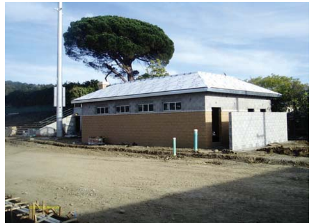
Building B - Mansard Roof complete
