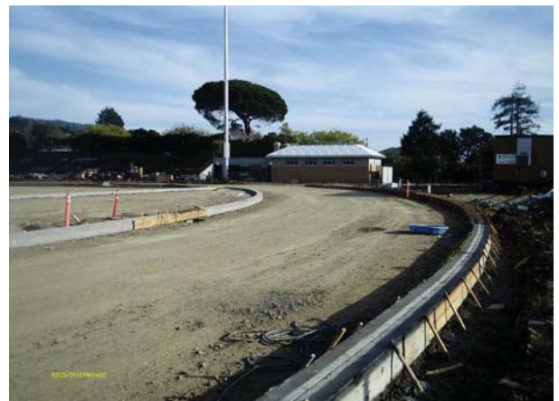
Stadium- Track Drains and Field Curbs
