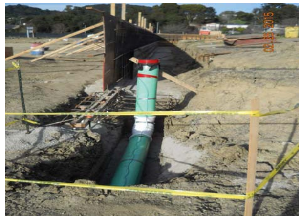
Storm Drain installation and retaining wall rebar
