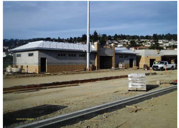
Building A - Windows installed
