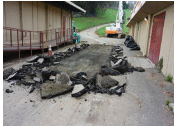
Preparing Truck Washout
