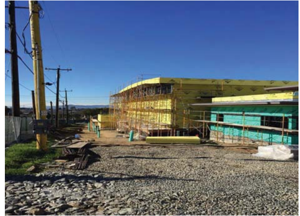
Building B - South View
