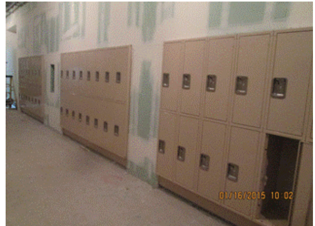
Building A - LPS: Lockers installed at corridor on 1st floor
