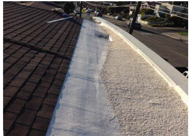
Building A-1 - Finish roof North side valley & drain
