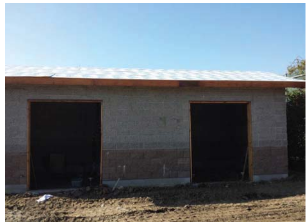
Pump House Waterproofing
