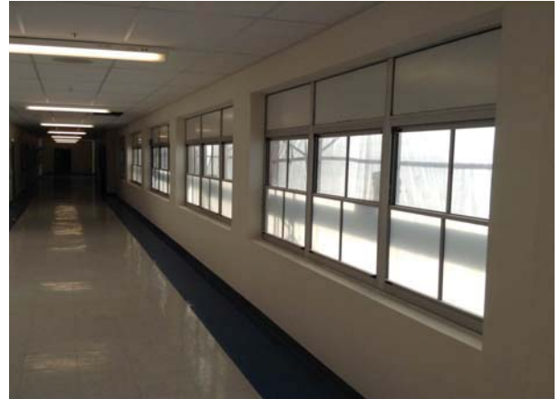
Building A - Second floor windows reinstalled
