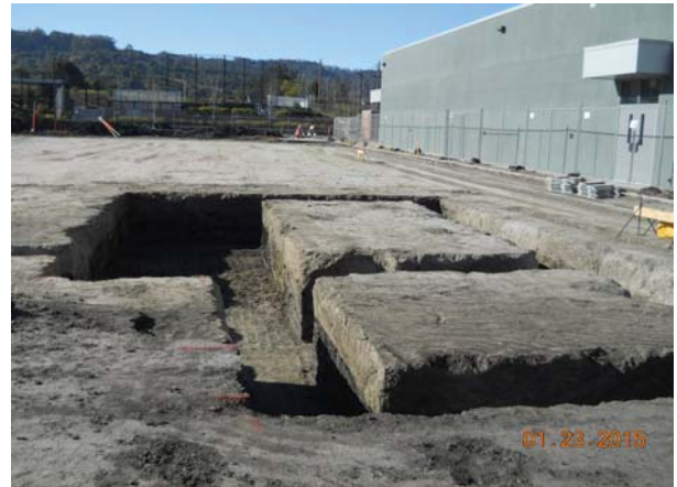
Footings at Building Pad
