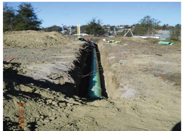
Storm Drain at Overflow Parking
