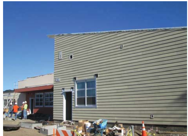
Building K - Siding
