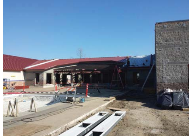
Building B - Roofing
