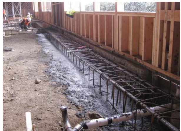
Concrete Pour for Footings at South Building
