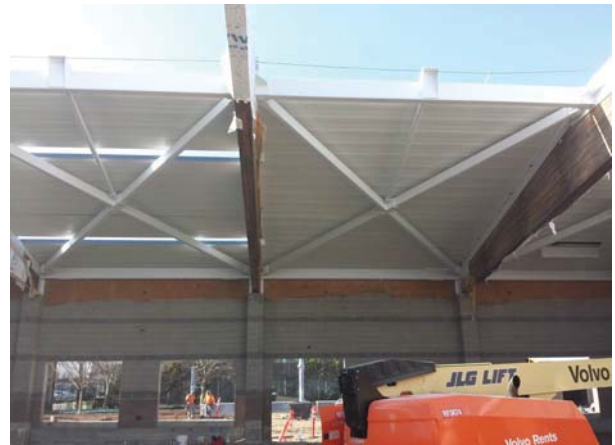
West Natatorium Decking
