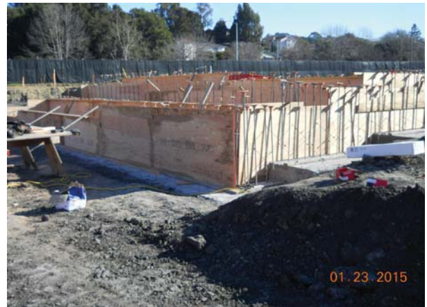
Formwork for Ramp Walls
