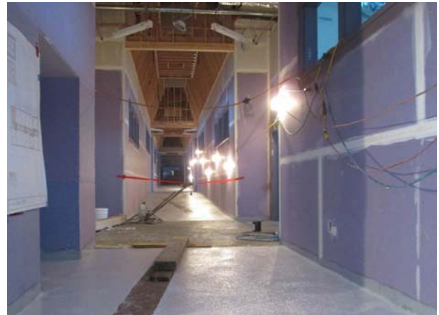
Building A - Terrazzo Floor
