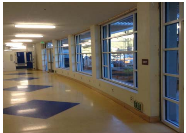
Building A-1 - Storefront interior hallway
