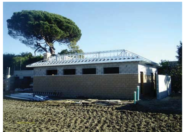
Building D - Roof Framing
