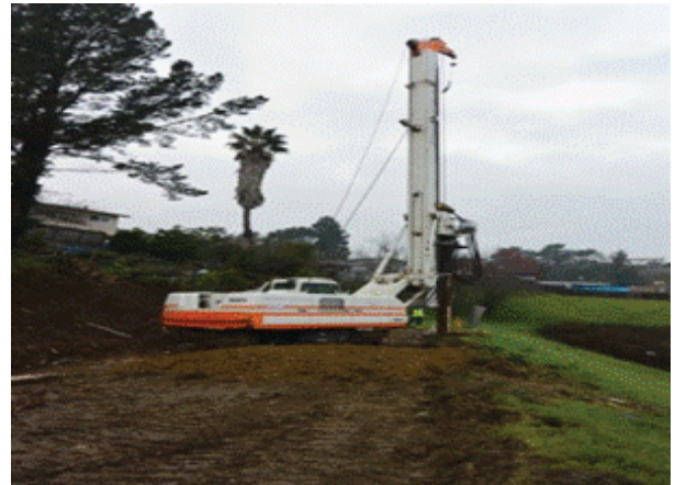
Drill and Set Piers
