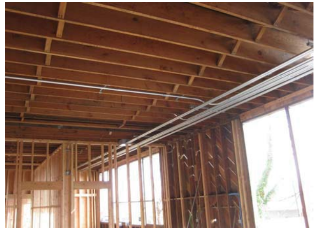
Installation of Electrical Rough-in at North Building
