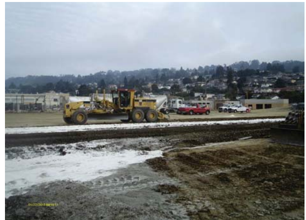
Stadium Field Lime Treatment
