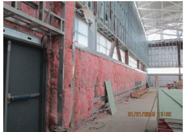
Building B - Gym: Insulation and Gyp board inside of walls
