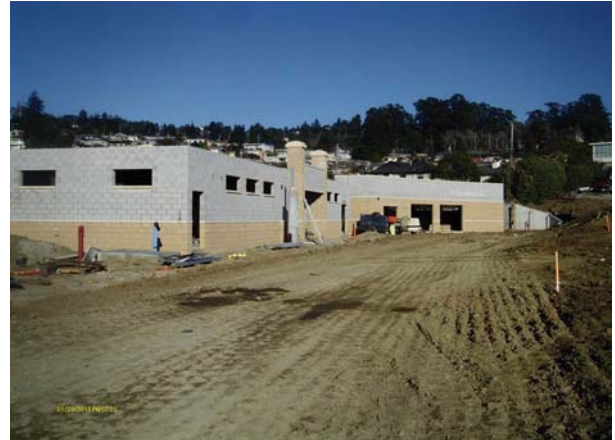
Building A & B - CMU & Roof Structure
