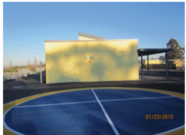
Exterior pavement and stripping
