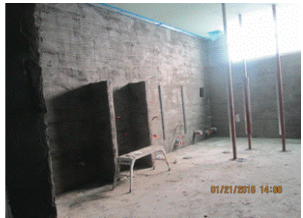
Building C - Gompers: Lath and Mortar on toilet room wall
