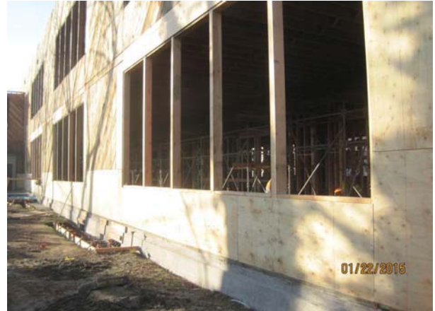
Installation of Replacement Diagonal Sheathing at South Building
