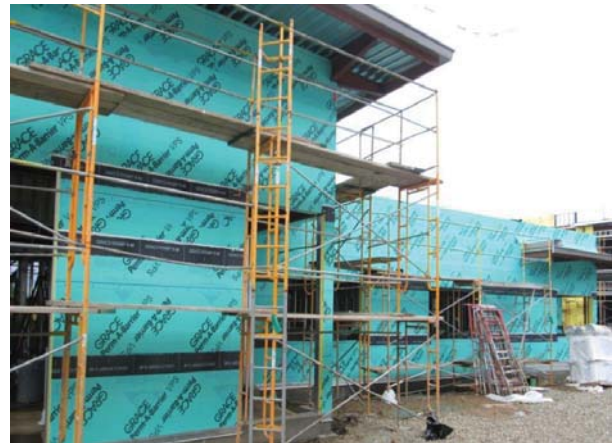
Building B - DensGlass® sheathing panel at exterior walls
