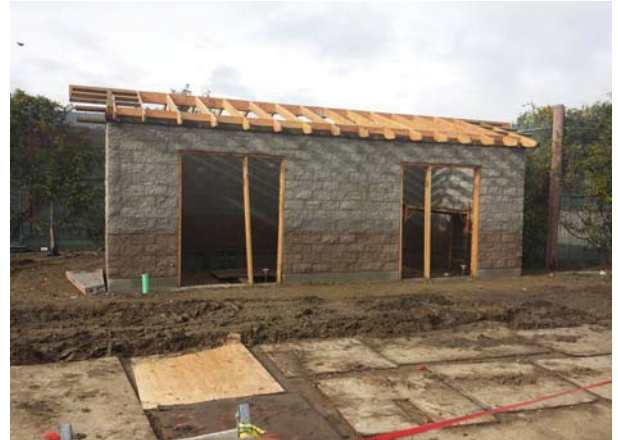
Roof Framing at CMU Pump House
