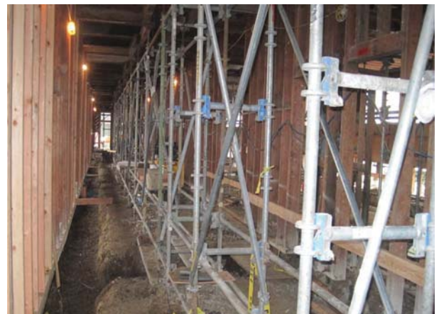
Installation of Shoring at South Building
