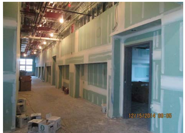
Building C - Gompers: Tape gypsum walls at corridors
