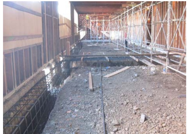
Rebar for Interior Footings at South Building
