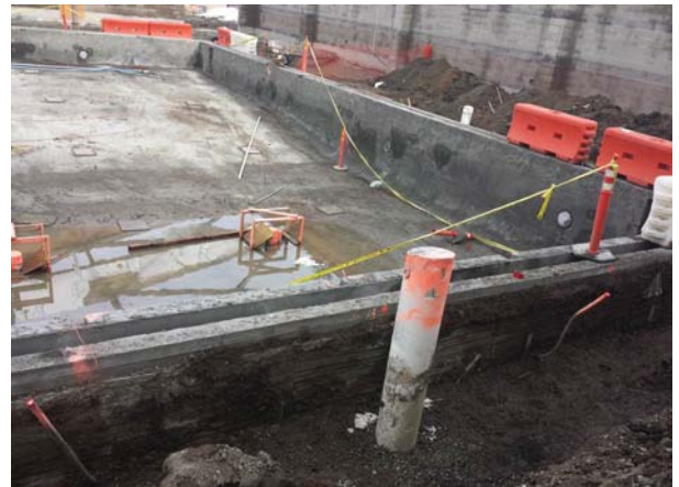
Main Pool Drain Trench
