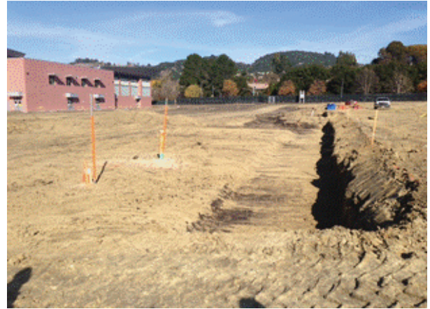
Excavation for retaining wall
