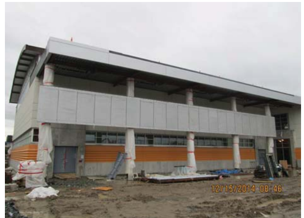
Building B - Gym: Metal wall panels installation at west side
