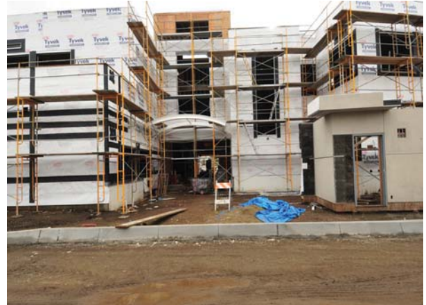
Building A - Entrance Exterior Wall Wrap Installation
