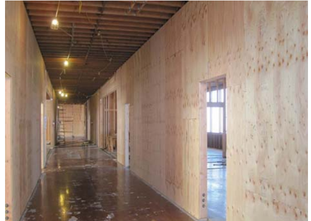
Installation of Shear Wall at South Building
