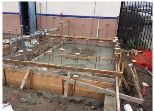
Chlorine Storage Tank Footings
