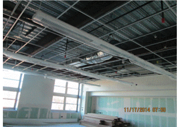
Building A - Heating equipment installed at classroom ceilings
