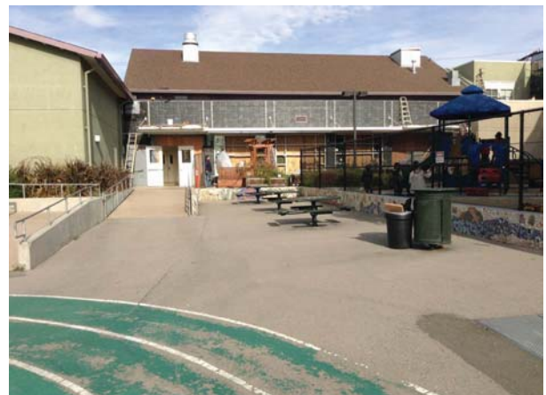
Storefront South Wall
