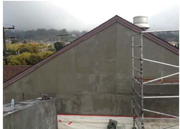
Theatre west wall stucco brown coat
