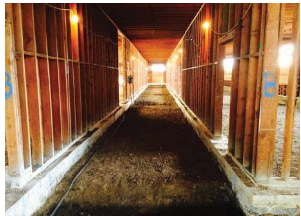
North Wing - Demolition of (E) Concrete Slab at Corridor
