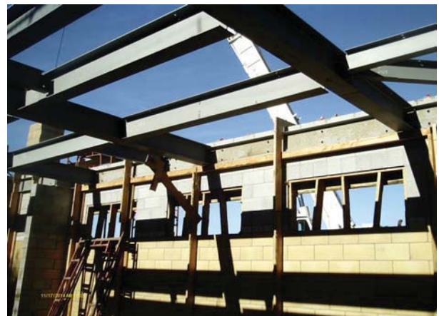
Building C - Steel Roof Framing
