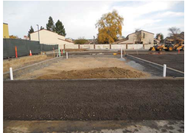
Playground concrete footing /pads/curbs
