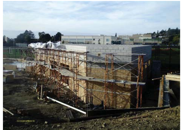
Building B - CMU complete
