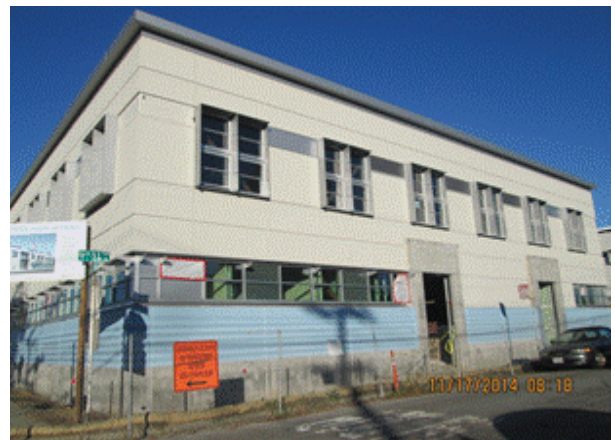
Building C - Finished painting / Installing metal wall panels
