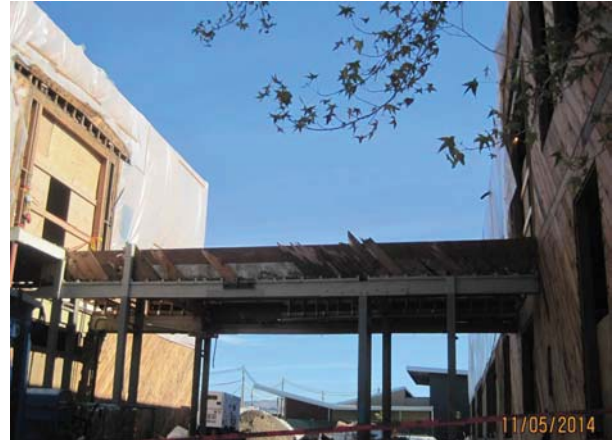
(E) Center Breezeway - Demolition
