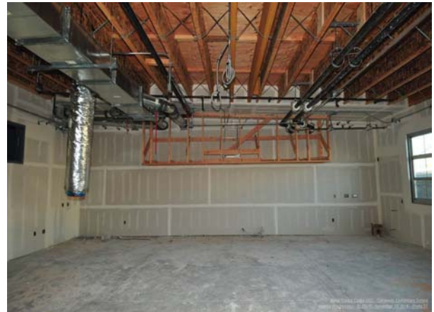
Building C - Classroom Interior Drywall Installation
