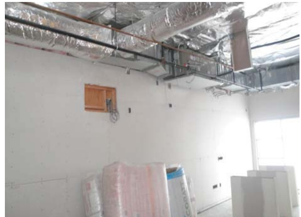
Building A - Sheetrock & Tape
