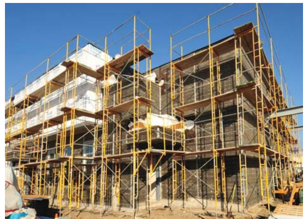
Building M - Exterior Plaster lath
