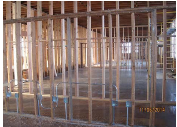
Installation of Interior Partition Walls with Junction Boxes
