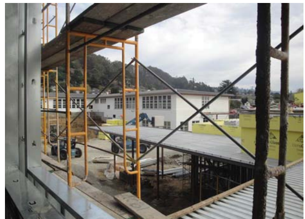
Building B - Roofing
