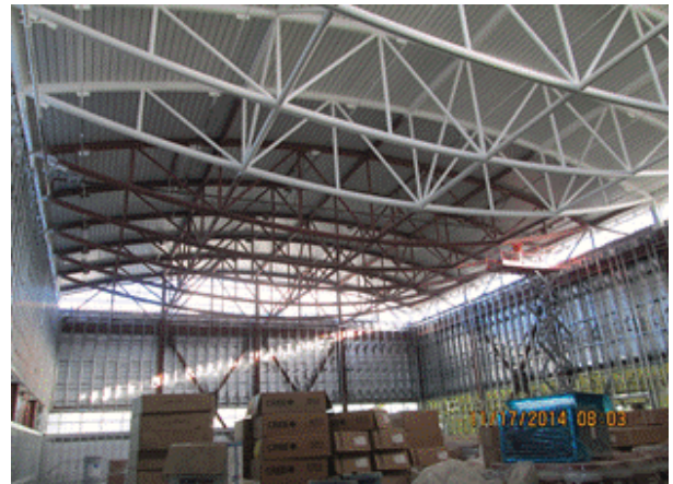
Building B - Painting exposed structural steel
