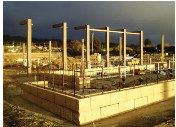
Building E - Two Courses of CMU & Under slab prep
