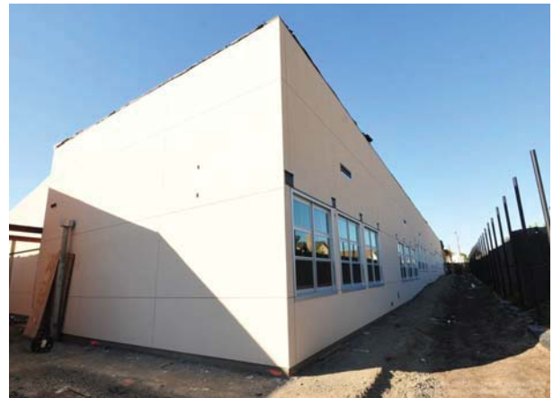
Building K - Exterior Plaster
