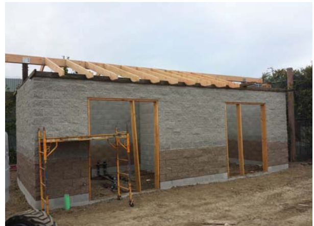
Pump House CMU & Roof Framing
