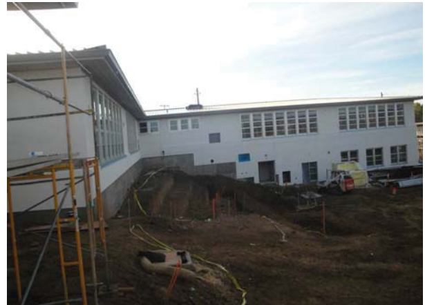
Building A - Stucco & Windows
