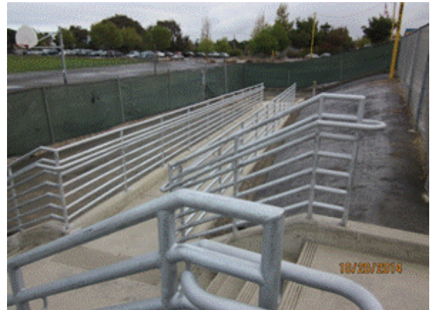
Steel handrails ramp walk way.
