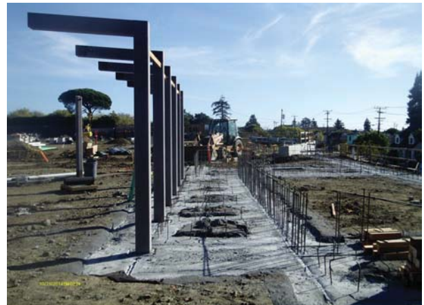
Building E - Footing poured with steel canopy frames
