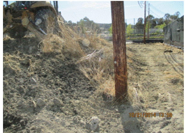
Clearing and Grubbing
