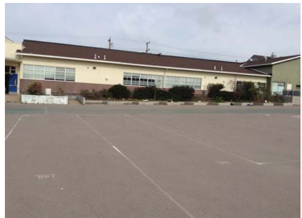
Building A-1 Exterior-Roof & Gutter
