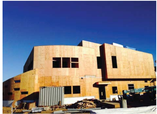
Building A - Exterior Framing
