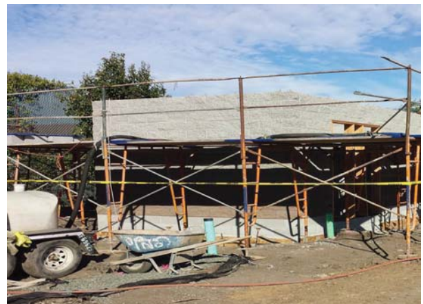
Grouting CMU Pump House
