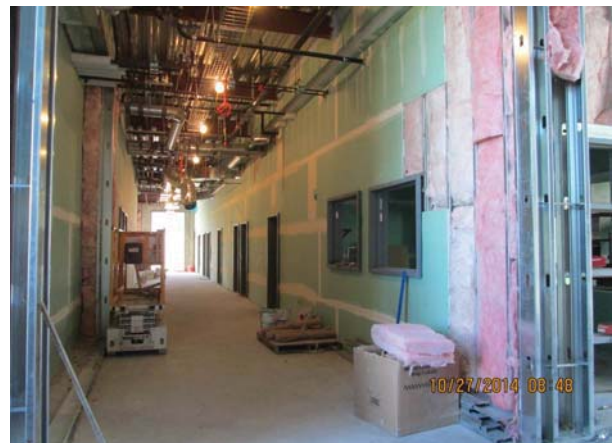
Building C - Interior gyp board & insulation
