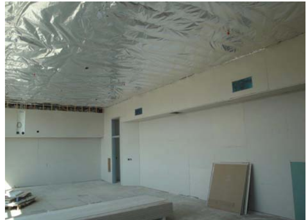
Building A - Sheetrock installation/Classrooms 1st floor
