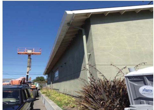
Building A - West end gutter replacement
