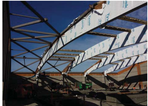
Structural Steel Cross Bracing
