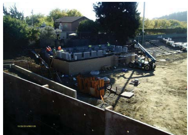
Building C - Team Room CMU wall installation
