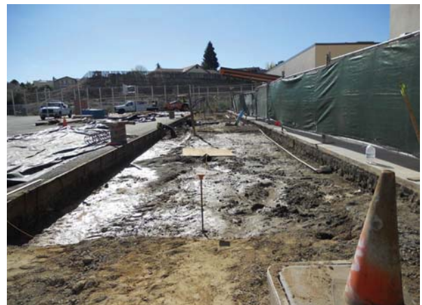
Excavating for planter boxes
