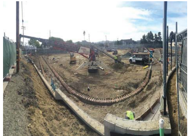
Trench drain at North Side of Track
