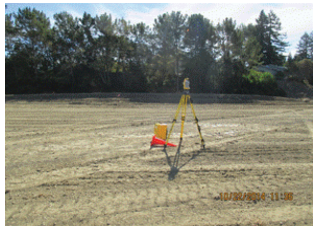
Survey Rough Grade
