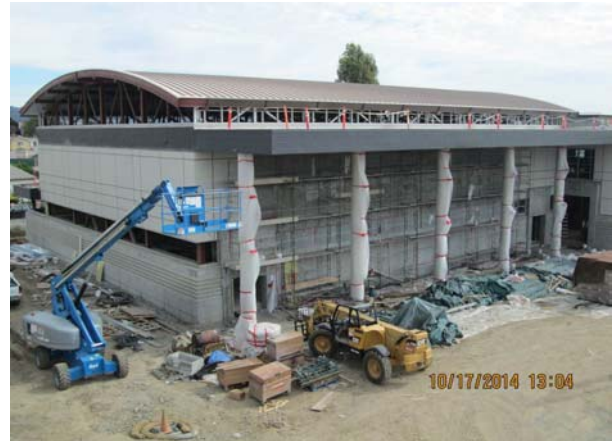
Building B - Exterior plaster at West and North sides
