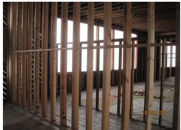
North Wing - Installation of Interior Partition Walls
