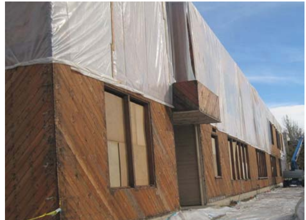
North Wing- (E) Redwood Siding & Trim Removed
