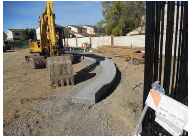
Site Concrete Curbs
