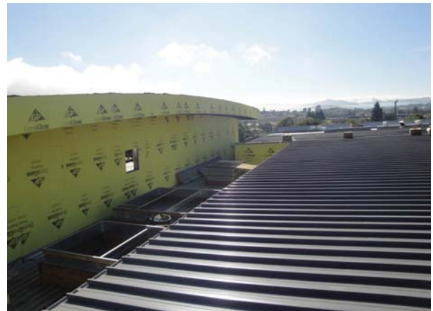
Building B - Library metal roof and GYM upper wall
