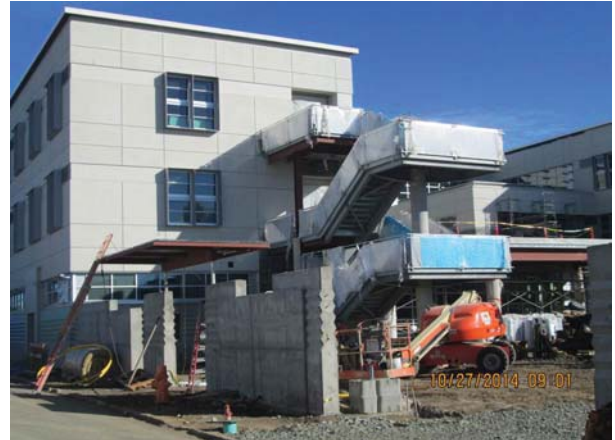
Building A - Handrails at stairs & entrance canopy on 8th st
