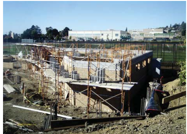
Building B - CMU wall set up to plate height
