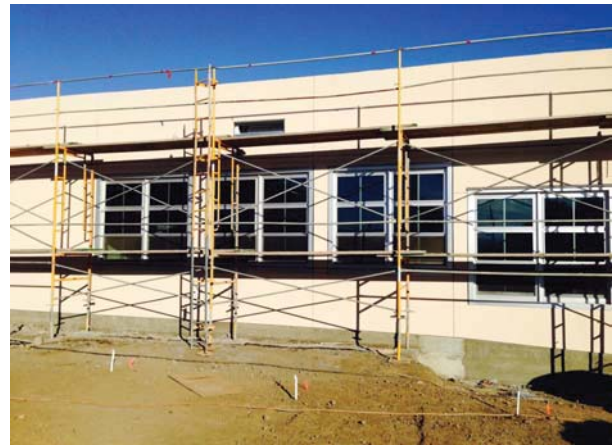
Building C - Classroom Plaster
