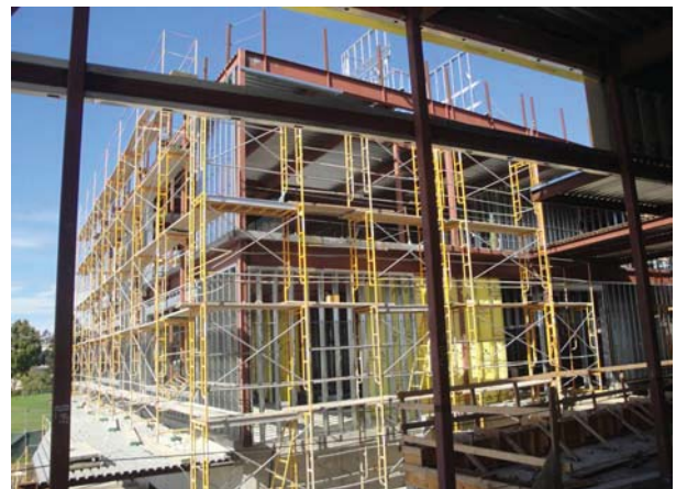
Building C - Exterior Framing
