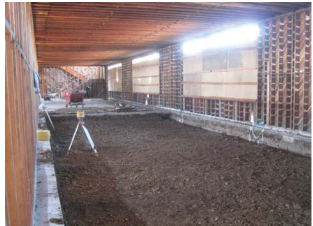
North Wing - Removed (E) Interior Concrete Slabs
