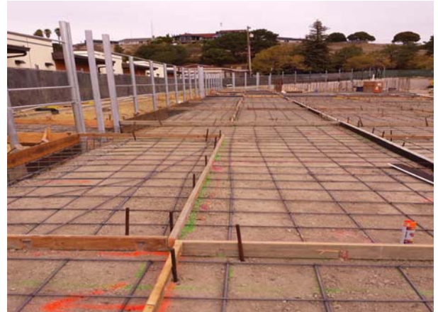
Form Work & rebar for Concrete Flatwork around Restroom Building
