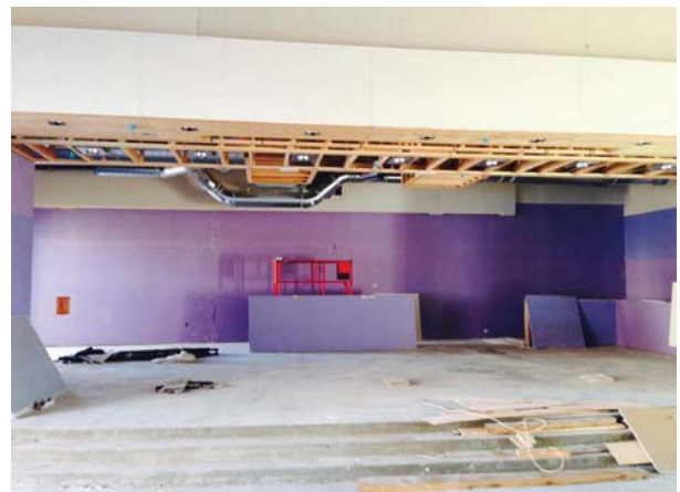
Multi-Purpose Room Stage - Gypsum Board Installation
