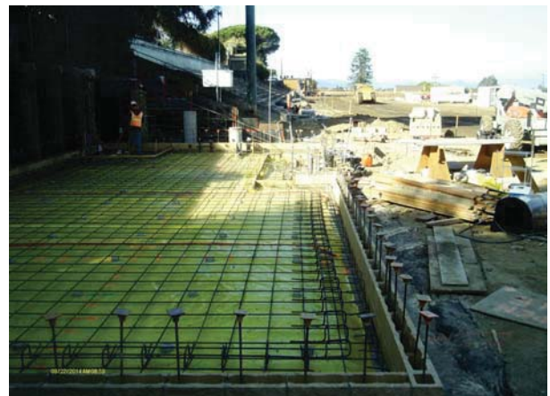
Building C - Team Room ready for concrete slab
