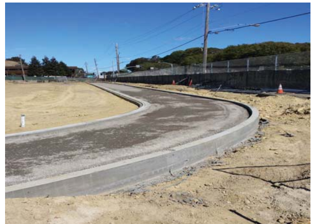
Soccer Field - Installation of AB at track
