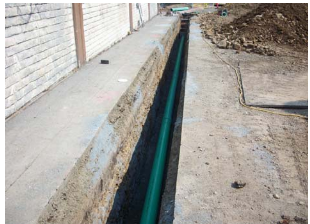
Trenching / Storm Drain Installation
