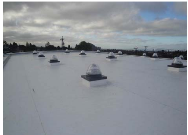
Building B - Sky Lights GYM Building
