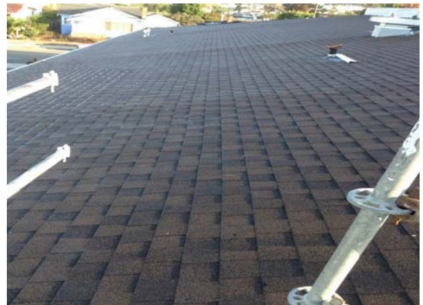
Complete Shingle Installation
