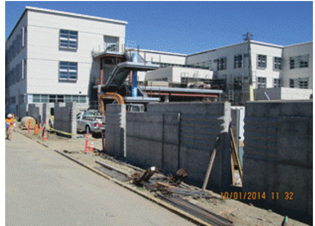
Building A - Scaffold removed & site walls on 8th street
