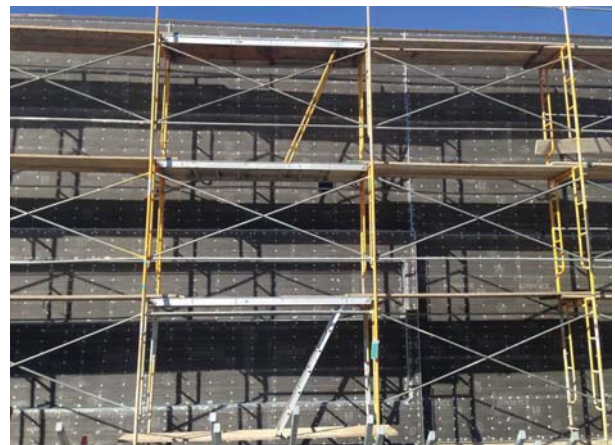
Building M - South Exterior Wall Lath Installation
