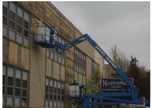
North Wing - Removal of Transite Panels
