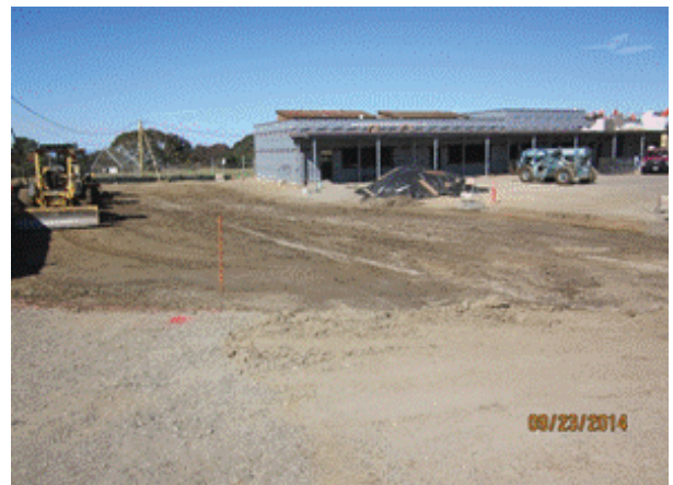
North West elevations weather barriers & finish grading
