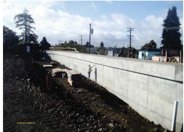
Final section of Ashbury Retaining Wall
