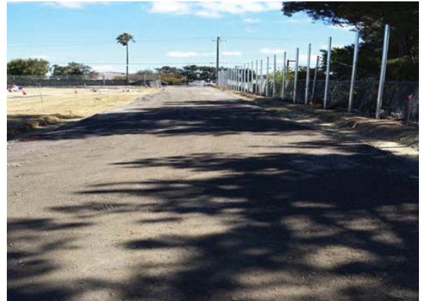
Installation of AB at fire lane & fence poles on South side
