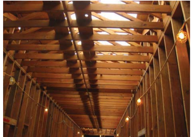
North Wing - Removed Roof Deck Membrane
