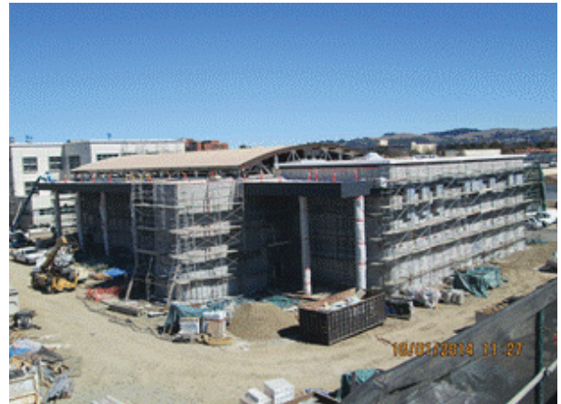
Building B - Gym: Exterior plaster
