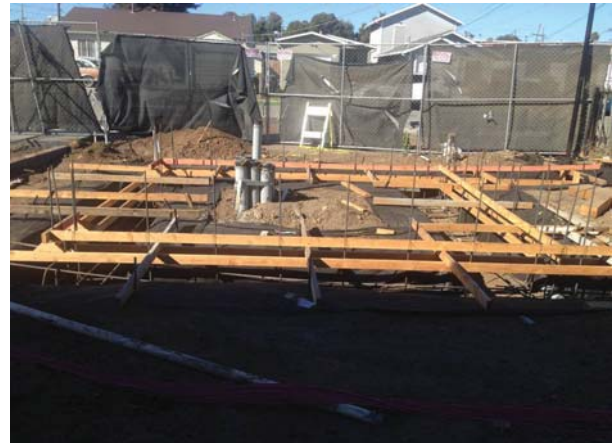
Footing Form Work for CMU PGE Enclosure
