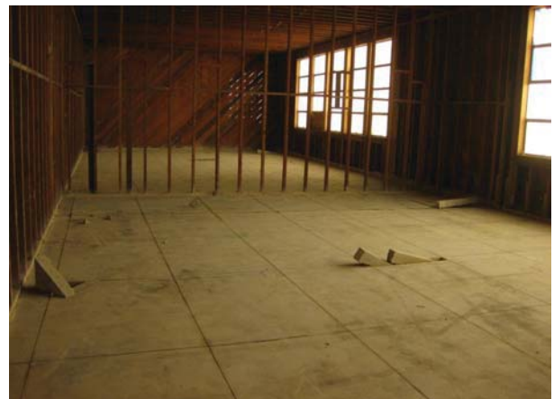
South Wing - Saw-Cut Existing Concrete Slabs
