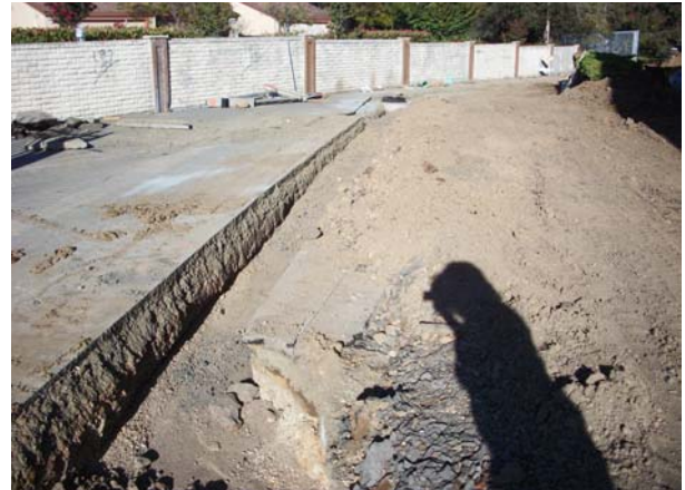
Backfill of Trench
