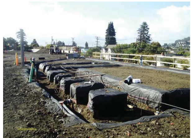
Building E - Footing excavation
