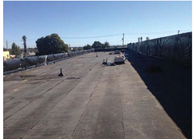
Building C - (East) Built Up Roof Placement
