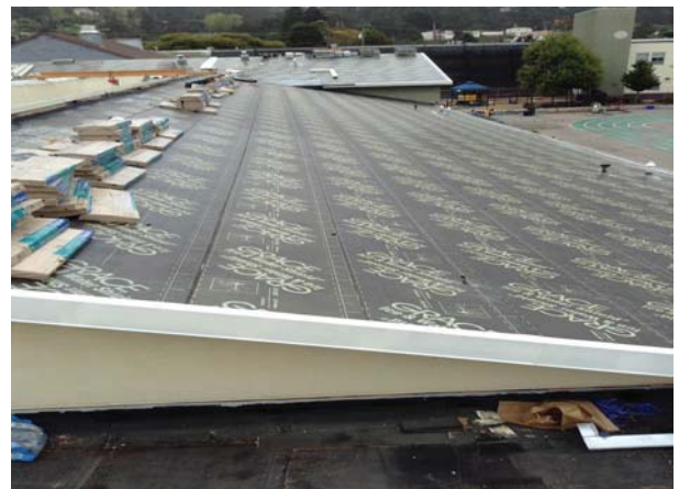
Roofing Membrane - looking east
