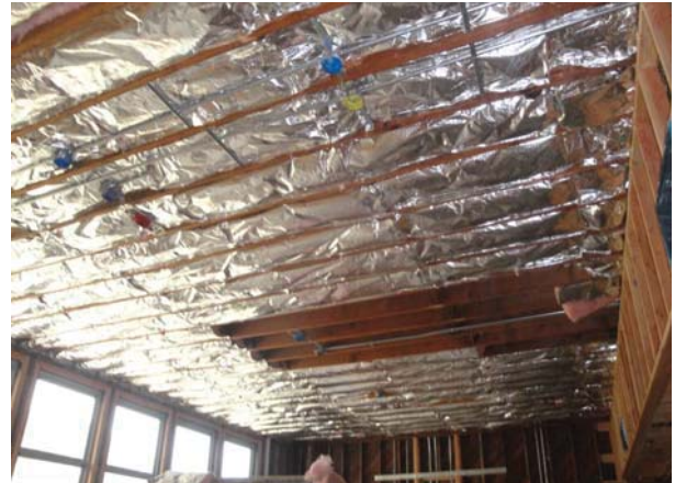
Building A - Insulation
