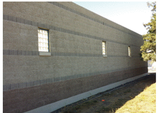
East Wall Sandblasting
