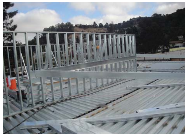
Building C - Roof Mechanical Parapet Wall Screen
