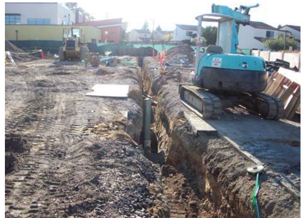
Storm Drain Work
