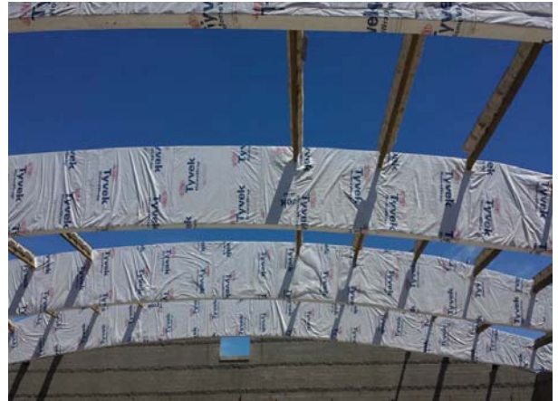
Demolished Roof and Wrapped Glulams
