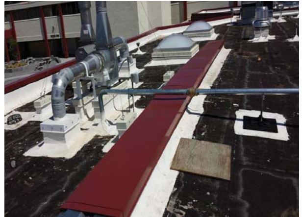
Parapet Flashing
