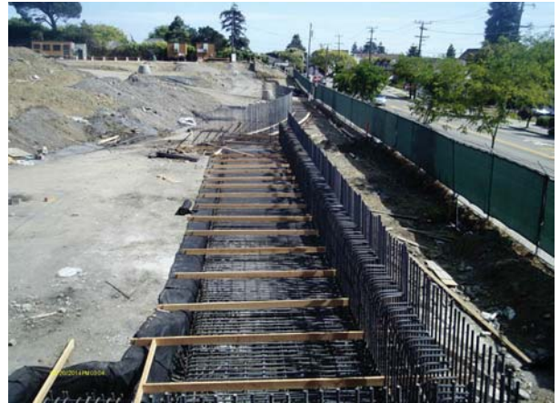
Ashbury retaining wall rebar installation ready for concrete.
