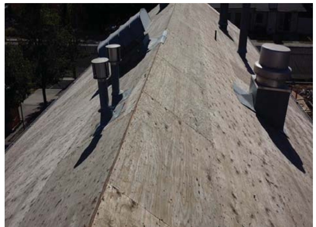
Pre-Inspection Roof Sheathing
