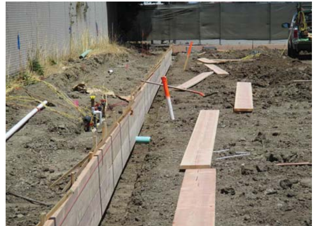
Forms for placement of concrete for curb
