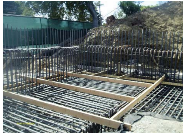
Ashbury retaining wall footing adjacent to tennis courts
