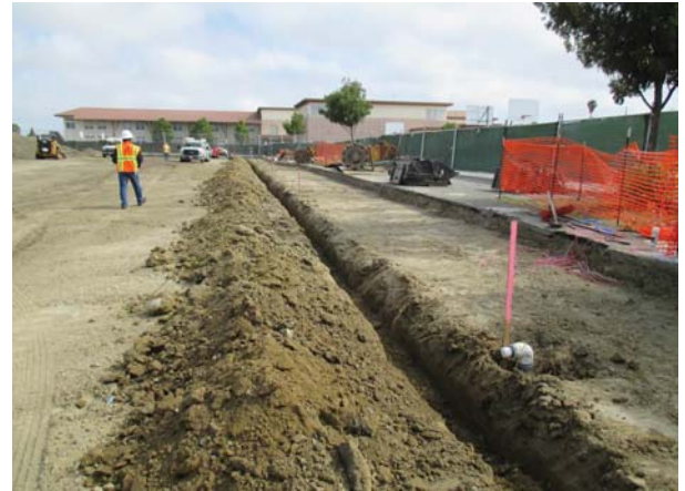
Irrigation trench excavated
