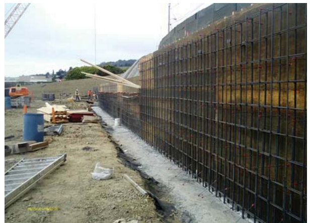
Lower Colusa Ave. retaining wall rebar installation
