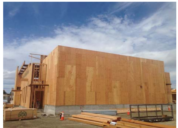
Building M Framing Exterior Ply
