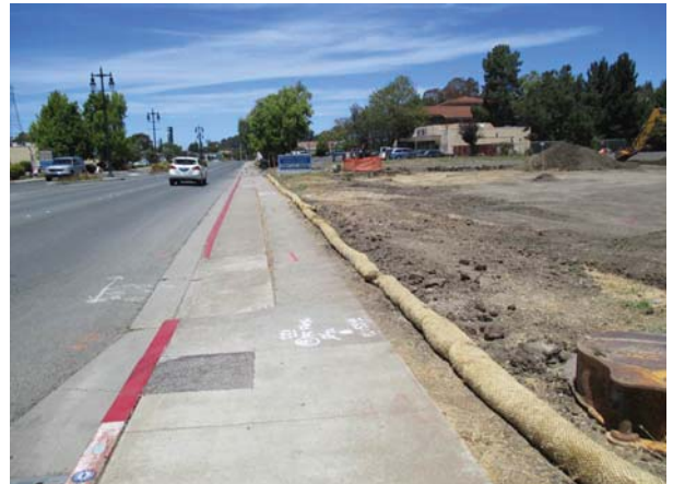
Grading at Church and SWPPP BMPs
