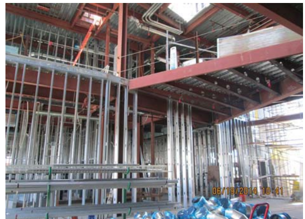
Building C - Interior Framing
