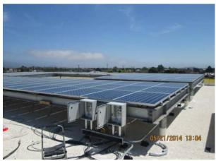
**Building C - Combiner Box for Solar Panels Installation**
