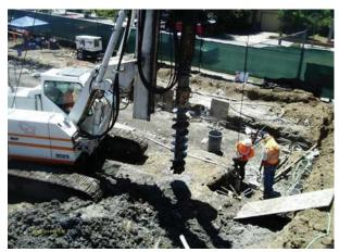
Drilling rig set-up for a 33'-0" deep concrete pier
