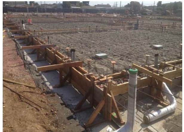
Building C Edge Forms & Rebar For SOG
