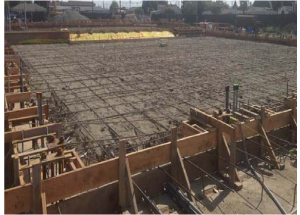
Multipurpose Room. Edge Forms for Slab on Grade
