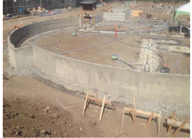
Bldg. A-Wall Northwest Section concrete poured & forms stripped
