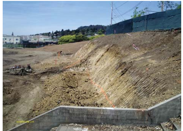
Colusa hillside cut in anticipation of retaining wall forming
