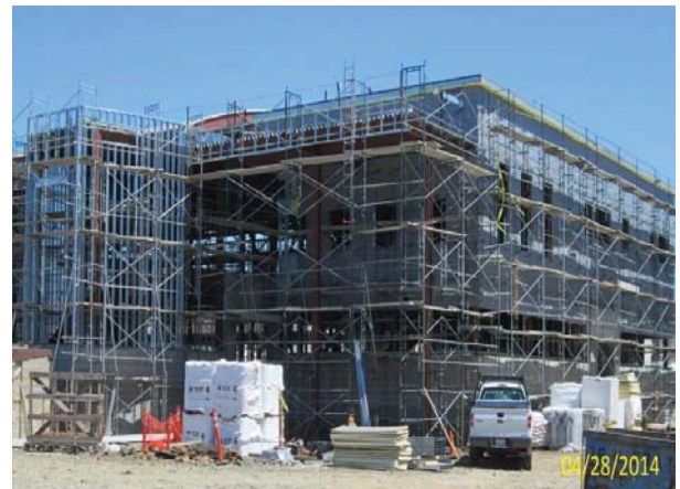
Building B - Metal Framing & Weather Barrier At South & West Sides
