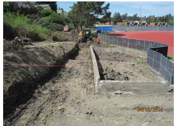
Excavation and Grading at Walkway
