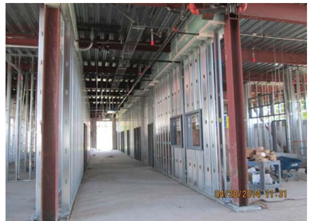
Building C - Interior Metal Framing at the Corridor in 1st Floor
