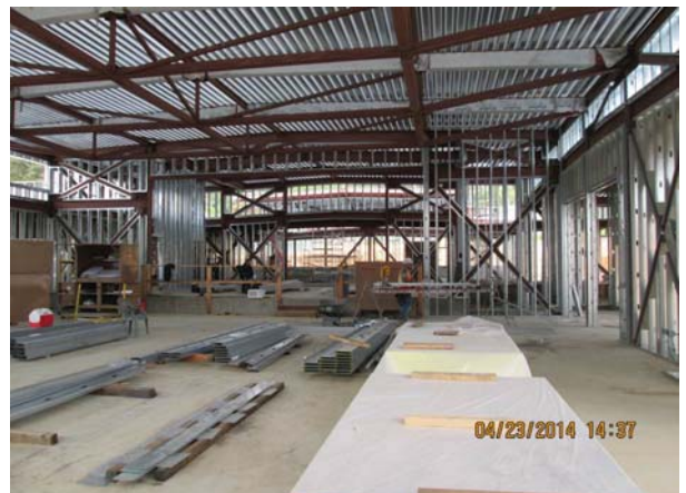
Building D MPR wall framing
