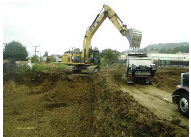
Over Excavation and Off Haul
