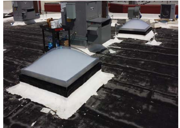
Flashing Tape at Skylights
