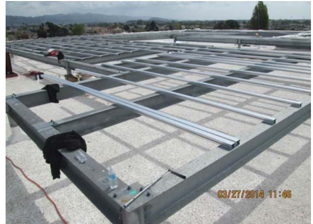
Building A - Solar Panel Support Railings
