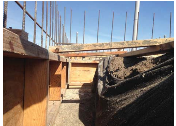
Building M Multi Purpose Room Wall Forming for Stage (1)
