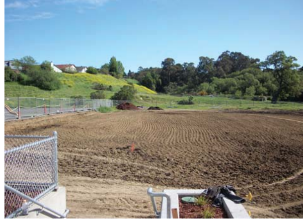
Prep subgrade for interim housing pad
