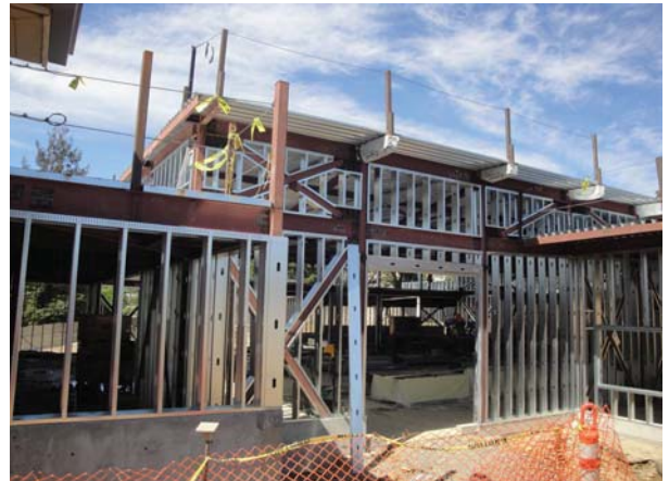
Building D Stud Framing
