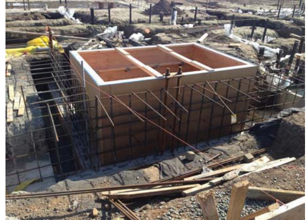
Building A Elevator Wall Forming
