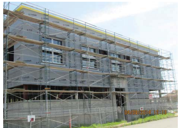
Building C - Window & Shadow Box Installation at West Side
