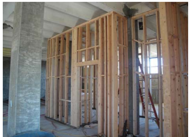
Building A Basement wall framing
