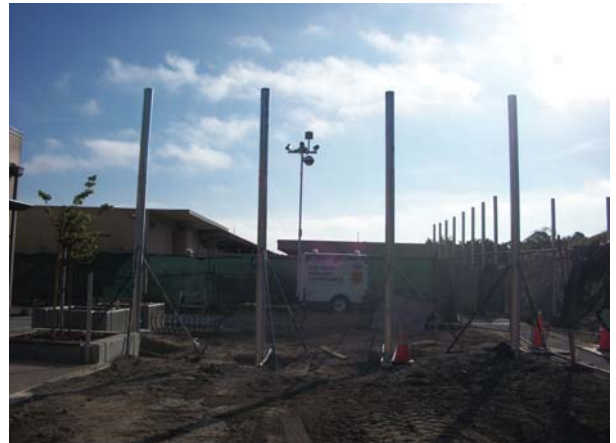
Pier installation for 20' Fence Posts
