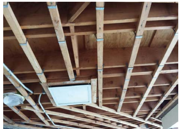
Covered Walkway Ceiling Removal
