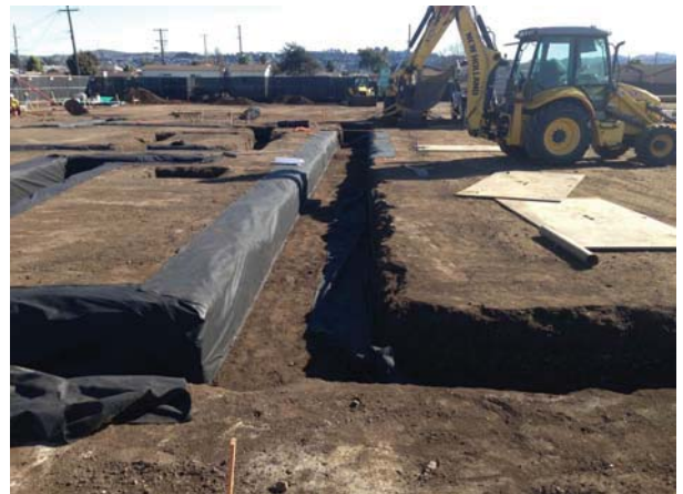
Building A Footing Excavation
