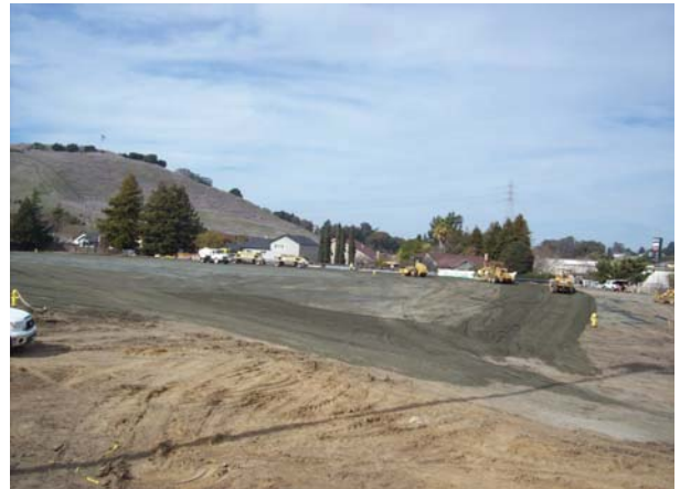
Installation of Class 2 Aggregate Base and Compaction
