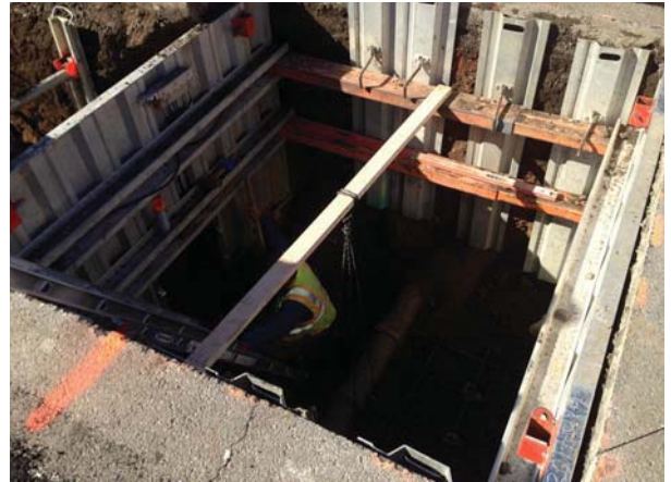
Underground Sanitary Sewer Tie-in
