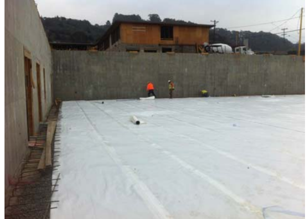
Building B GYM Vapor Barrier prior to slab pour.
