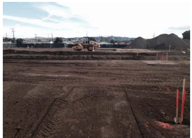
Bldg. M & Parking Lot-Rough Grading & Preparing Building Pad
