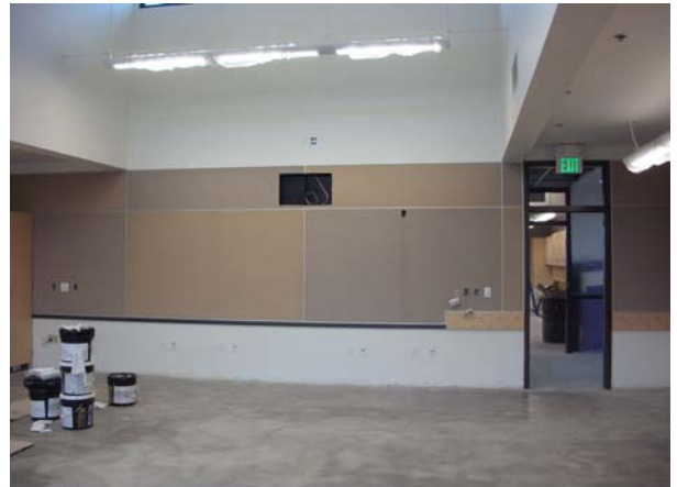
Building B - Classroom Tackboard Install
