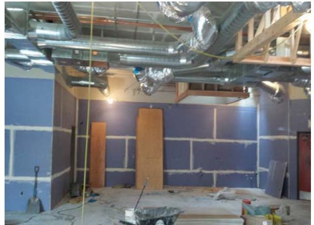
Room 407 - Drywall and Taping
