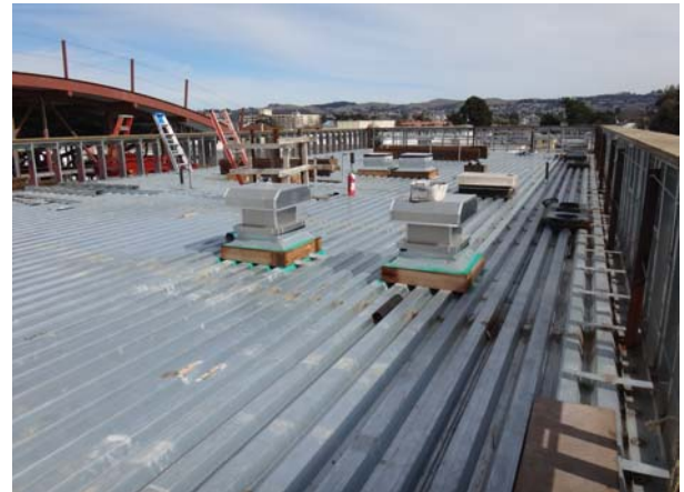
Building B - Wood Curbs at HVAC Units at the Roof
