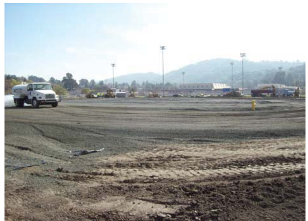
Installation of Class 2 Aggregate Base and Compaction
