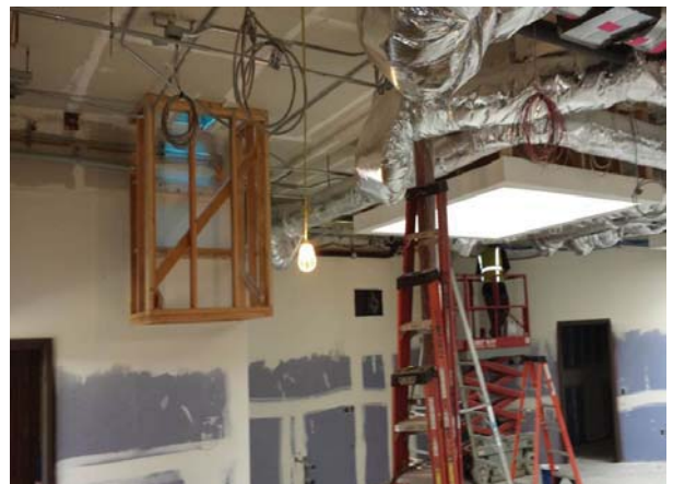
Room 408 - Skylight and Fume Hood Soffits
