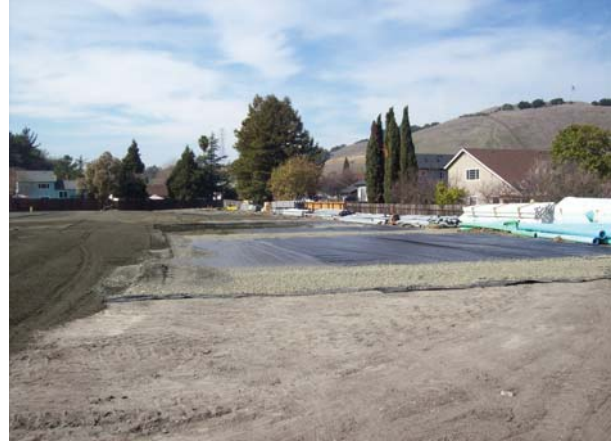
Installation of Fabric and Class 2 Aggregate Base
