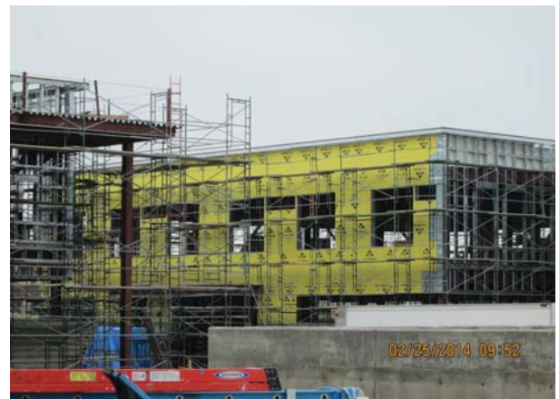
Building C - Z Metal and THERMAX Installation at North Side
