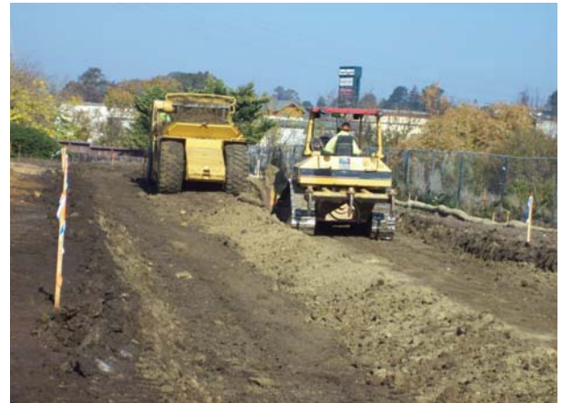
Excavation for Detention Basin
