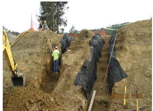
Building C - Step Footing Excavation
