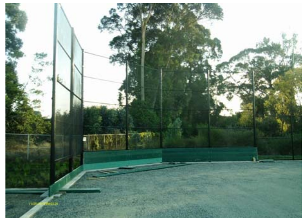
Baseball backstop and class II perm base rock for synthetic turf
