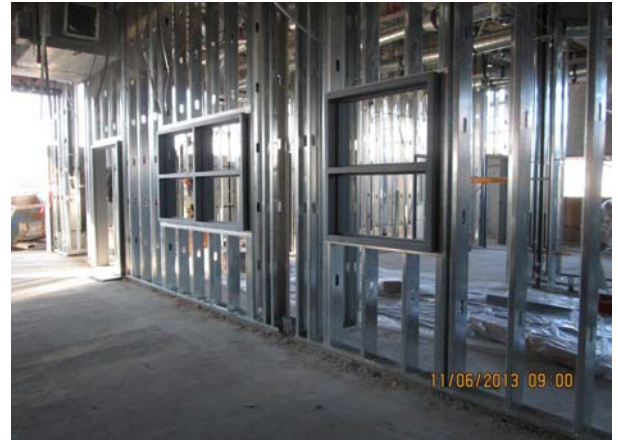
Building A - Interior Metal Stud Framing
