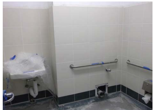
Downer Restroom Tile Installation - IN PROGRESS
