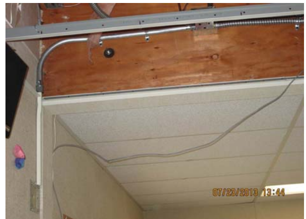
New wiremold, conduit and device location in Portable Bldg.
