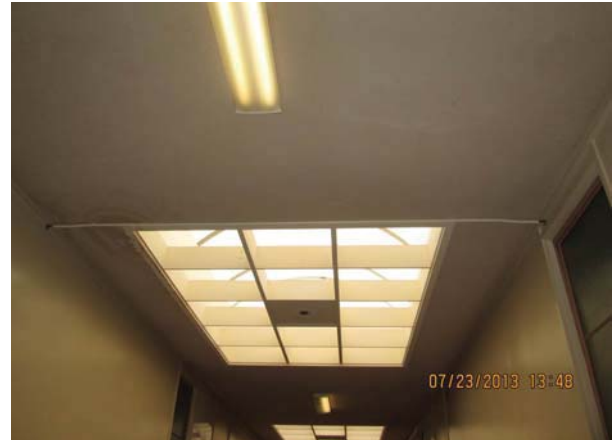
Wiremold at skylight in Classroom wing
