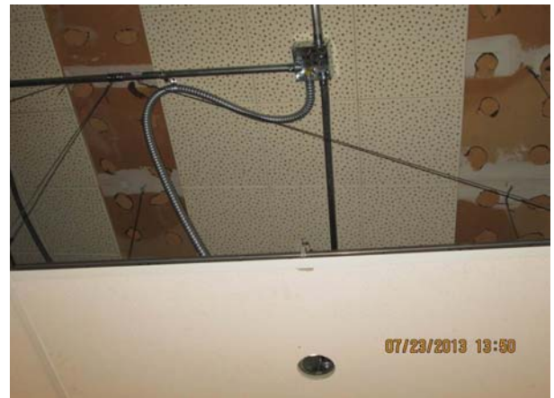
New conduit and junction box above ceiling in classroom
