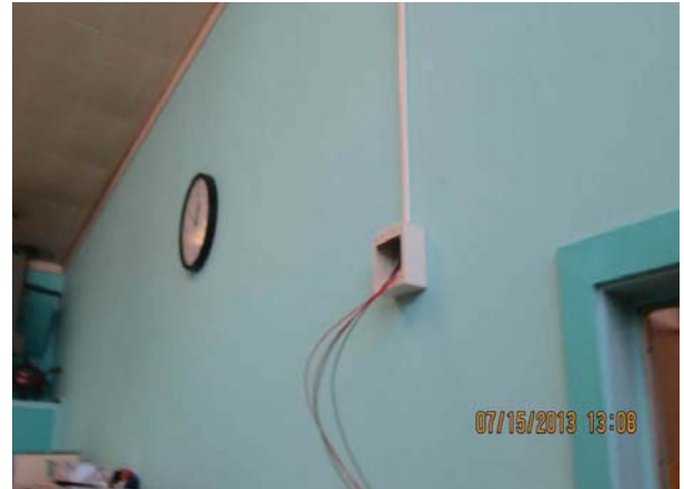
Wiremold, pullstation location and wiring in Teachers Lounge
