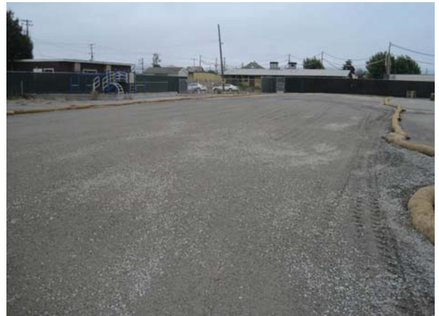
Kinder Area Compacted w/ Recycled Concrete
