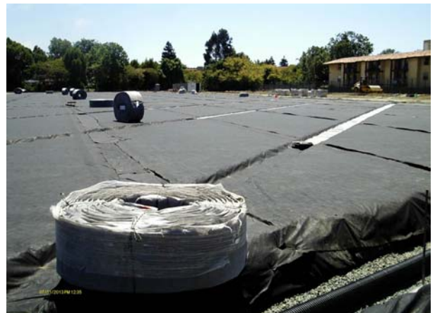
Installation of drainage fabric with flat panel drains on main field
