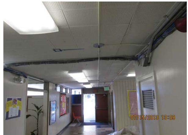
Wiremold and device location in Administration Building
