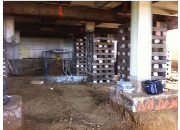
Lowering of Building A Basement Slab & Footings 30%.
