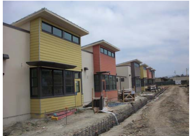
Sunshades/Retaining Wall Rebar on South Side
