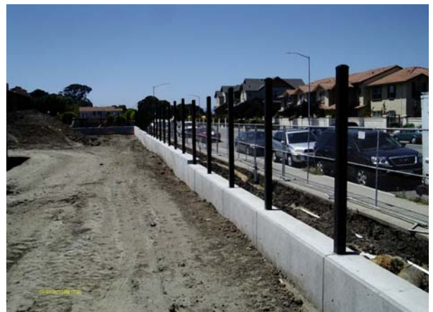
Road 20 retaining wall is back filled with ornamental fence
