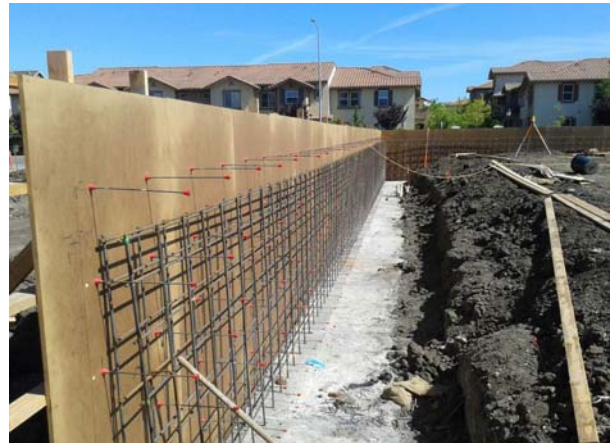
Concrete retaining wall forms and rebar around track at Road 20
