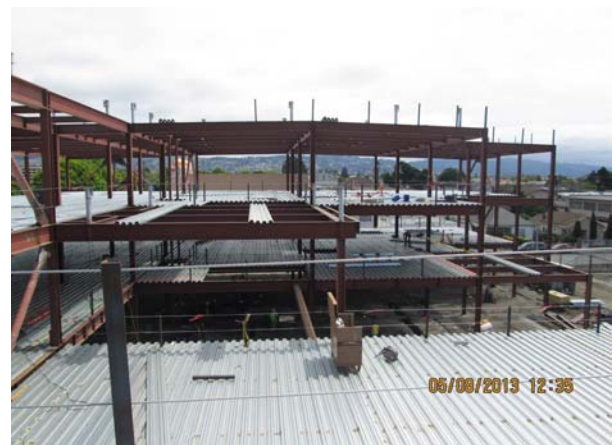
Building A - Steel & Pan Decking
