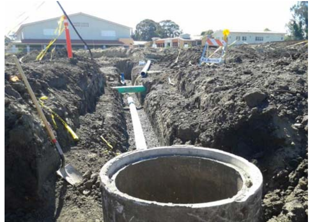
Community sanitary sewer trenching and rough in.
