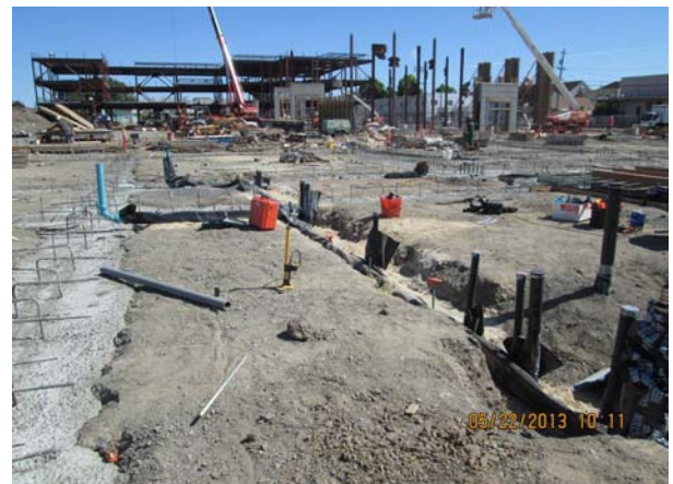
Building C - Underslab Plumbing
