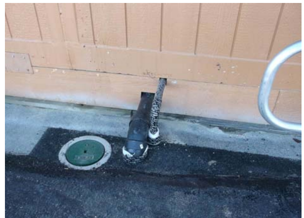
CCS @ Downer - Install Water Shut off Valve - IN PROGRESS
