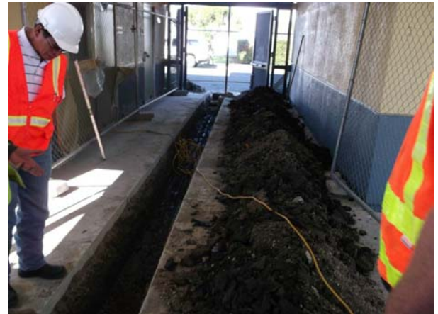
Installation of Underground Storm Drains - IN PROGRESS
