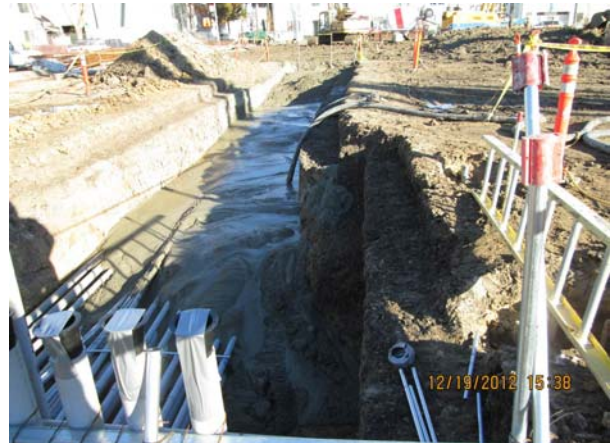
Electrical Trench Backfill
