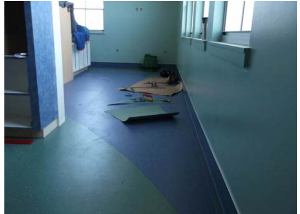
Installation of (N) Linoleum Flooring - COMPLETED
