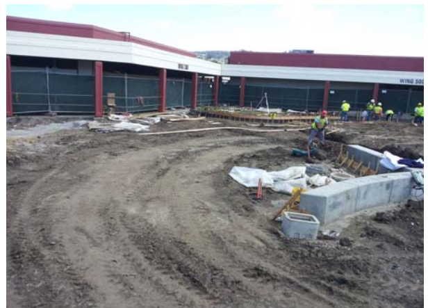
Forming Mow Strip and Flatwork
