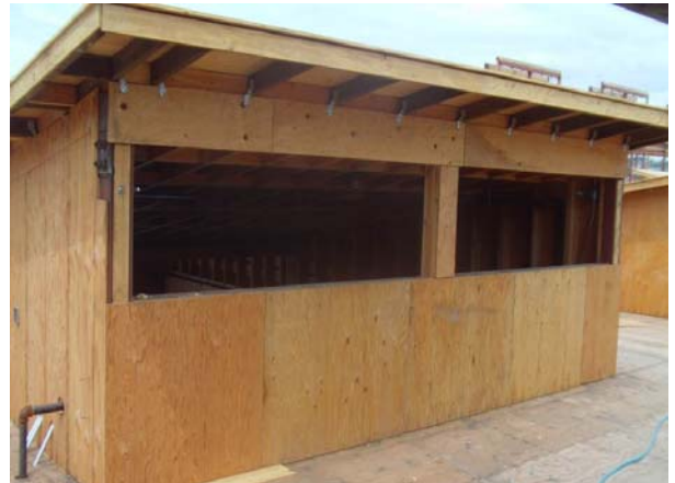
Building B Classroom 102 Clerestory Framing at Butterfly Roof
