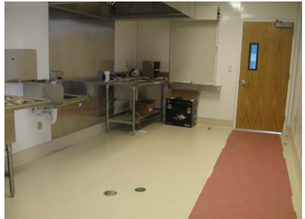
Refinished Epoxy Floor in Kitchen
