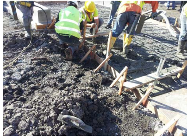
Concrete pour for walkway path posts & bench
