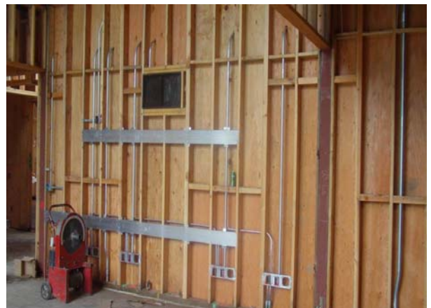
Classroom B119 Blocking Installation/Electrical Rough In
