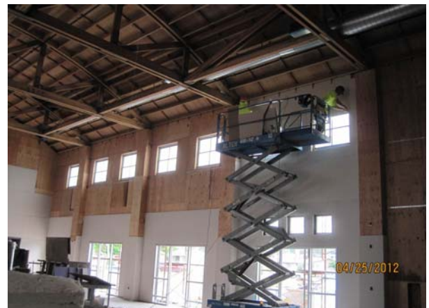
Building C - Hanging of Gypsum Boards
