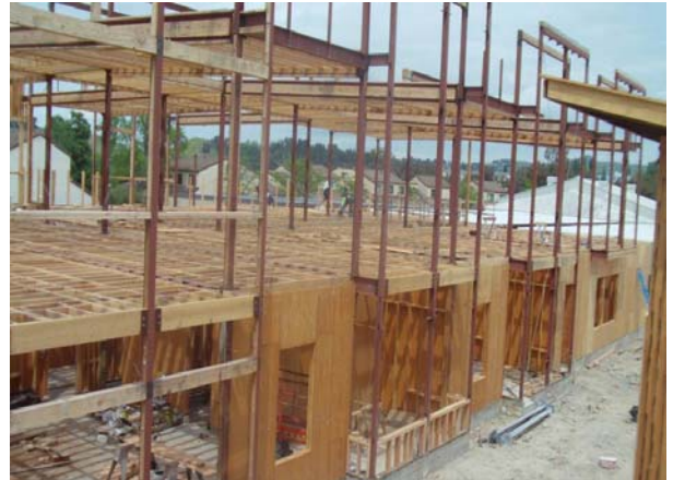
Building A Second Level Rough Framing
