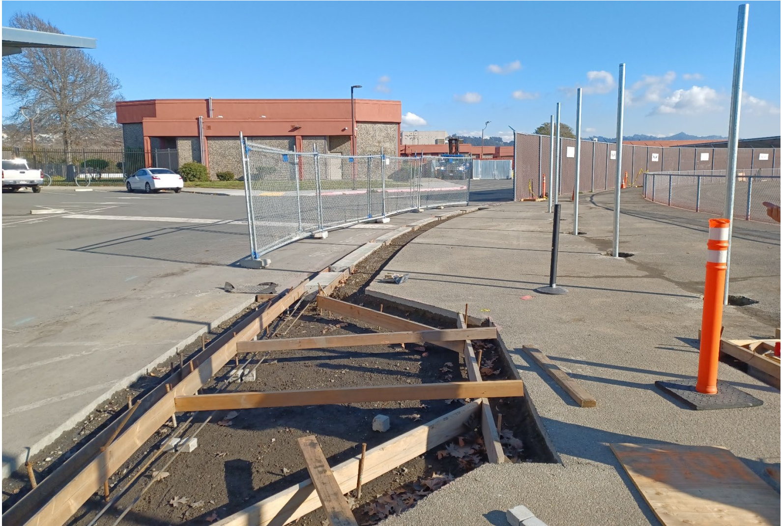
New Fence Post and Forming for New Curb and Ramp
