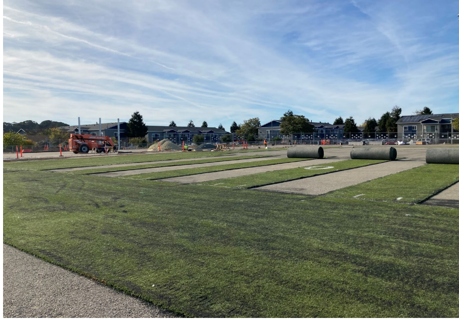
Removal of Existing Field Surface
