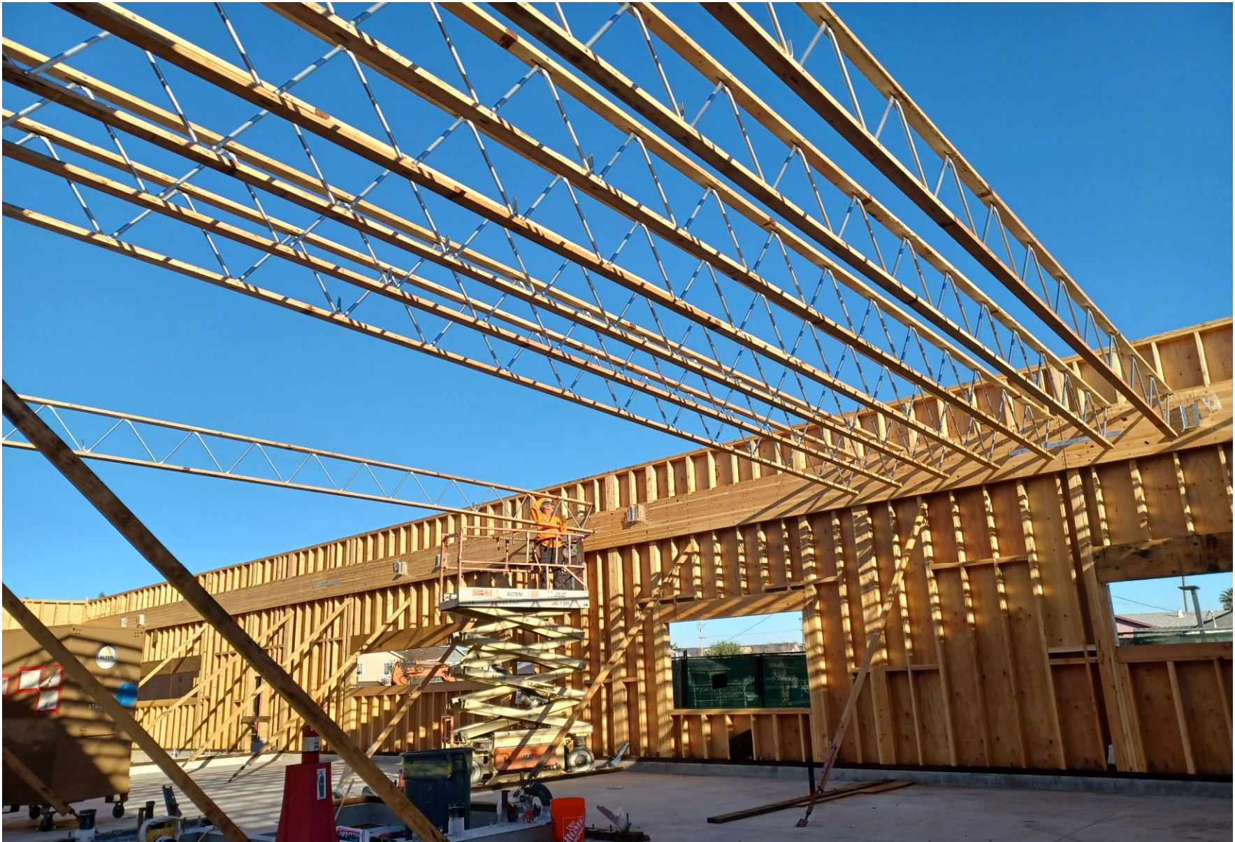
Building F – Setting Open Web Joist
