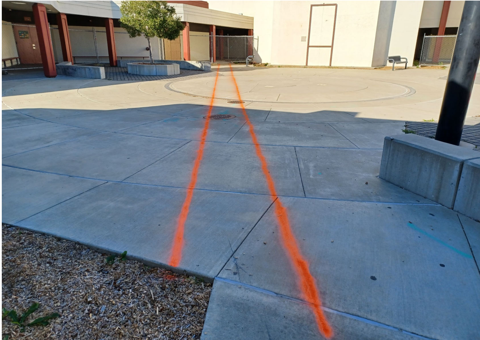
Layout for Utility Trenching
