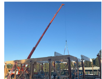
Craning a Beam into Place
