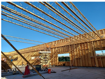
Installing Roof Joists
