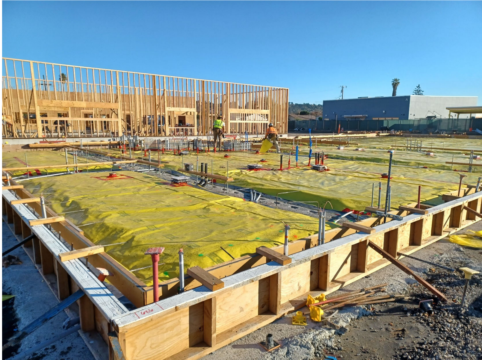
Building E – Exterior Framing, Building D – Preparing for the Building Slab
