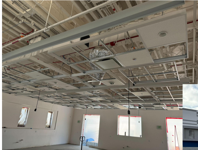
Installation of drywall and interior painting, completion of ceiling grid
