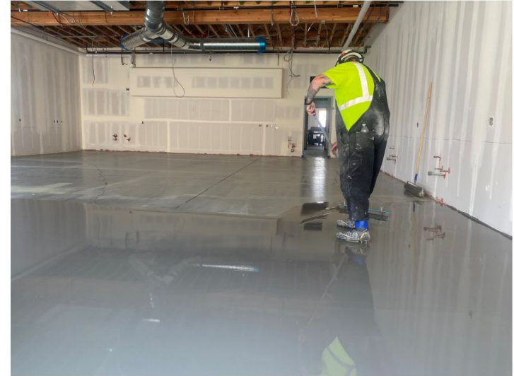
Applying moisture vapor control system in HS classrooms
