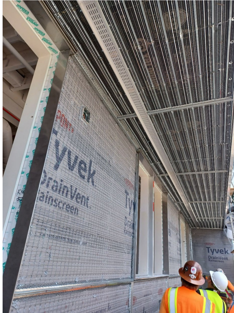
Waterproofing and Lath in Preparation for Stucco
