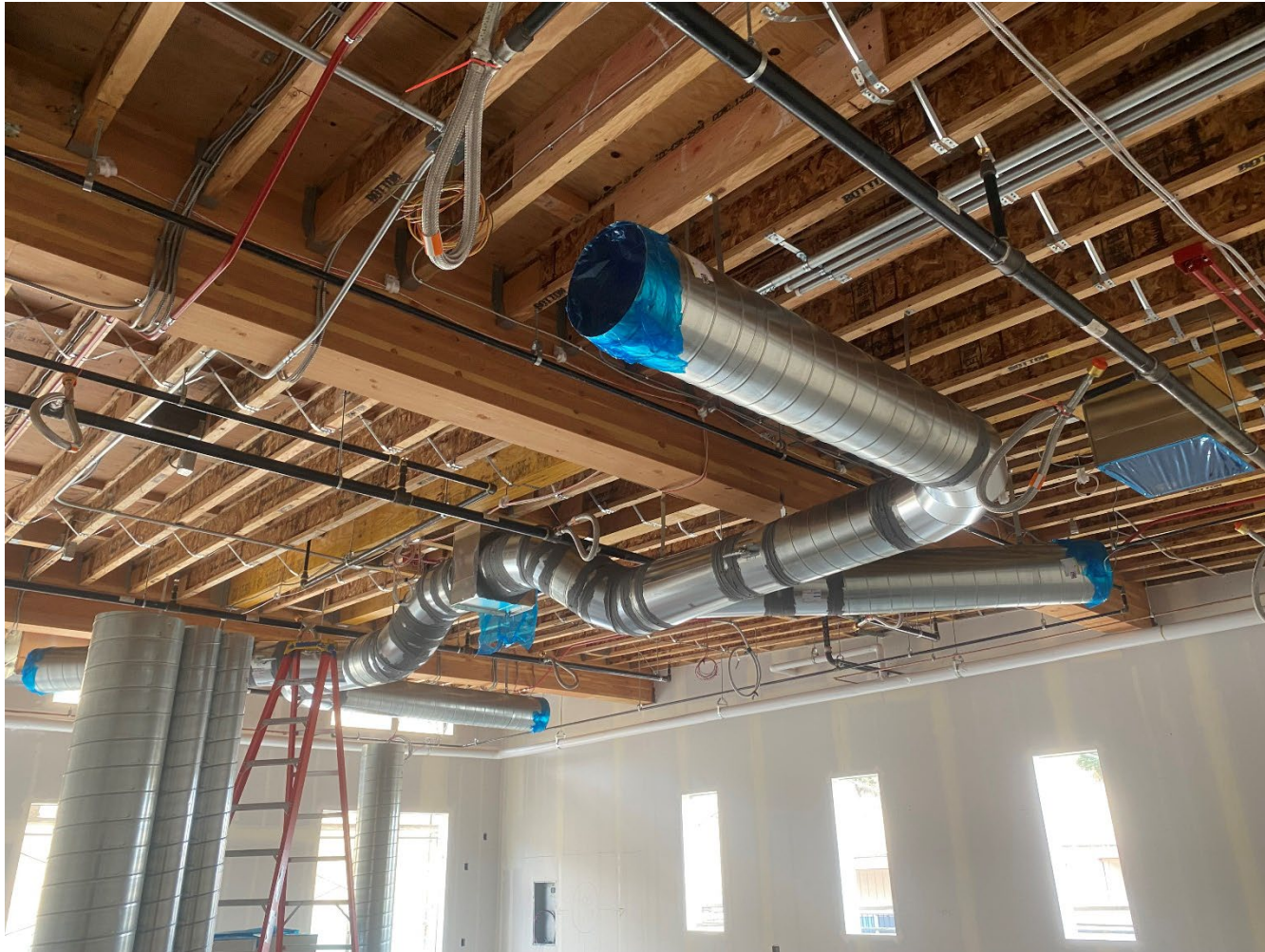
Installing Ductwork High School Side
