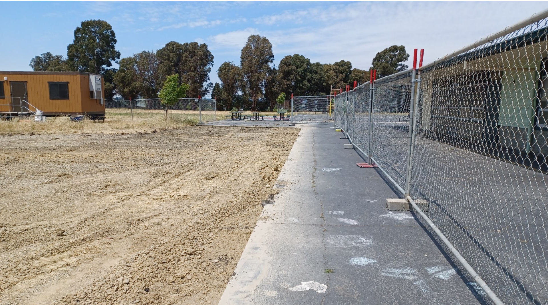
Removed Asphalt Paving
