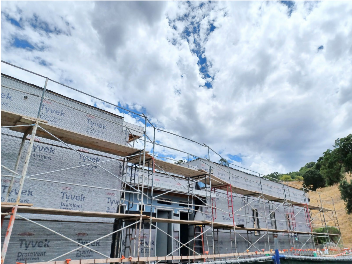
Waterproofing and Lath in Preparation for Stucco
