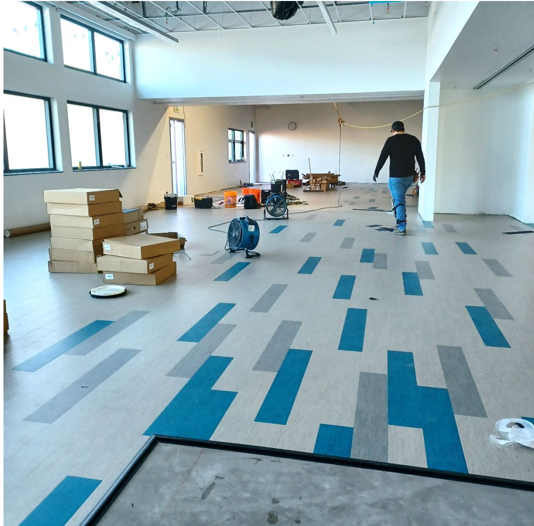
Building A – Installing flooring in the Library and Community Room
