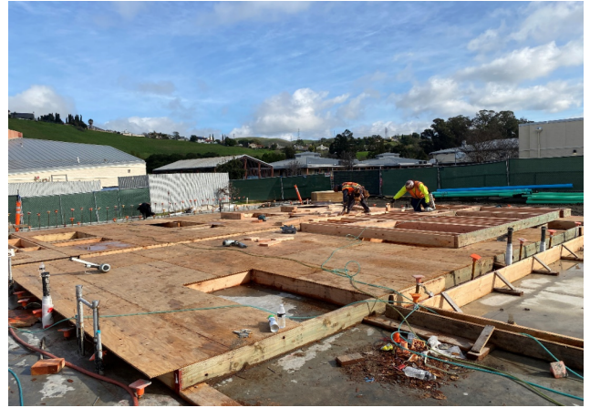
Install plywood on Middle School exterior walls
