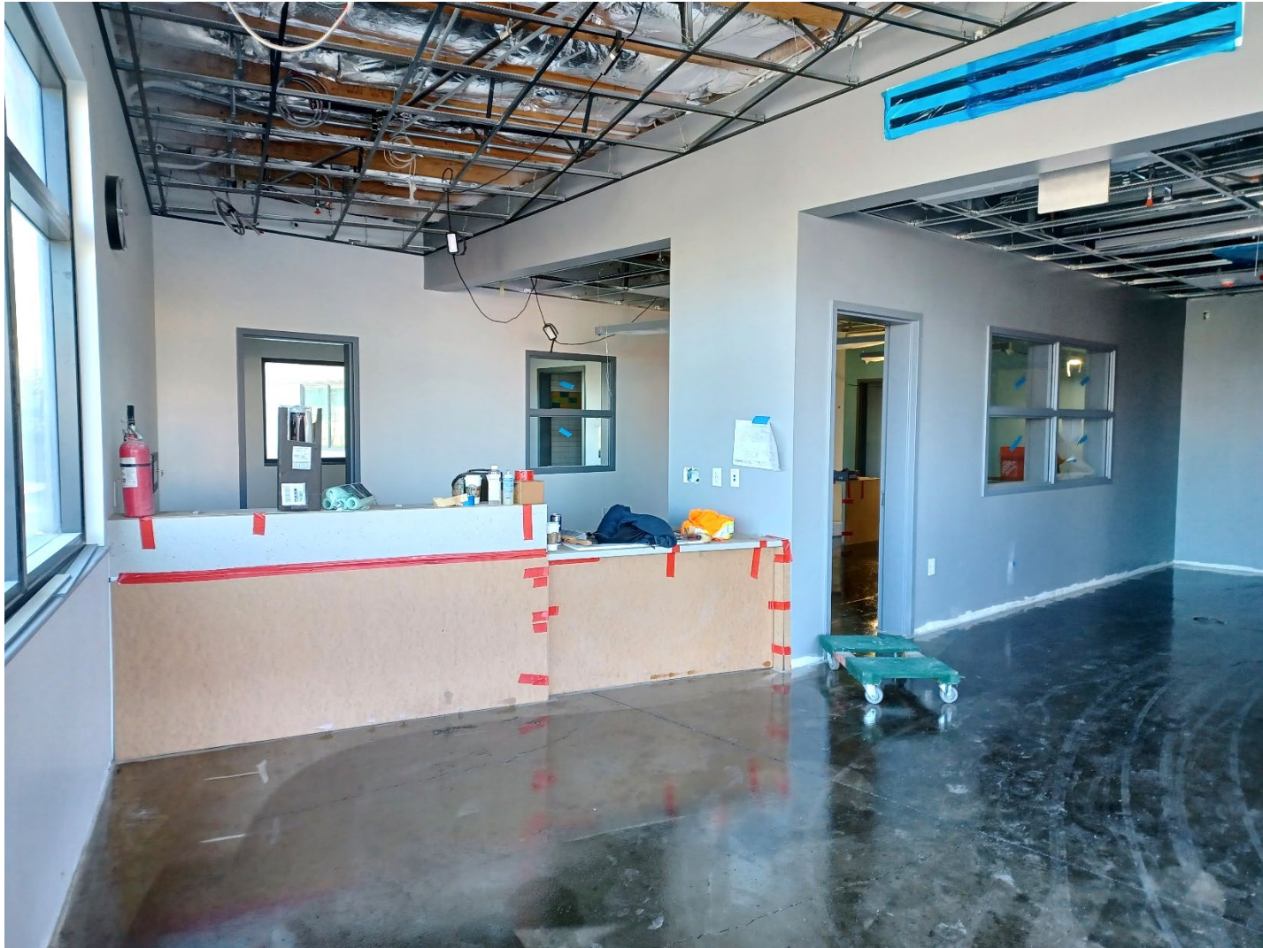
Building A – Front counter, glazing installed in interior windows, prepping for flooring
