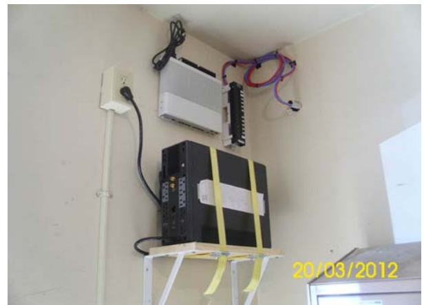
IDF installation in Building 500 of wireless system
