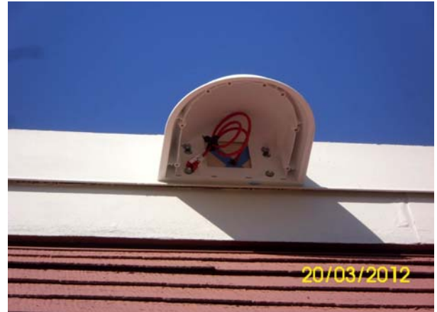
Camera mount with CAT 6 Cable
