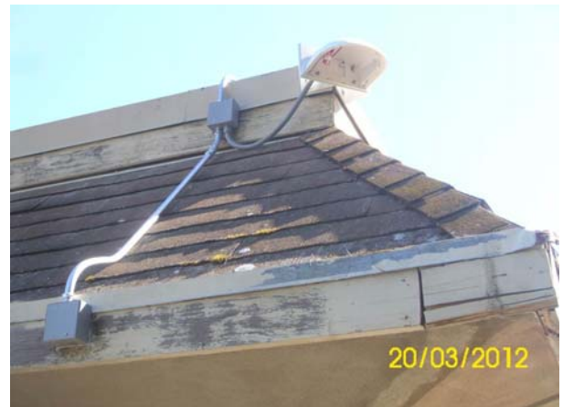
IDF penetrations with corner camera mount and conduit feed onto roof
