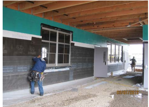
Building B - Vapor Barrier, Building Paper & Lath
