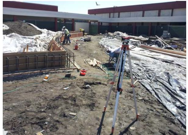
Seat Wall Forming at East Wall Quad
