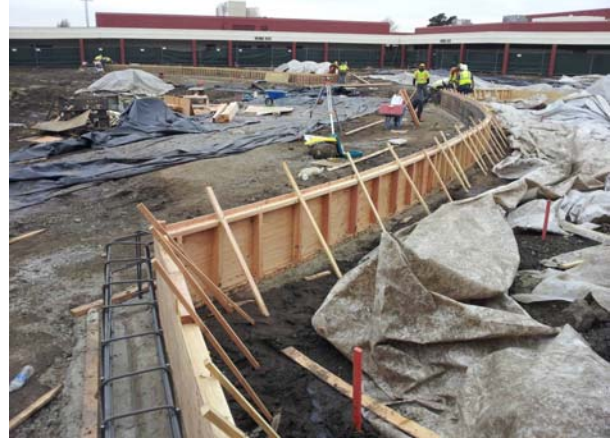
Seat Wall Forming at West Main Quad
