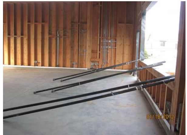
Building B - Fire Sprinkler Rough-in
