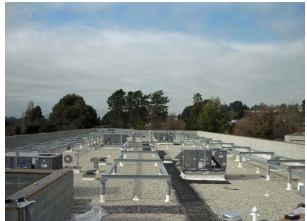
Building 5: Installation of Roof Gravel
