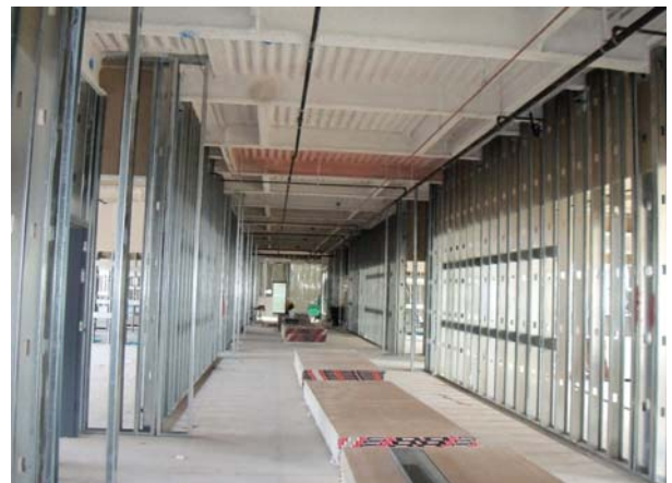
Building 6: Installation of Interior Metal Stud Framing
