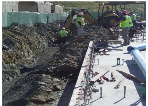
Trenching for Placement of Underground Utilities
