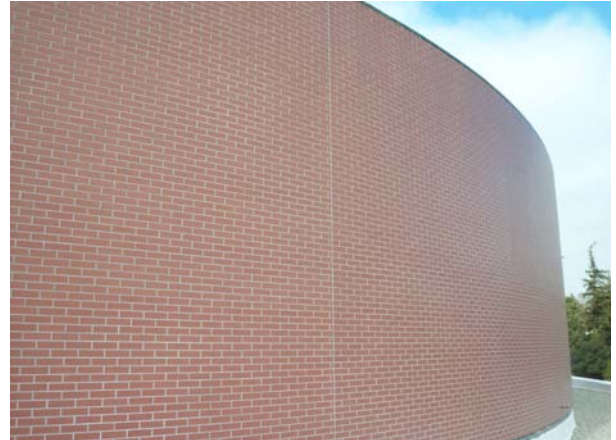
Building 2: Installation of Brick Veneer
