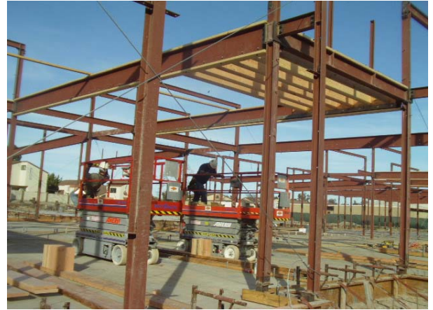
Installing Nailers and Wood Joists at Building B
