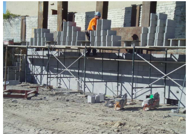
Formation of the Concrete Masonry Retaining West Wall
