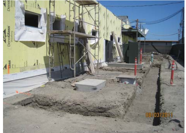
Footing for Trash & Electrical Enclosure
