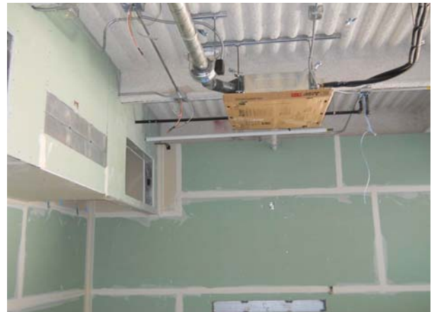
Building 9: Installation of Drywall
