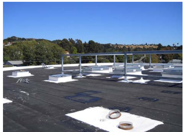
Building 2: Installation of Build-up Roof
