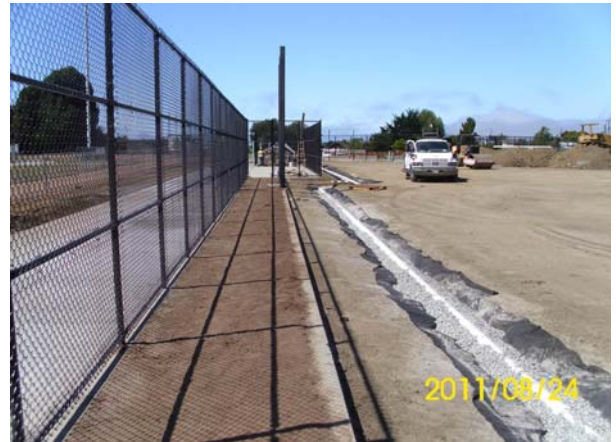
Perimeter fencing, loam perimeter track with adjacent field drain pipe
