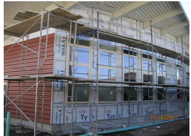
Radius Windows and Metal Wall Panels
