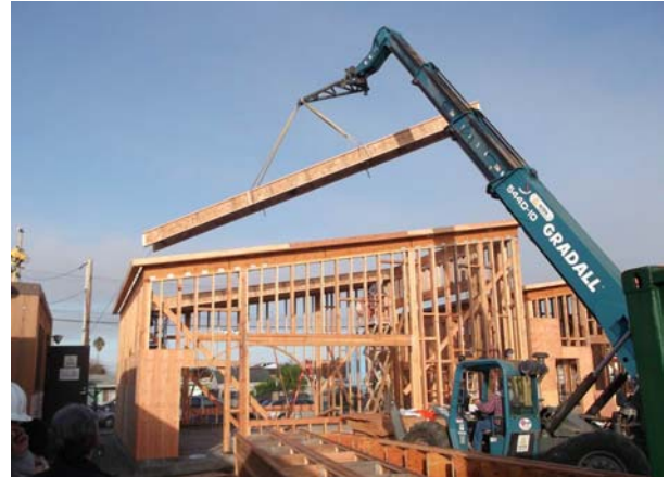
West Side of Site Framing & Installation of Joist - Building B
