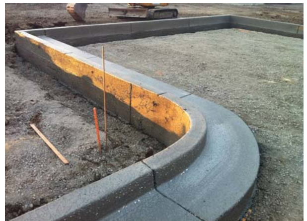
Finished Concrete Curb at Staff Parking Lot
