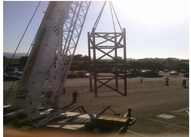
Setting of Elevator Frame
