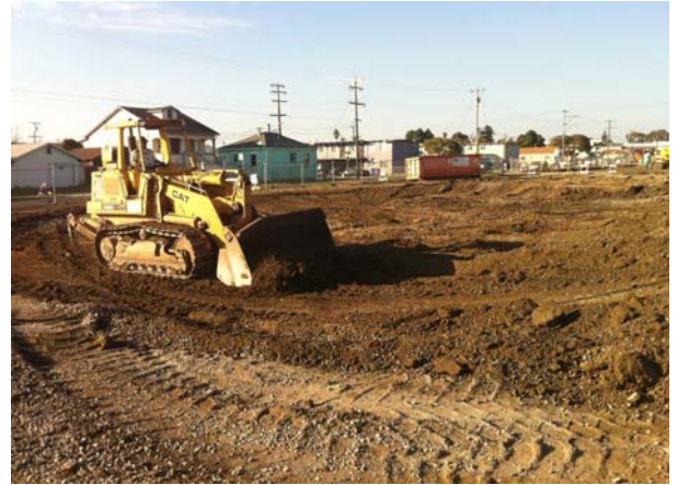
Rough Grading Work at New Play Field and Track
