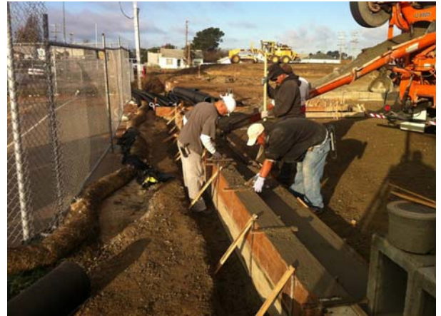
Concrete Curb Pour at Staff Parking Lot adjacent to MP Room
