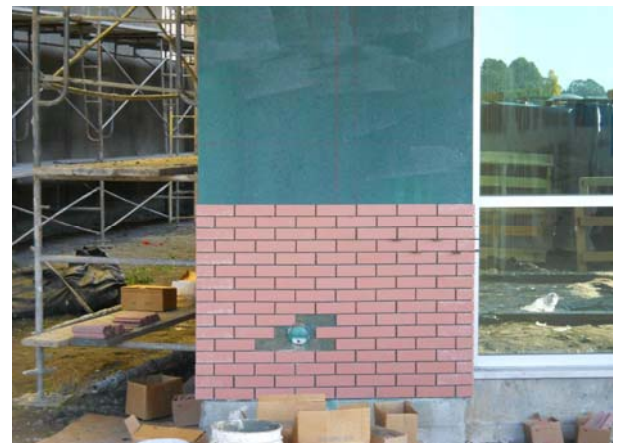
Building 9: Installation of Brick Veneer
