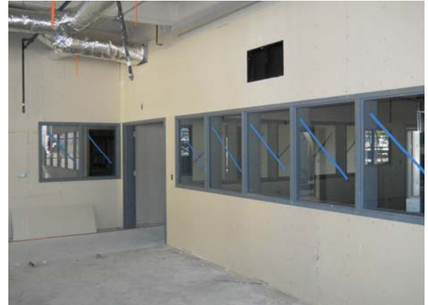
Building 1: Installation of Interior Windows
