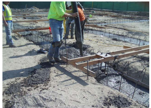
Building B Concrete Pour for Footings
