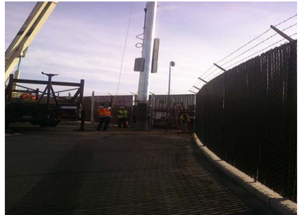
Mounting of Field Light Pole
