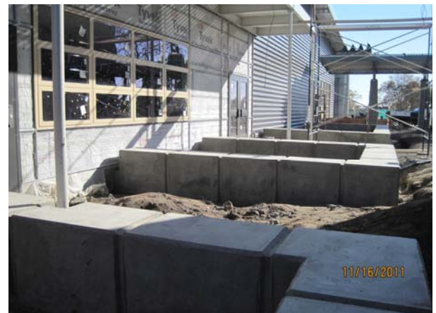
Site Grading and Planter Seat Walls
