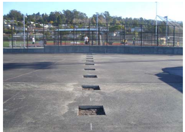
Tennis court paving complete fence post divisions cut for fence pole ...
