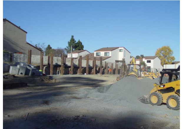
Shoring for Concrete Masonry Wall
