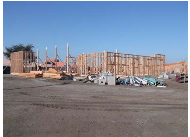
East Side of Site Wall Framing - Building C
