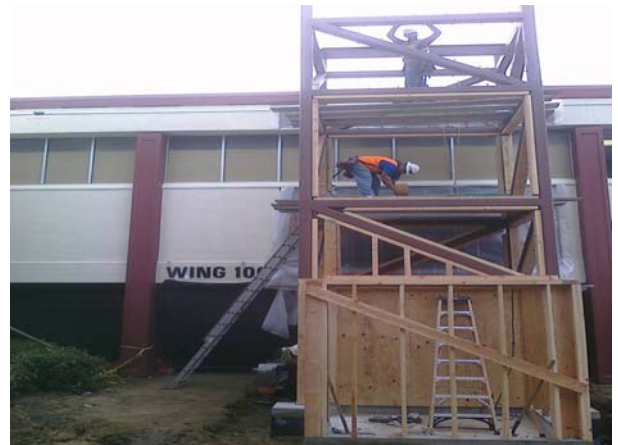
Framing for Elevator Cage
