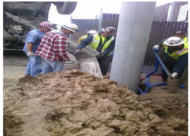
Field Lighting - Mounting of Field Light Bases
