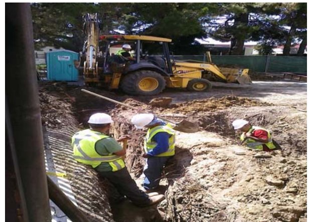
Trenching to Re-locate Storm Drain
