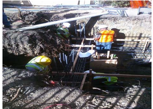
Framing for Elevator Pit
