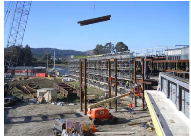
Building 12-Breezeway: Erection of Structural Steel
