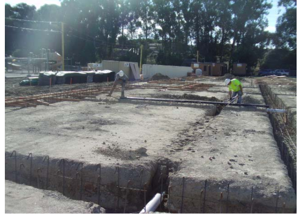
Rebar Installation for Building B Footings
