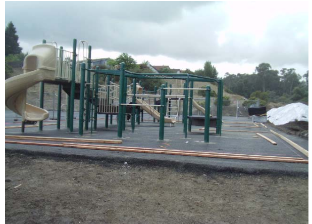
Forming Curbs at Temporary Play Structure
