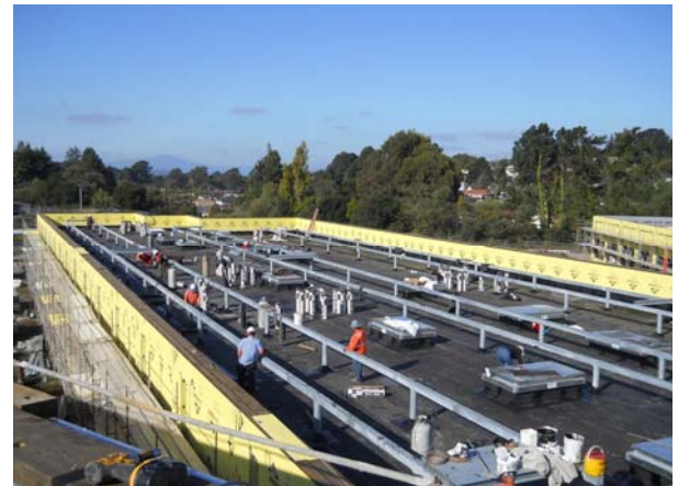
Building 6: Installation of Built-Up Roof
