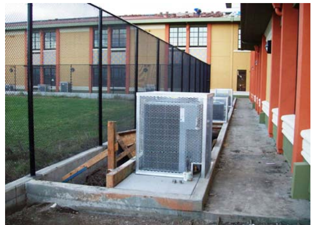
HVAC Units Mounted at the Rear of Building Areas A & B
