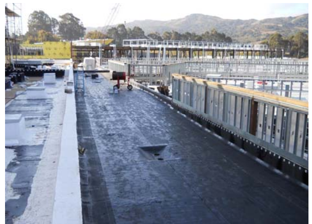
Building 11: Installation of Build-up Roof
