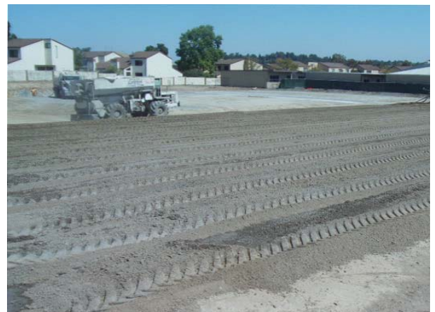
Building B Pad Lime Treatment
