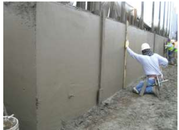
Shotcrete retaining wall at Ashbury Ave..
