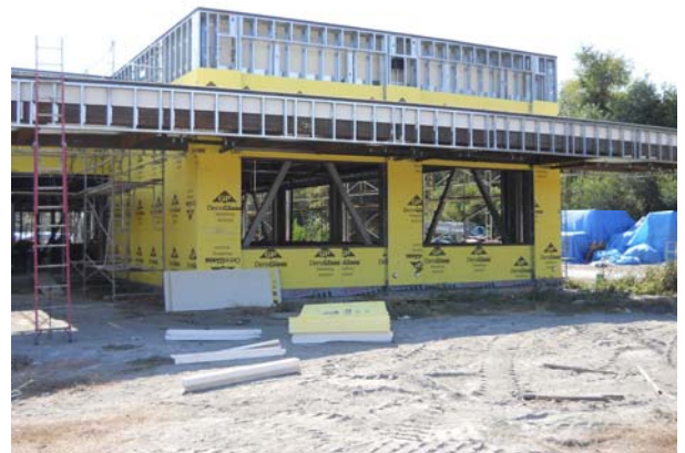
Building 3: Installation of Exterior Sheathing
