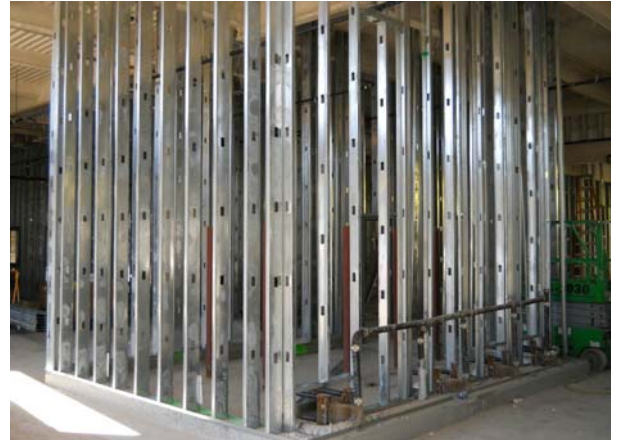
Building 1: Installation of Interior Wall Framing
