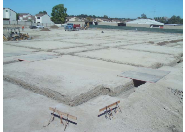
Trenching for Building A & B Footings
