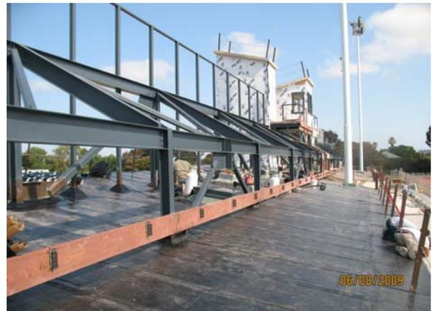
Torch down roof installed. Painted steel structure
