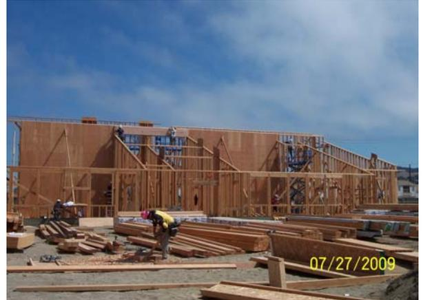
**Building A West Framing - Walls, Wall Ply, Glulam & I-joist**
