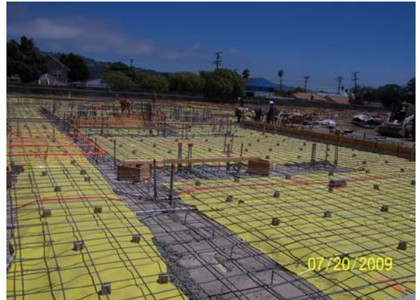
**Building A East SOG - Baserock, Vapor Barrier & Rebar**
