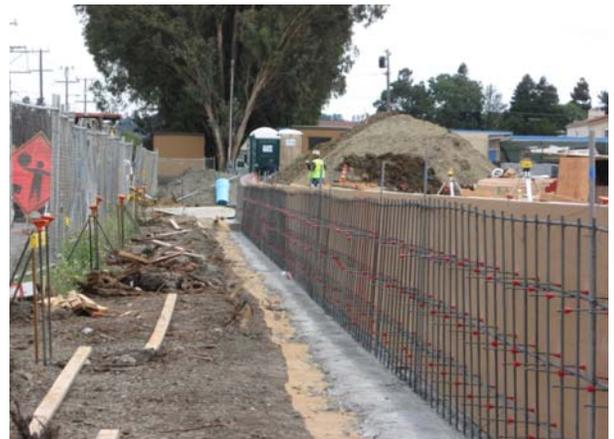
**Installation of Footing Rebar and Stem Wall**
