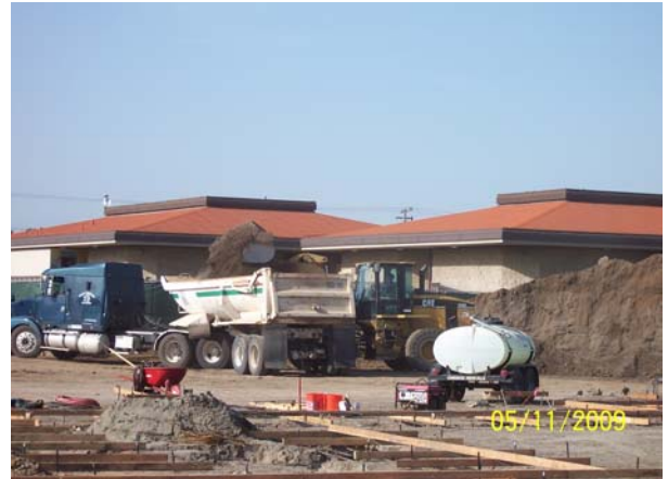
Off-haul of excavation spoils
