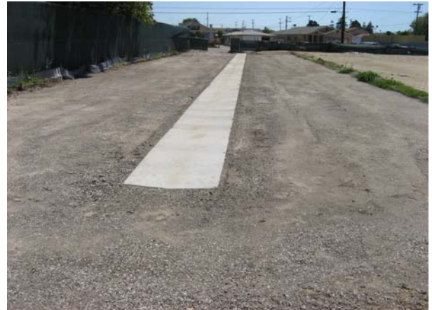
Increment 1A-Concrete Swale and Parking Area-COMPLETED
