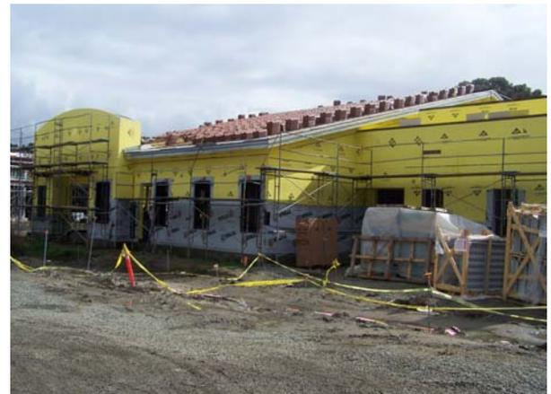
Finished Installation of Exterior Gyp Sheathing at Bldgs. MC/A
