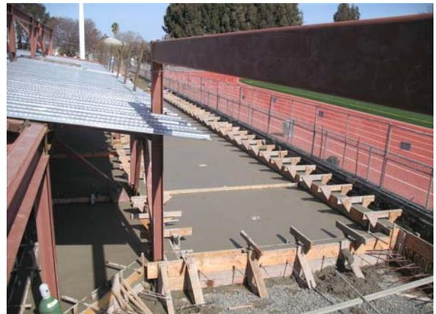
2nd Floor metal decking & new concrete slab
