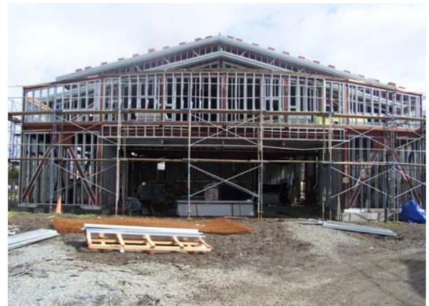
Finished Metal Stud Framing at Bldg. M
