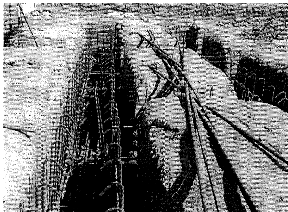
Installation of grade beam rebar
