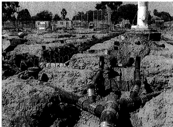
New rough plumbing under building slab
