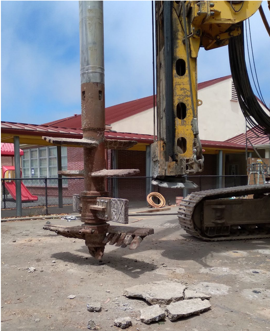
Mixing auger and creation of stabilization columns
