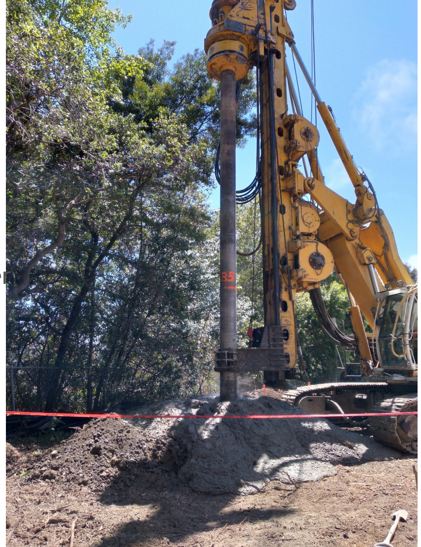
Mixing auger and creation of stabilization columns
