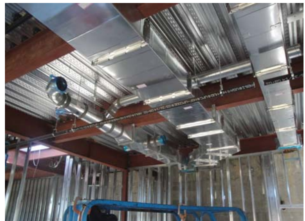
Locker Room Metal Framing and Mechanical Ducts
