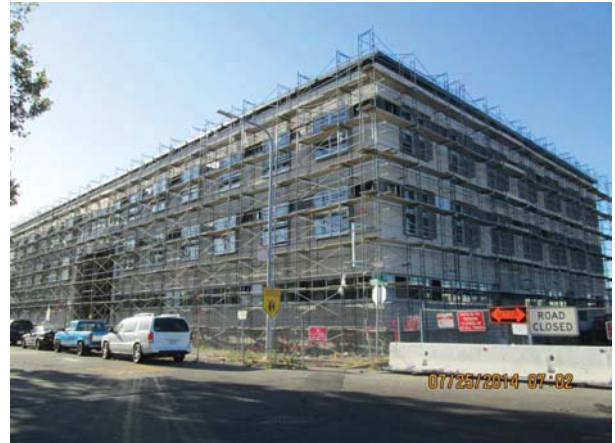
Building A - Plaster completed at west and north sides
