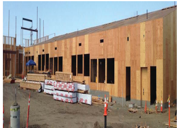
Building C Exterior Framing (West)
