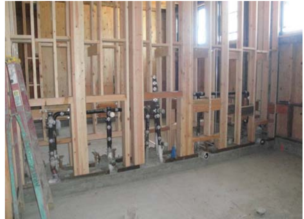
Building A Bathroom Framework and Plumbing
