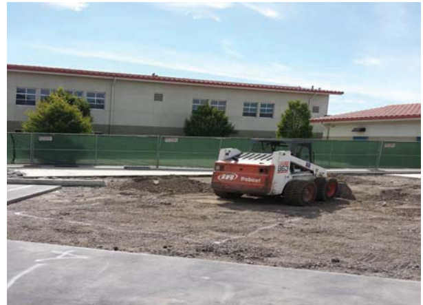
Recycling Center - Site Demolition-2
