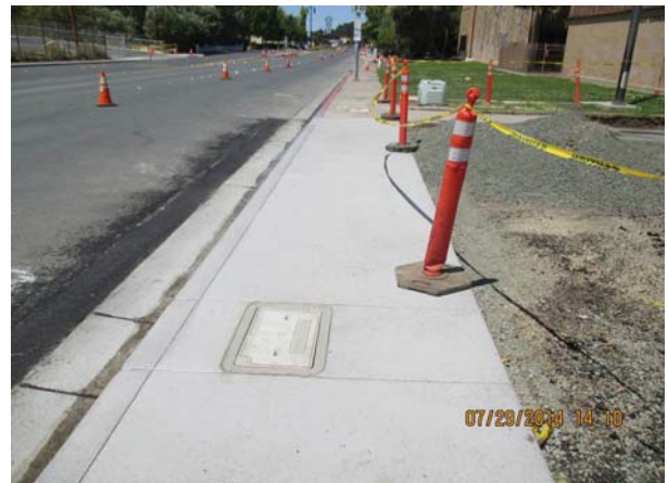
Finish Sidewalk at Library
