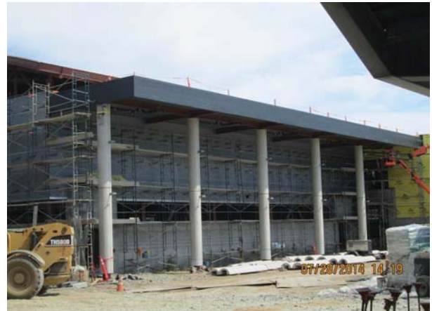
Building B - Pre-cast concrete column covers installation
