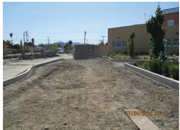
Subgrade at Bus Turnout
