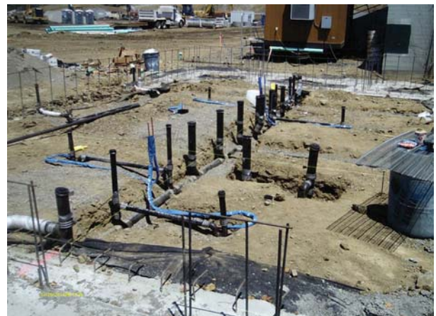
Building D rough in under slab plumbing
