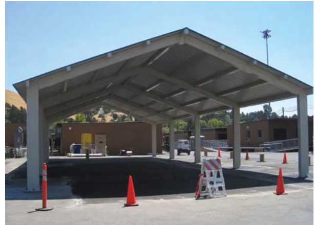
Installation of Shade Structure
