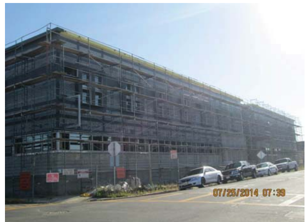
Building C - Rain screen at South side
