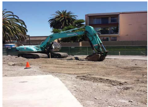
Recycling Center - Site Demolition-3
