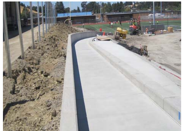
Walkway at Plateau - Concrete Poured
