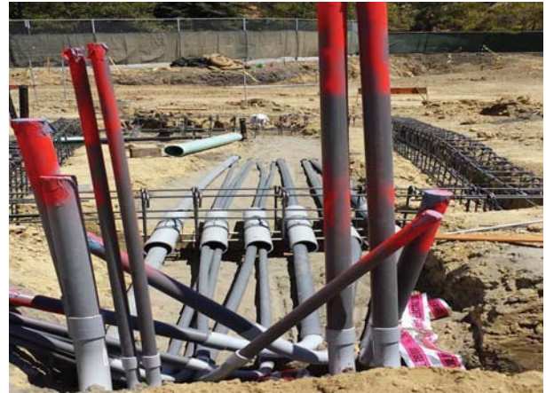
Electrical Stub-ups at Restroom Building
