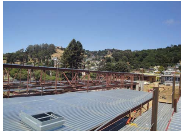
Building B Roof Metal Deck & Building C Structural Steel
