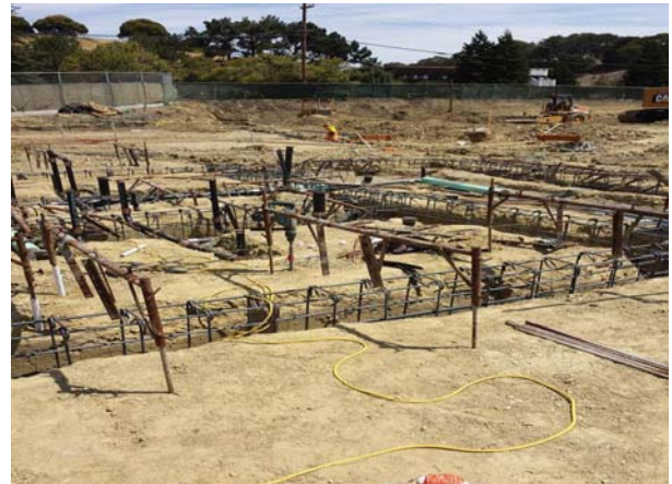
Rebar for Footings at Restroom Building
