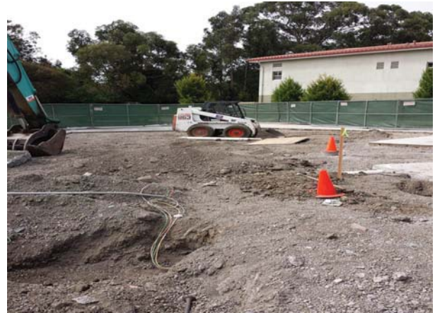
Recycling Center - Site Demolition-1
