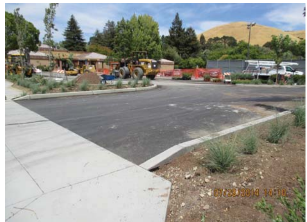
Paving at Library
