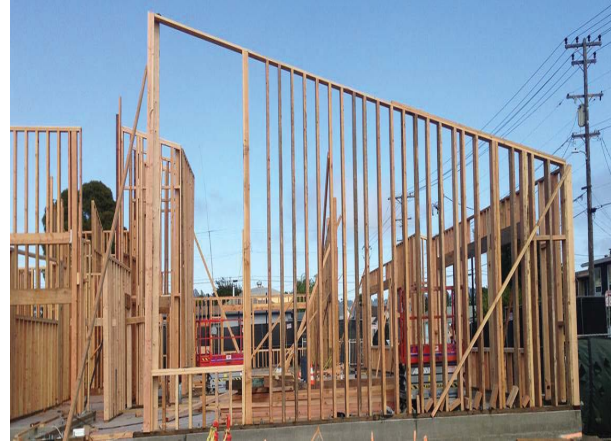
Building K Wall Framing
