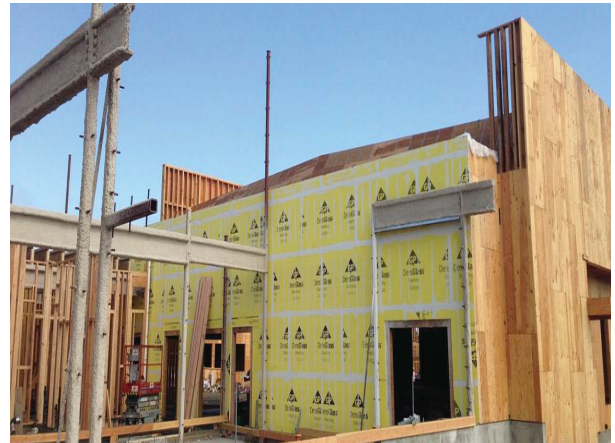
Building M Drywall Installation
