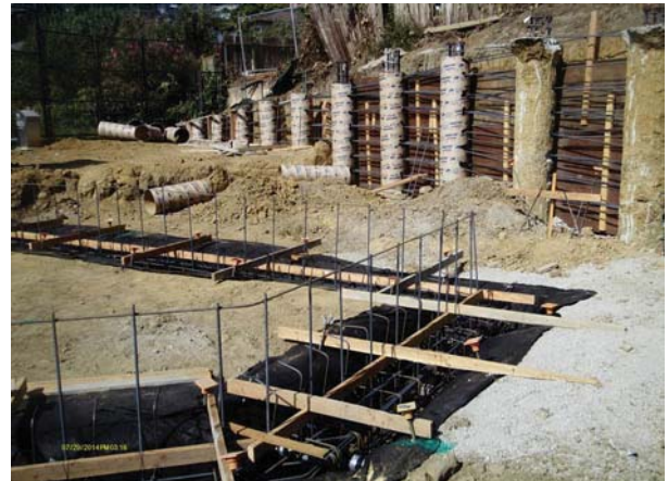
Building B footing complete & retaining wall
