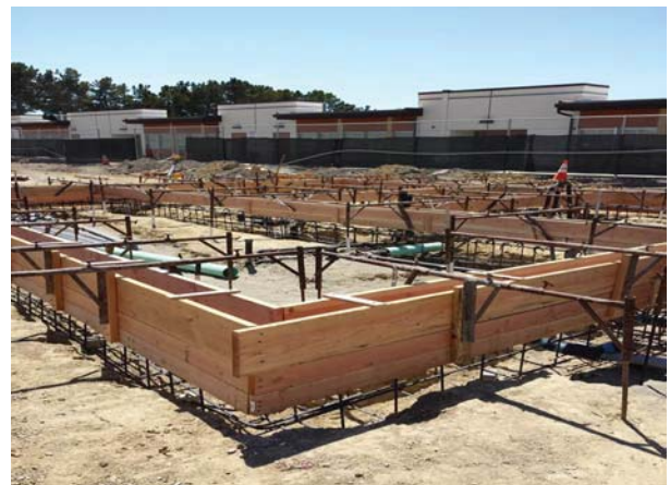
Footing Forms at Restroom Building
