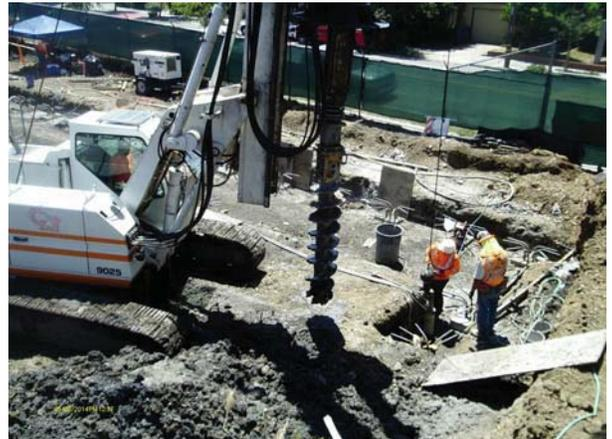
Drilling rig set-up for a 33'-0" deep concrete pier
