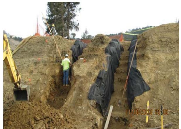
Building C - Step Footing Excavation
