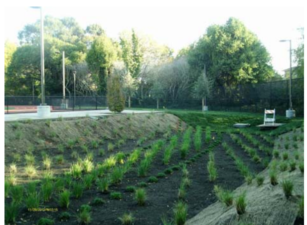
Landscaping completed at the southwestern bio swale
