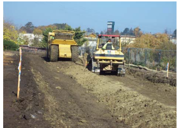
Excavation for Detention Basin
