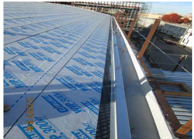
Building B - Roofing
