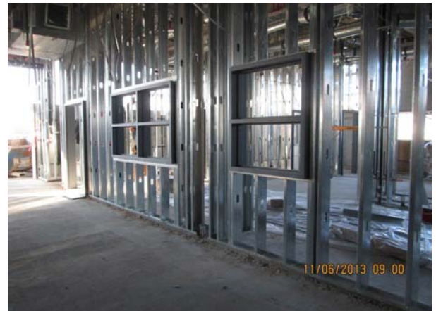
Building A - Interior Metal Stud Framing
