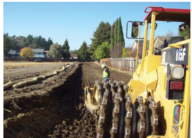
Placement of fill in North & West slopes
