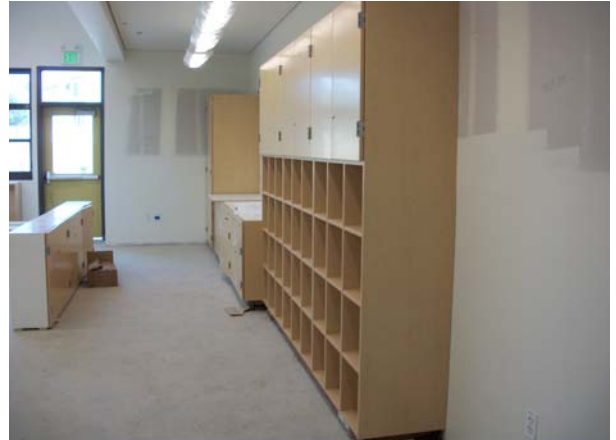
Building A - Casework & Finishes
