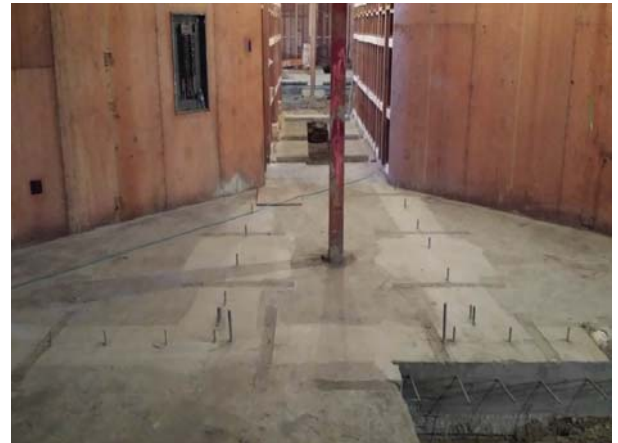
Poured Footings & Dowels
