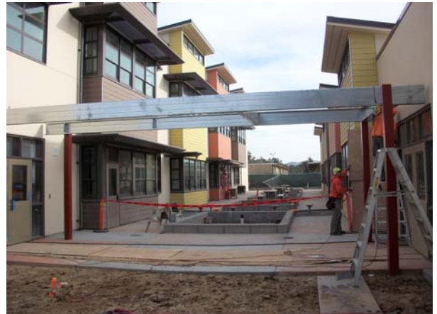
Covered Walkway from Building A to B
