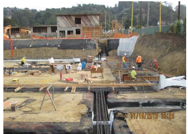
Building B - Footings
