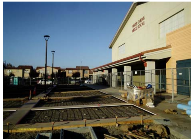
Concrete flatwork between Community Center and Gym ready for pour
