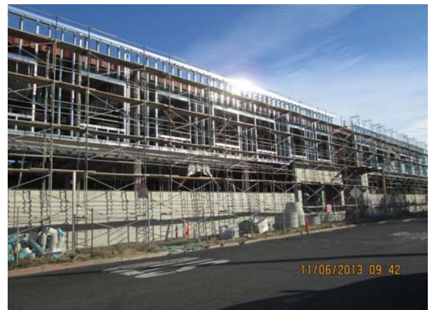
Building C - Exterior Metal Stud Framing
