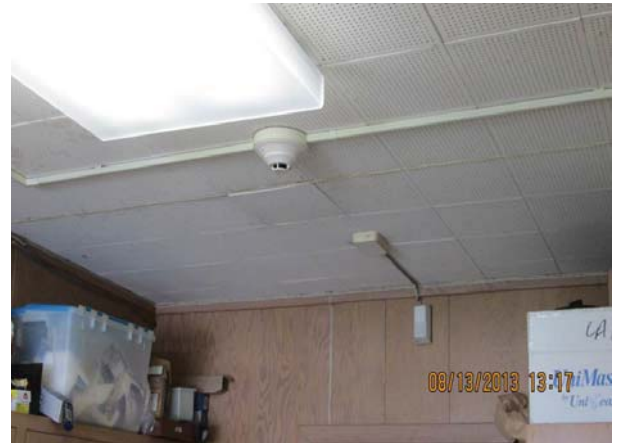
New Smoke Detector in Principal's Office
