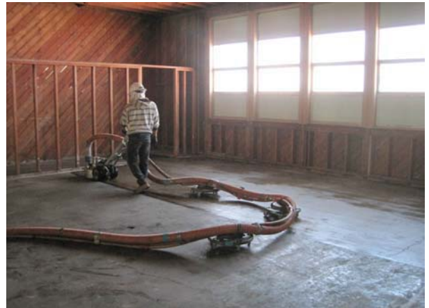
Water Pressure Clean Concrete Floors
