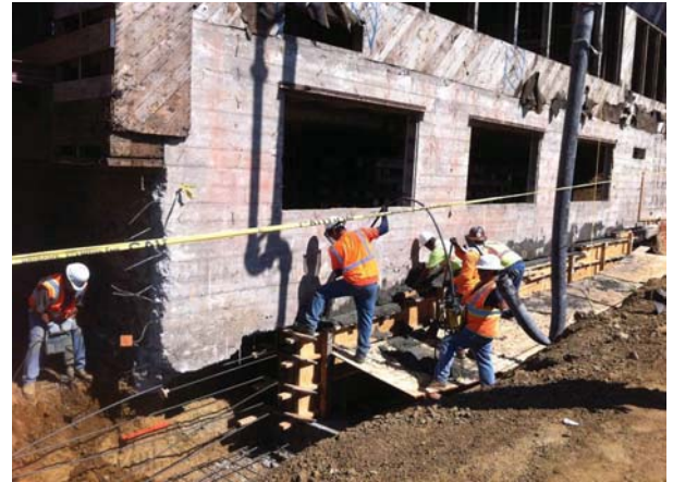
Lowering of Building A Basement Slab & Footings 70%.
