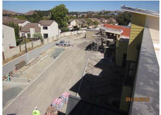
Building A - North side curbs & grading
