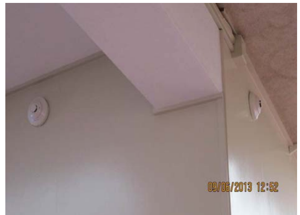
New smoke detectors in classroom corridor
