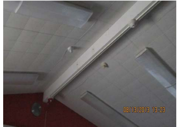
New Hornstrobe and Smoke Detector in Kindergarten Bldg.
