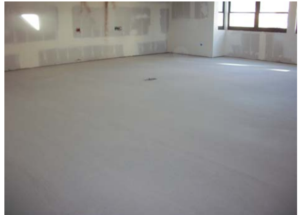
Building B - Classroom floor leveling
