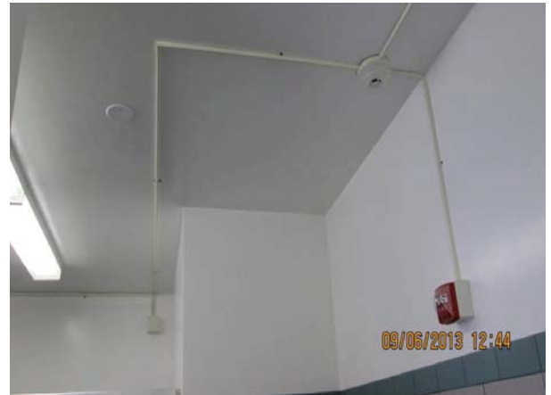
New devices in restroom
