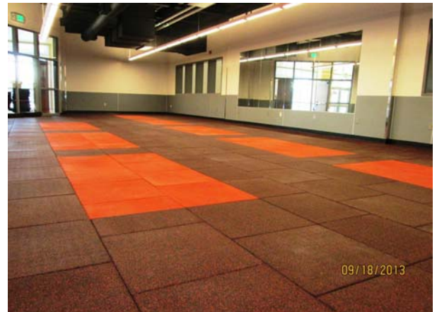
Installation of Fitness and Weight Room Flooring
