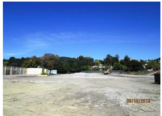
Demolition of Existing Campus 200 & 300 Wing
