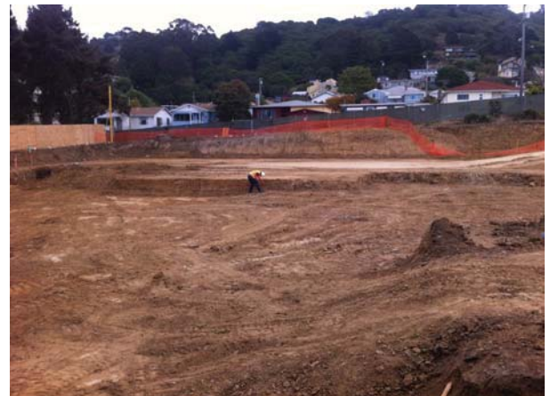
Building D Pad Engineered Fill
