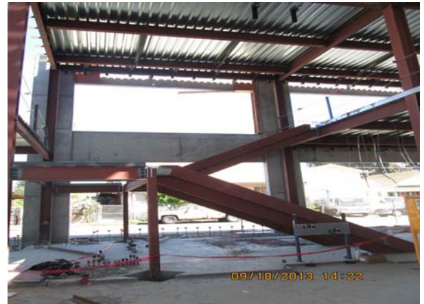
Building B - East stair installation
