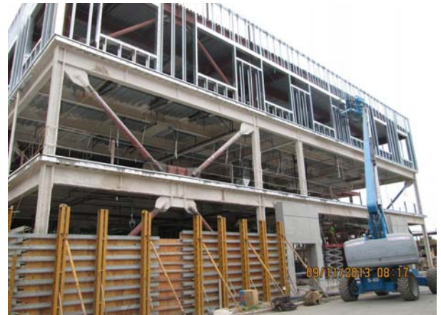
Building A - Metal stud installation & arch walls
