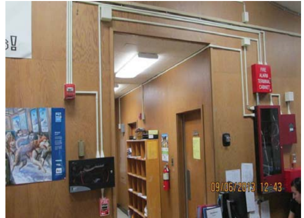
New FACP and Annunciator Panel in Administration Office
