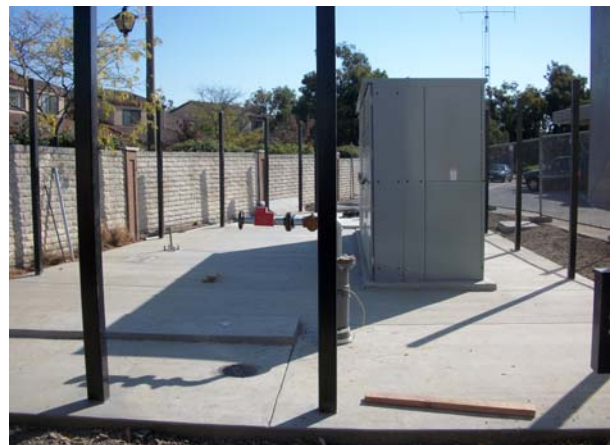
Building C - Utility yard/switchgear
