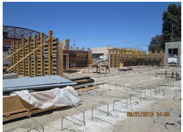
Building C - Architectural Concrete Walls
