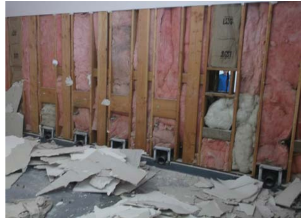
Downer Restroom Demolition - IN PROGRESS
