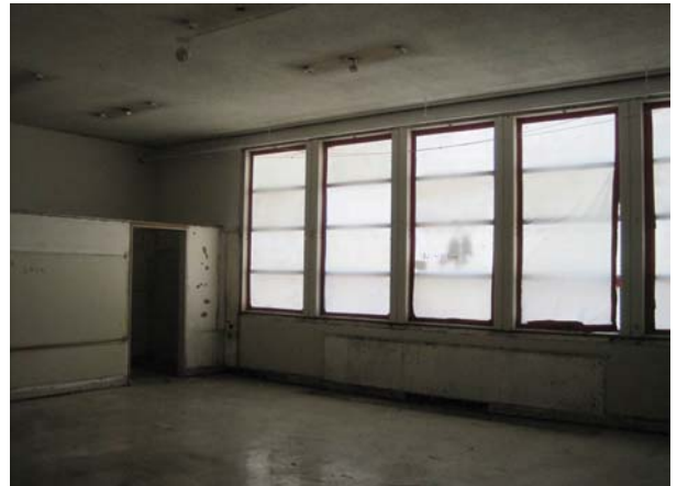
Typical Classroom with Trims Removed
