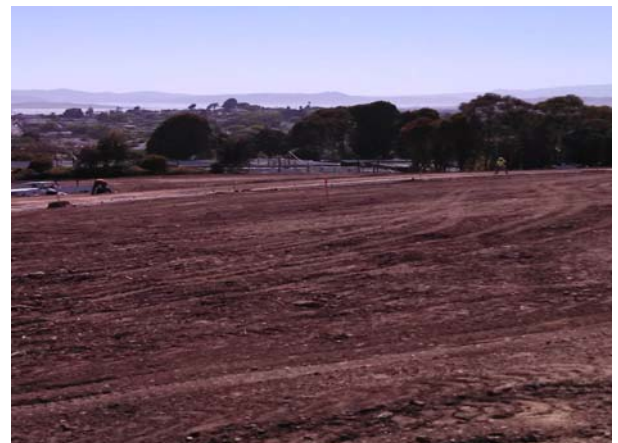
Finish Grading operations at the North East corner
