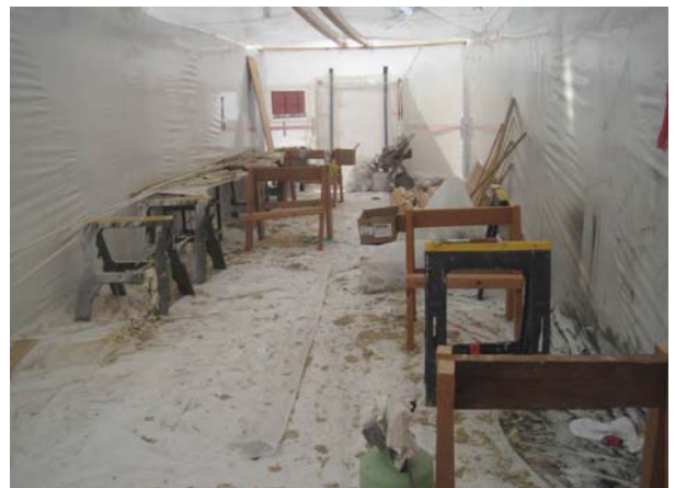
Trim Lead Paint Removal Room
