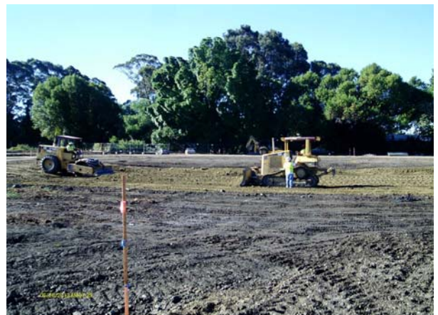
Chlordane pit has been backfilled and ready for non expansive soil.
