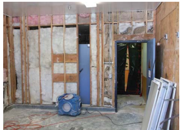
Downer Restroom Demolition - IN PROGRESS
