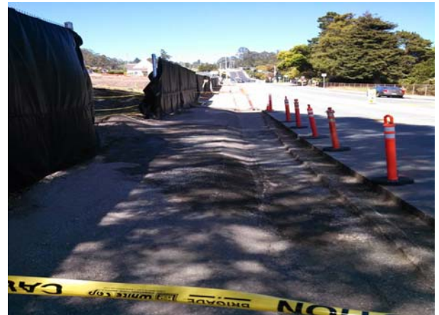
New curb installation at North West corner
