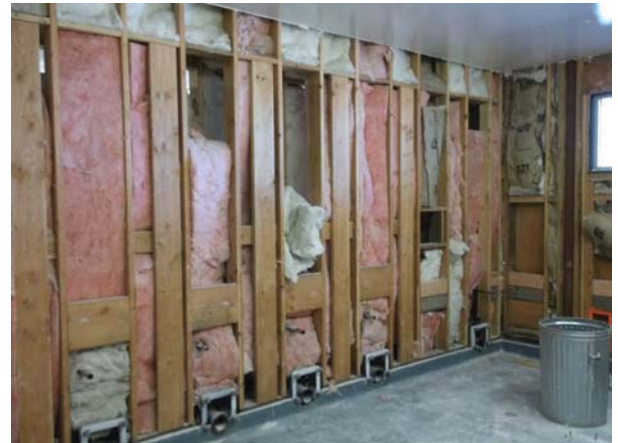
Downer Restroom Demolition - IN PROGRESS
