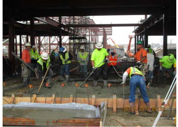
Building A - SOG
