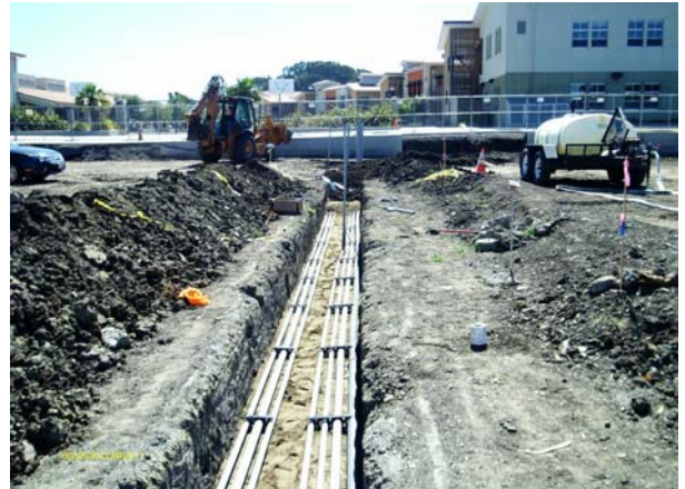
Electrical trenching and conduits installed.
