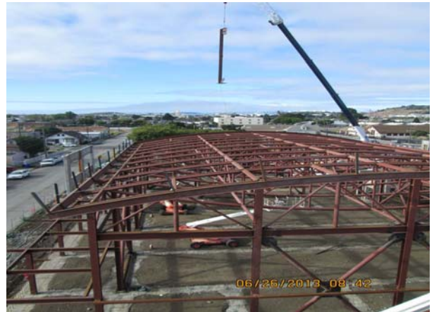
Building B - Steel Erection South Side
