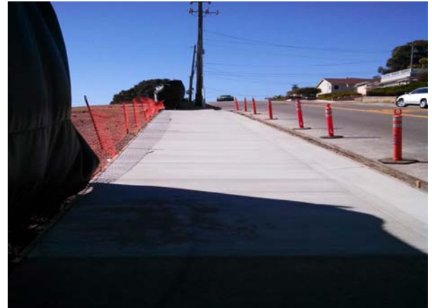
New curb at North East Corner
