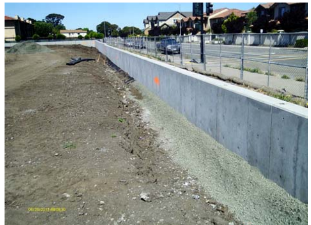
Concrete retaining wall at Road 20 complete with drain rock.
