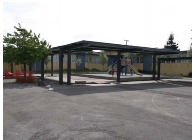
Phase 3 Covered Canopy - COMPLETE
