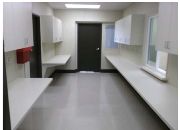
CCS @ Downer-Interior Punchlist Work - COMPLETE
