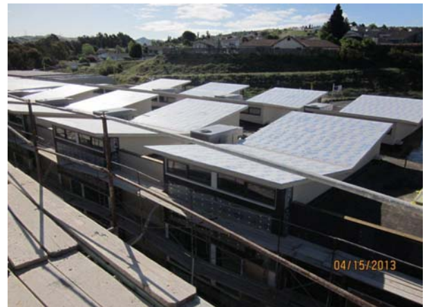
Butterfly Roof 2nd Layer Underlayment
