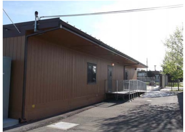
CCS @ Downer Portable, Fencing, & Container - COMPLETE
