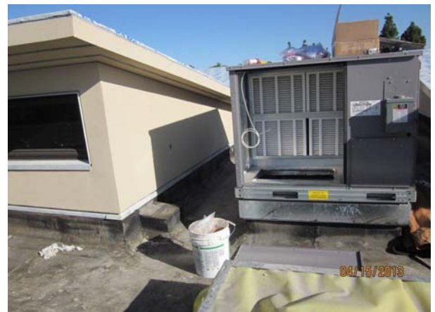
HAVC Units / Stucco at Rooftop
