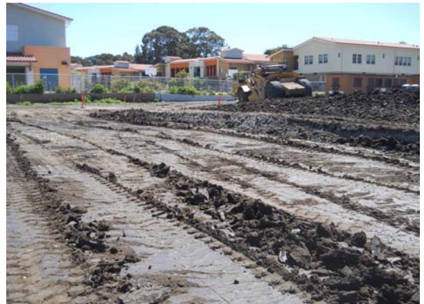
Soil excavated by scraper at Community Center Pad
