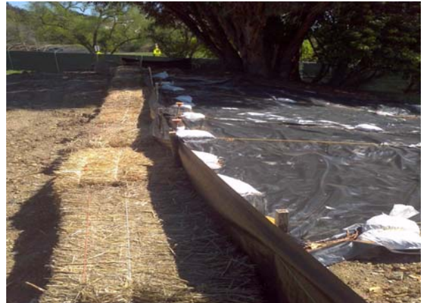
SWPPP measures @ South West corner of site
