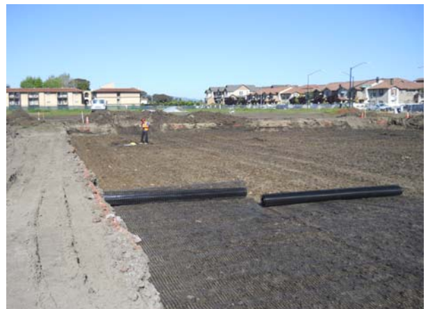
Community Center Pad compacted with Geotech Fabric
