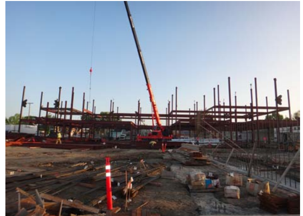
Building A - Progress of Structural Steel
