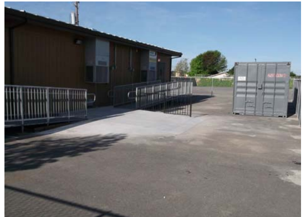
CCS @ Downer Portable, Fencing, & Container - COMPLETE
