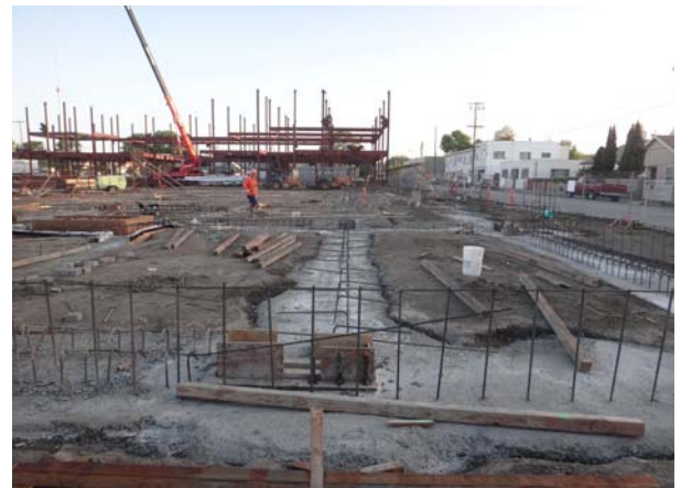
Building B - Grade Beams Poured
