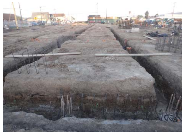
Building C - Grade Beam Trenches & Rebar Being Installed
