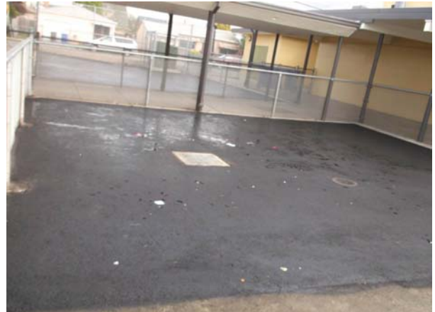
Site Work & Asphalt - COMPLETE
