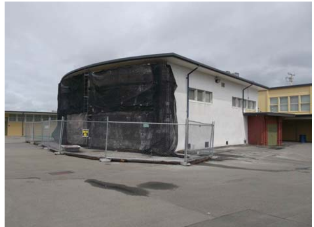
Bldg. E - Installation of Stucco - IN PROGRESS
