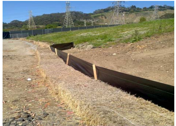
Bottom of the hill at the AC paving
