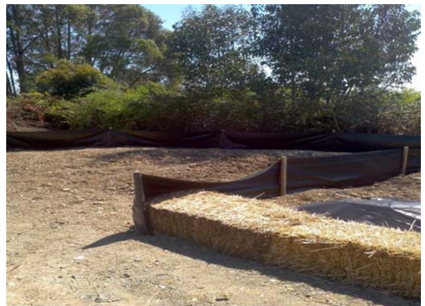
SWPPP measures between the two lower staircases
