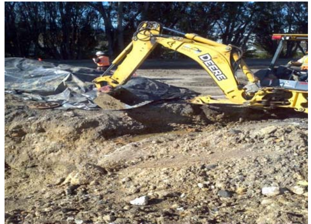
UST Pit additional excavation
