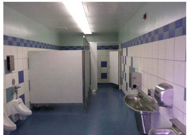
Restroom Renovation 11(B & G) - IN PROGRESS
