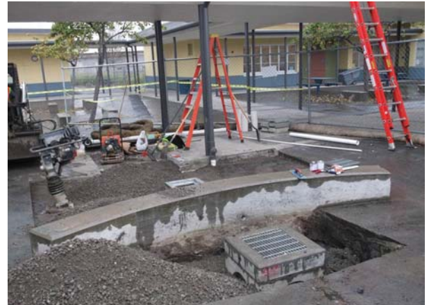
Installation of Underground Storm Drains - IN PROGRESS
