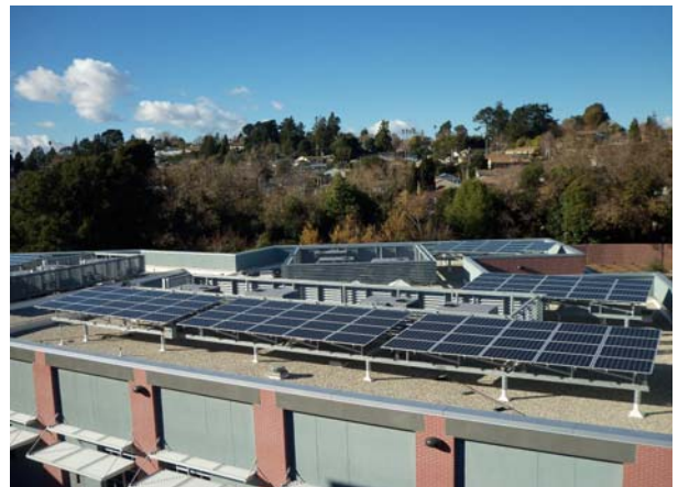
Building No. 3 Roof - PV System Panels
