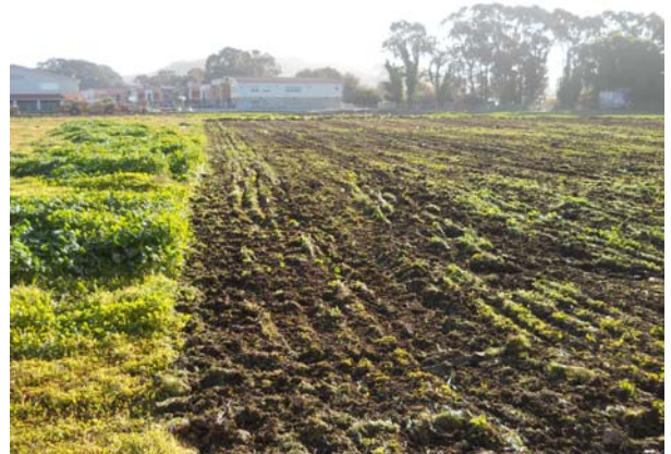
Clearing and Grubbing existing weeds and bushes
