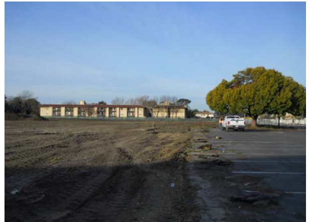
Site clearing and fence demolition
