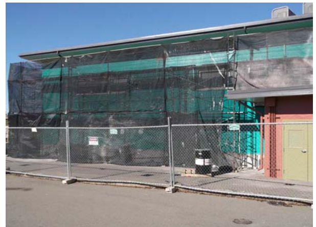
Bldg. E - Installation of Stucco - IN PROGRESS
