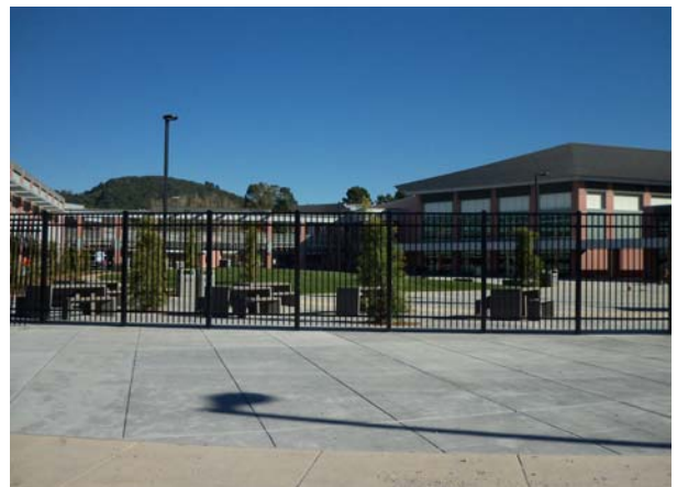
Site Work - Ornamental Fence
