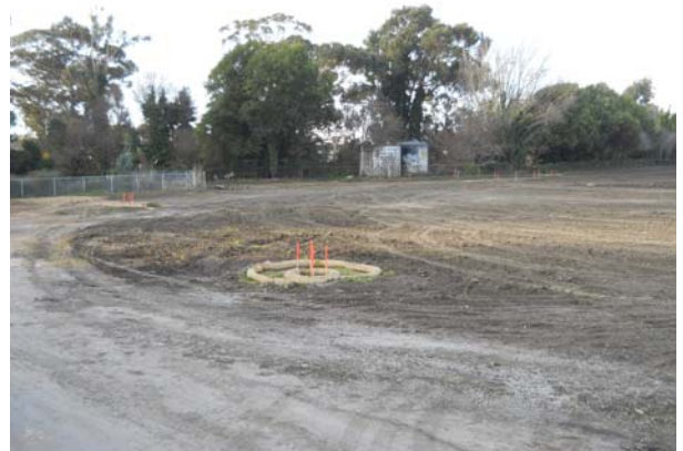
Storm water protection measures installed.
