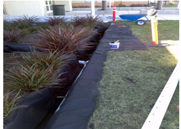
Trench and filter fabric at North side of Campus
