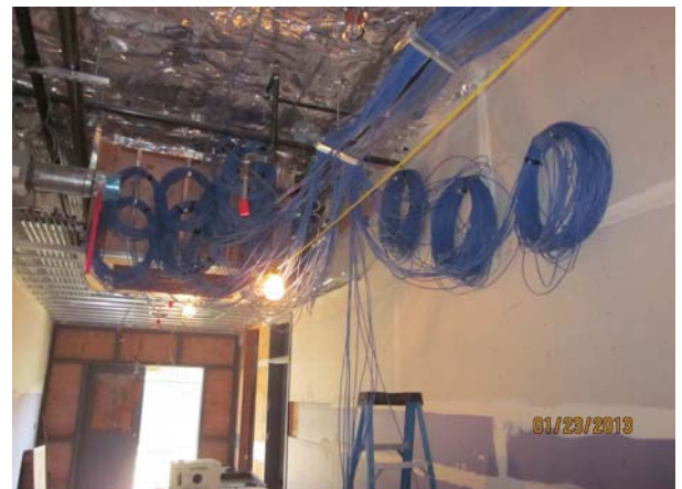
Ductwork in Building A
