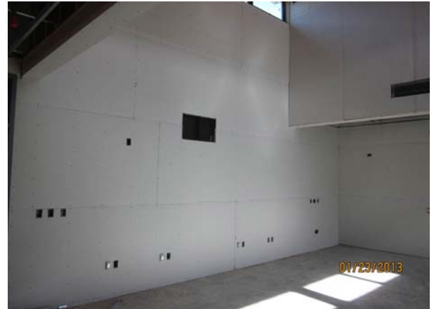
Clerestory Window Installation on Building B
