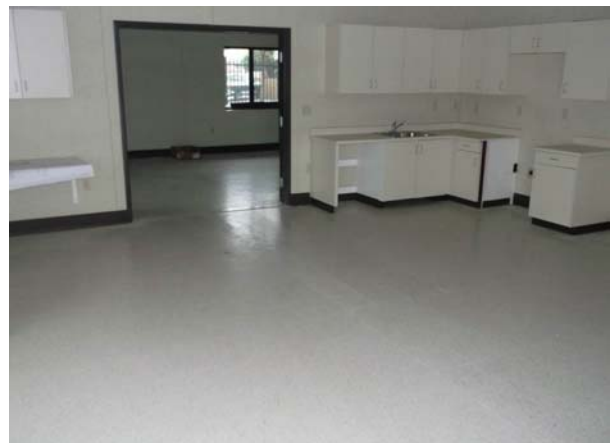
CCS @ Downer-Cabinet Installation - COMPLETE
