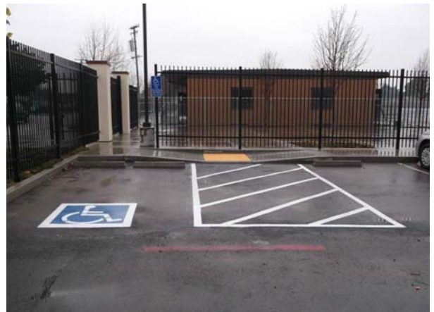
CCS @ Downer- ADA Parking & Gate Opening - COMPLETE
