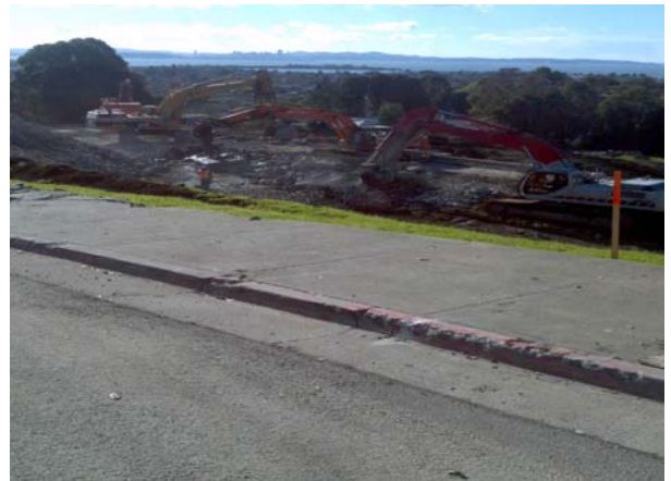
Concrete & rebar removal Main Classroom Building
