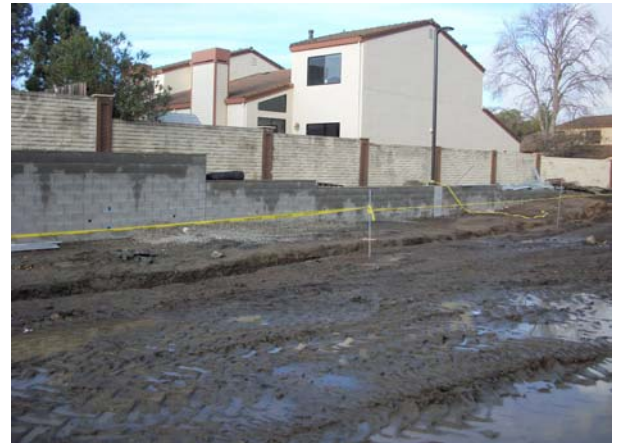
PG&E Joint Trench for Gas & Power
