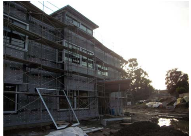
Clerestory Window Installation on Bldg. B
