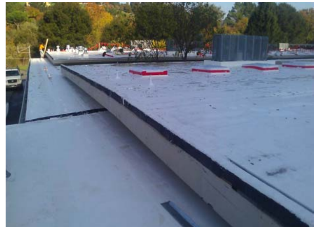
Buildings K & C - Walkway Canopies
