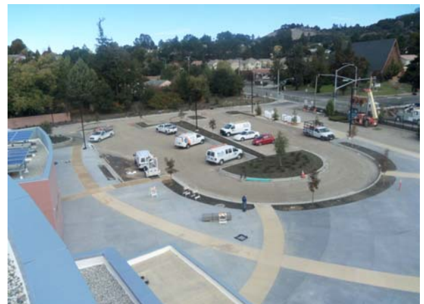
Site Work--Concrete Flatwork
