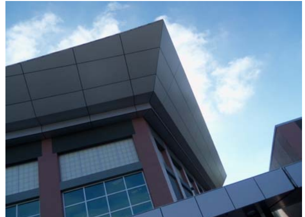
Building No. 8--Gymnasium Canopy Panels
