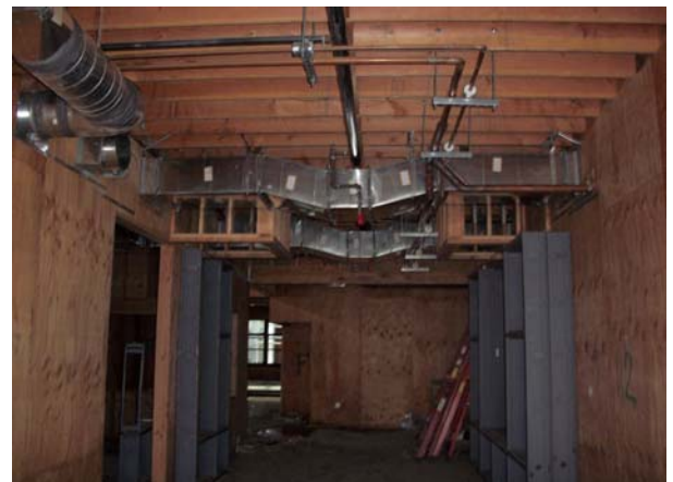
Ductwork in Bldg. A
