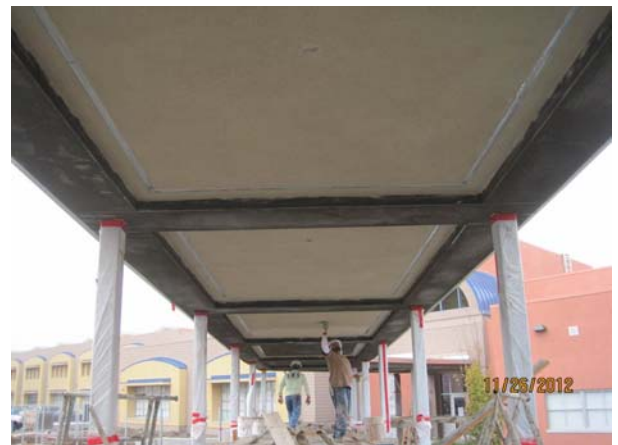
Walkway Canopy Color Coat
