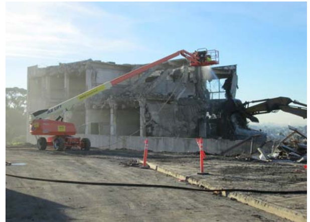
Main Classroom Building- Exterior Demolition
