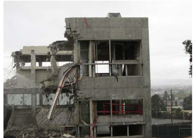
Main Classroom Building- Exterior Demolition
