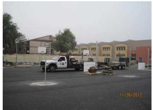
Playground Equipment Install
