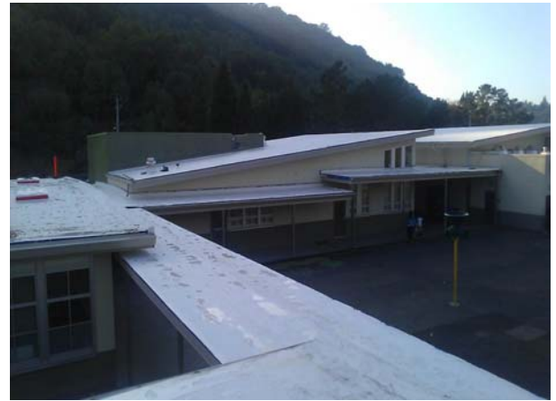
Buildings A & M - Walkway Canopies
