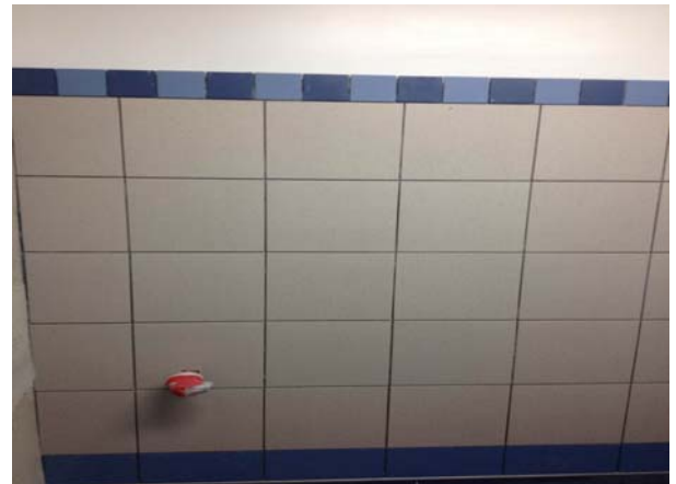
Harding E.S. M104 Restroom Tile Installation
