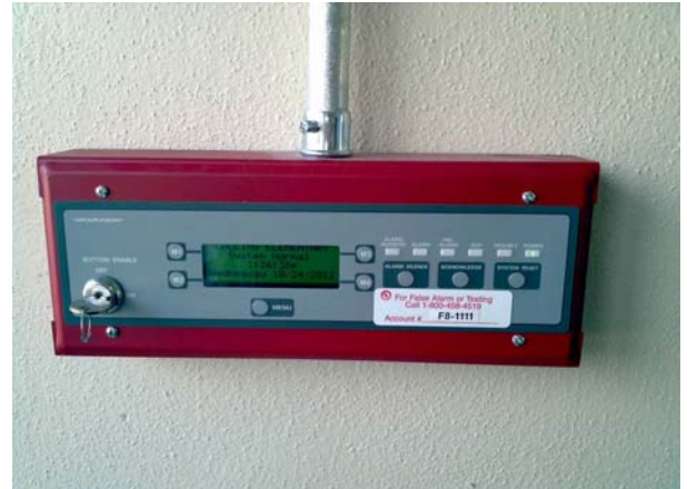
Fire Alarm Control Panel @ Principal's Office
