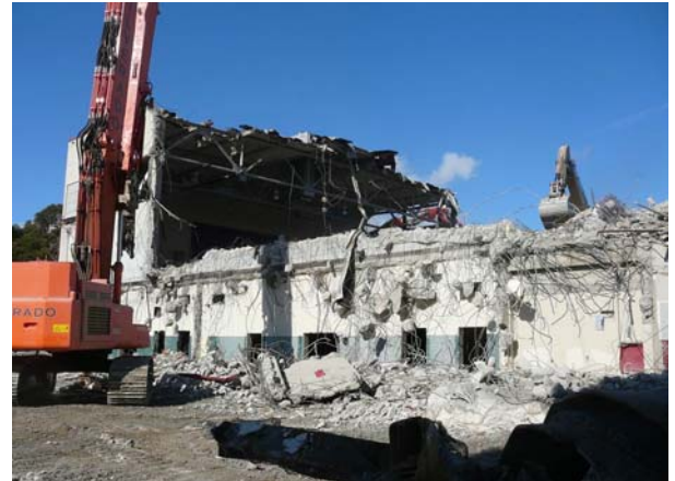
Gym - Exterior Demolition
