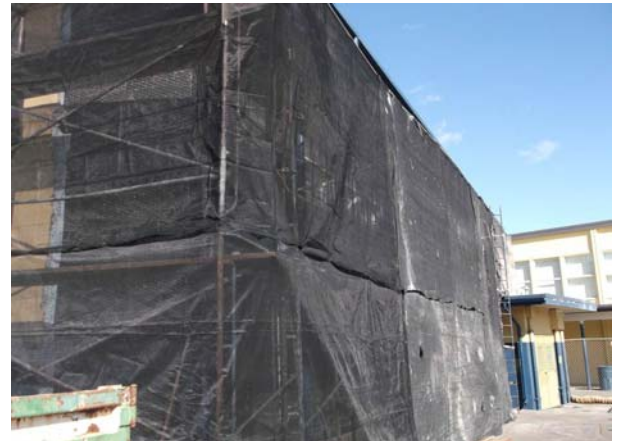
Repair and Paint Stucco Wall-Bldg. E - IN PROGRESS
