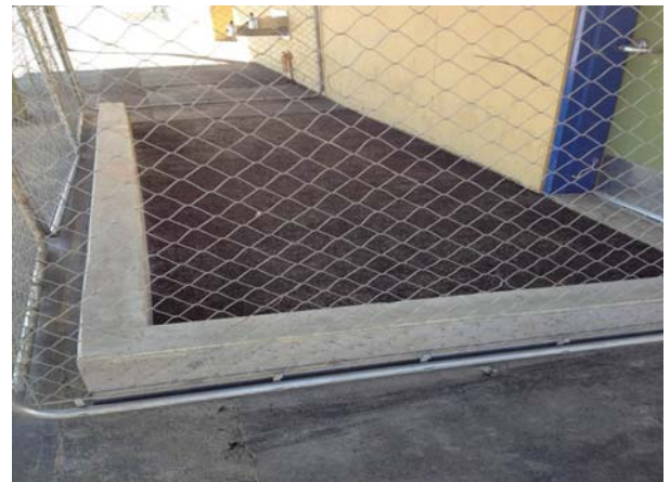
ADA Ramp At Tara Hills E.S.
