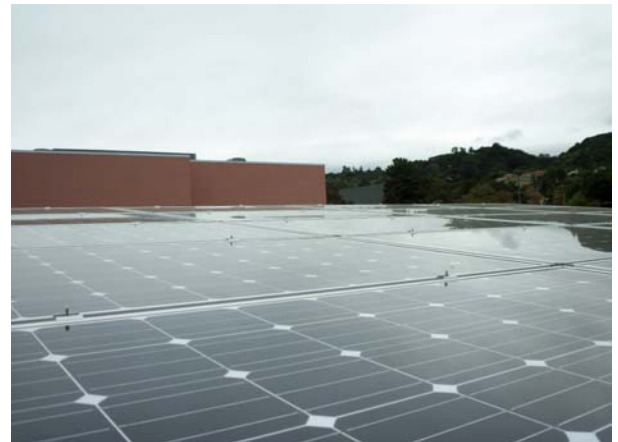
PV System--Install Panels
