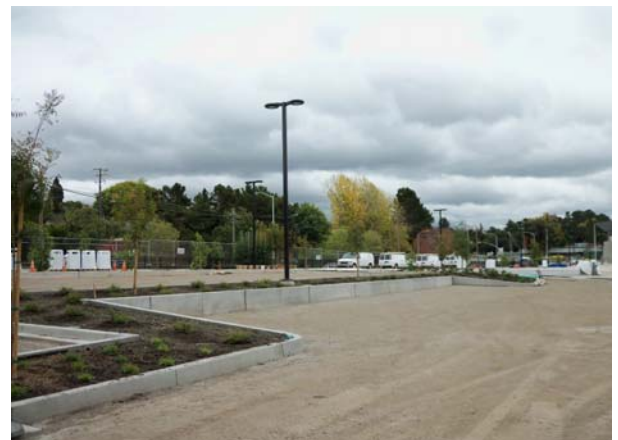
Site Work--North Parking Curb Installation & Landscaping
