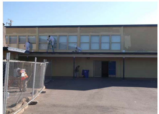
Exterior Painting of Bldg. D - IN PROGRESS
