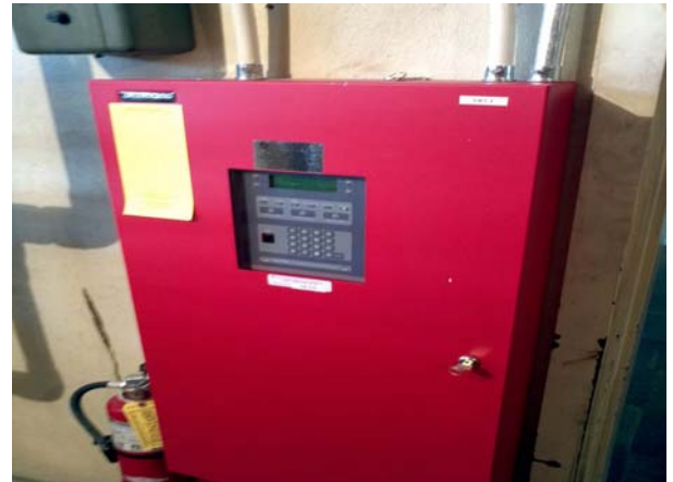
Main Fire Alarm Control Panel
