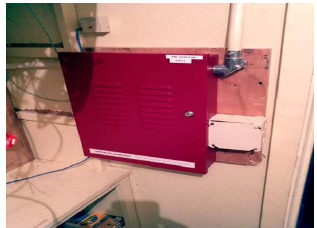
Secondary Fire Alarm Control Panel
