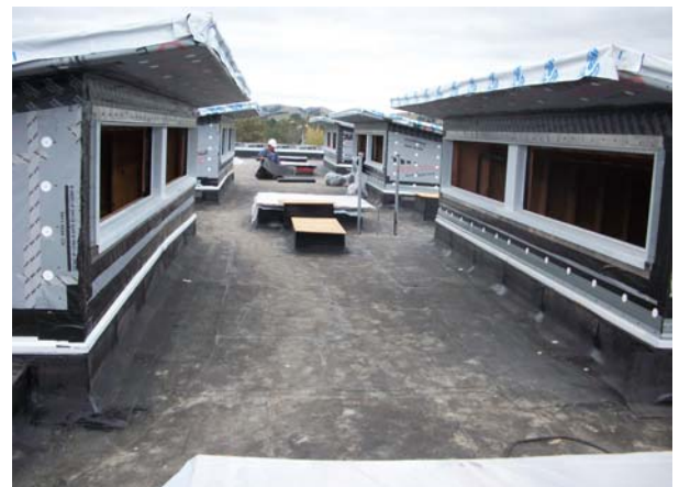
Bituminous Roofing on Bldg. A
