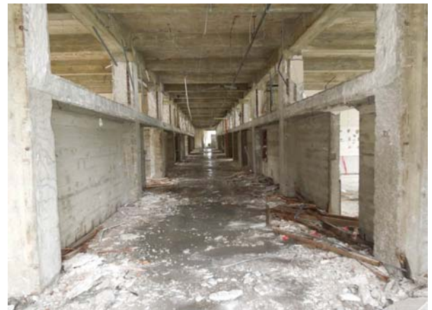
Main Building - Interior Demolition
