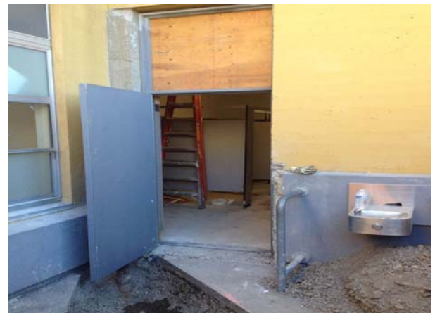
Installed Transom Door At Lincoln Girl's Restroom
