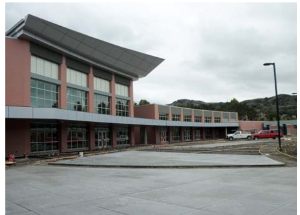
Site Work--Install Concrete Flatwork
