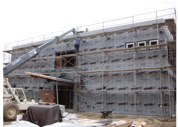
Bldg. A with Metro Wrap installed
