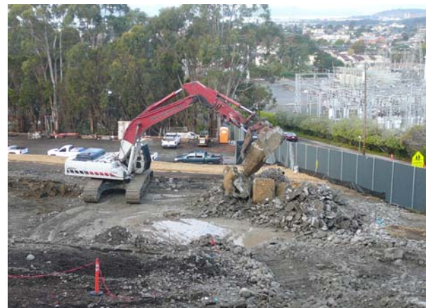
Shop Building - Demolition of Foundation
