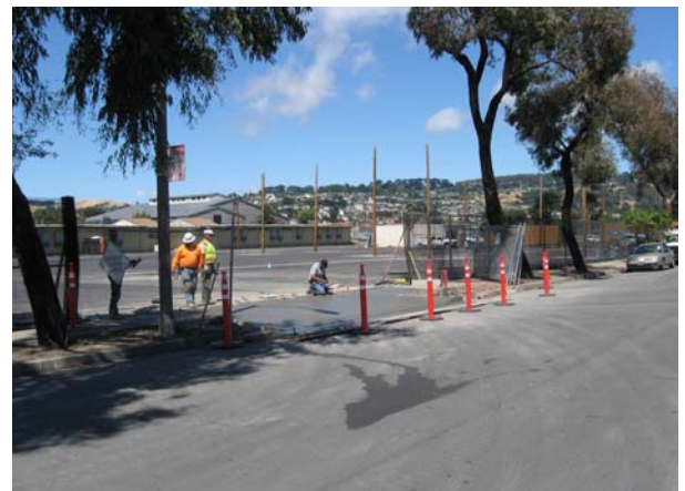
Finishing concrete entry way
