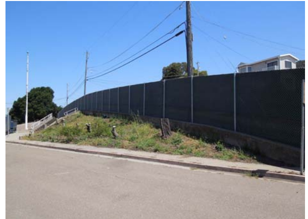
Perimeter Construction Fence Installation Complete
