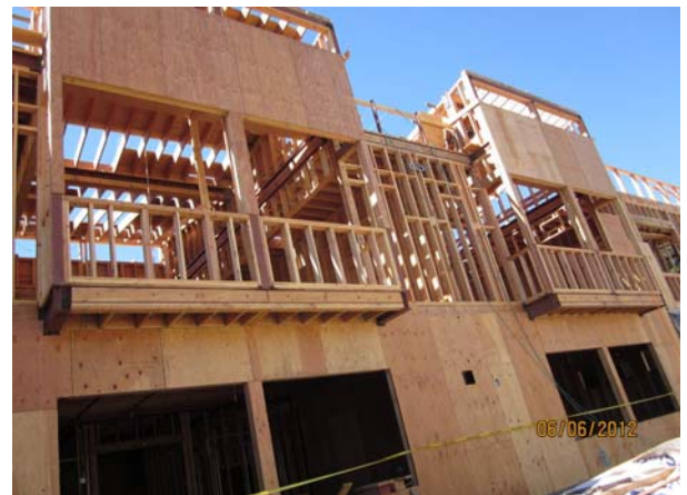
Building A Side 2
