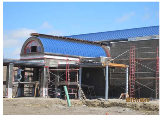
Bldg. C Entrance- Metal Roofing & Plastering
