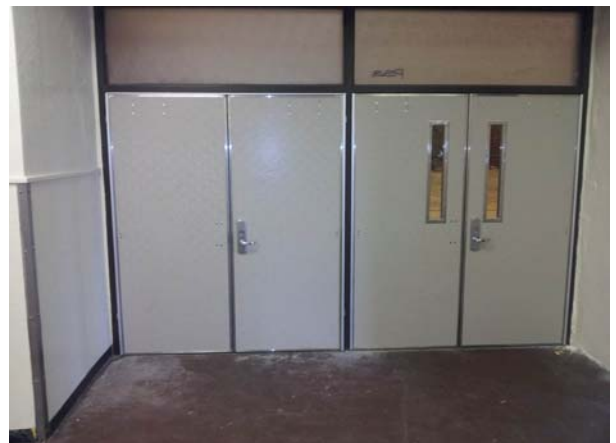
Replacement Door at Northwest Atrium
