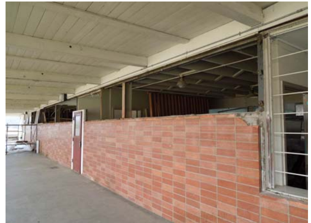
Abatement of Exterior Windows at Shop Building
