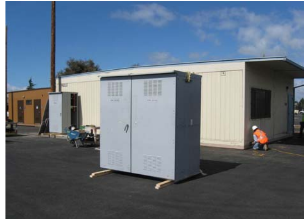
Switch and Electrical Panel
