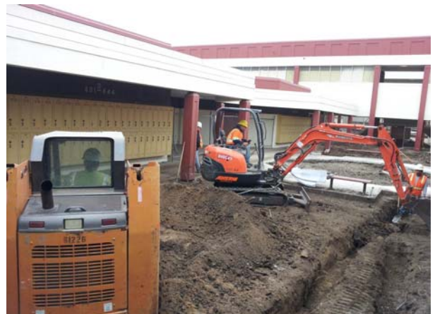
Trenching for Main Water Line
