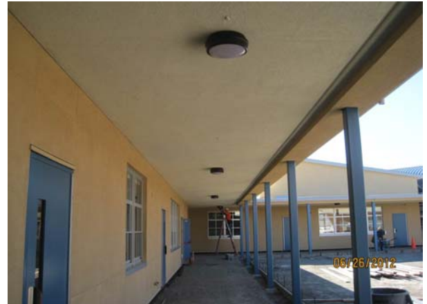
Bldg. B Canopy- Light Fixtures and Site Grading
