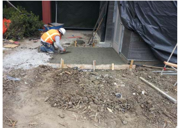
Concrete Paving at Machine Room
