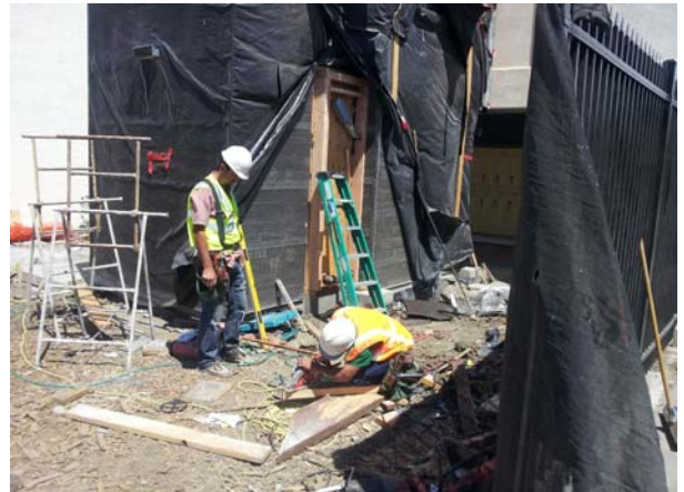
Soffit Framing - Elevator and Machine Room
