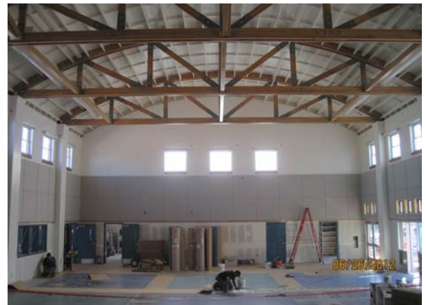
Bldg. C - Resilient Flooring & Wall Panels
