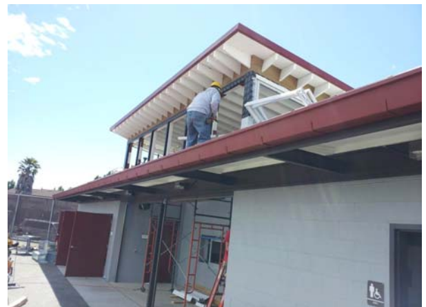
Stand - Exterior Clerestory Window Flashing
