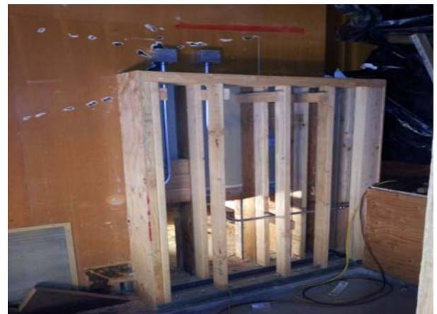
ADA-Multipurpose Room Conduit and Framing
