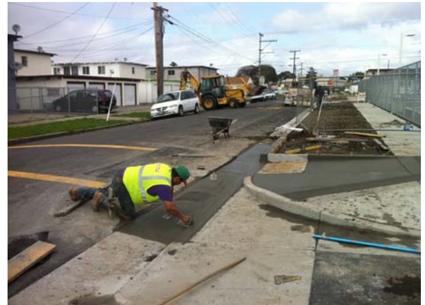
Install of Access Ramps at 39th Street Driveway
