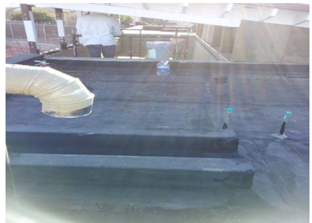
Painting and Built-Up Roofing
