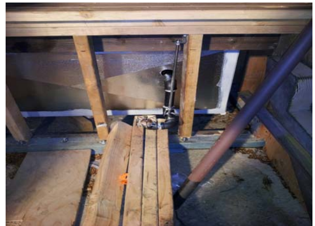
ADA - Re-Routed Sprinkler Line
