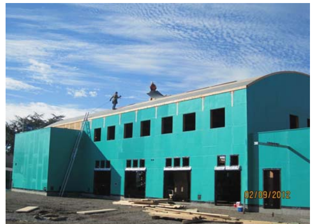
Building C - Barrel Roofing
