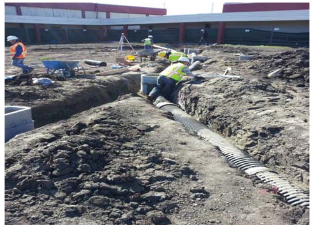
Quads Upgrade - Install Trench Drain
