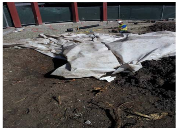
Quads Upgrade - Install Catch Basin
