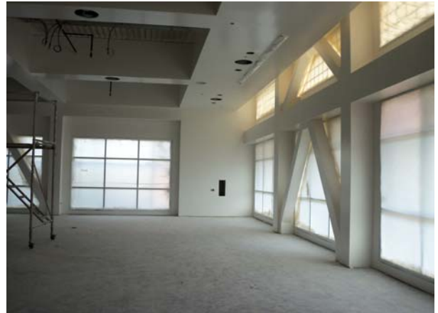
Building 1: Interior Finish Work
