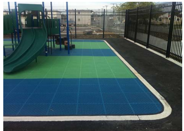
Completed Kindergarten Play Structure
