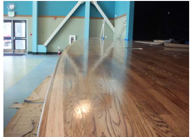
Wood Floors at stage in Multi-Purpose Room
