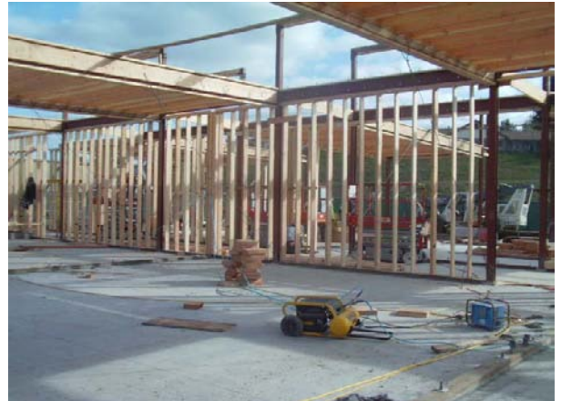
Rough Framing at Building B
