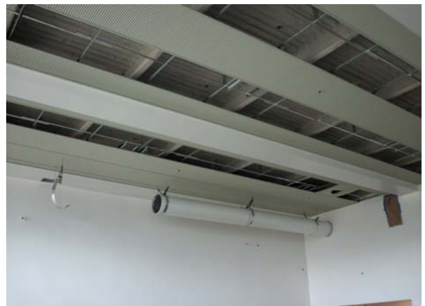
Building 9: Install HVAC Ducts & Ceiling
