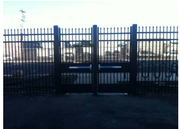
Fence and Gates at Kindergarten Play Yard
