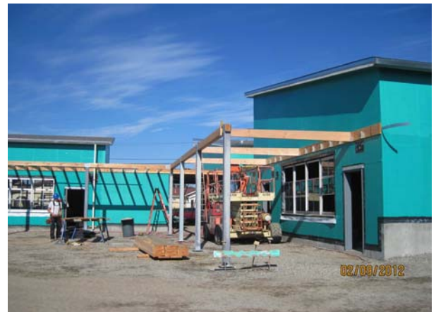
Building B - Covered Walkway Framing
