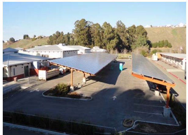
Parking Lot B - Arrays #2 & #3 Roofs
