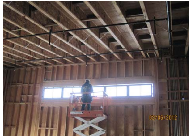
Building B - Window Frame and Glazing
