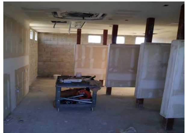
Concession Stand - Women's Restroom
