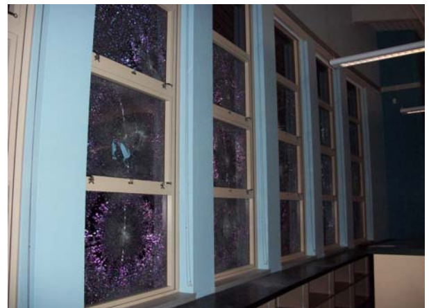
Vandalism- Broken windows in Library
