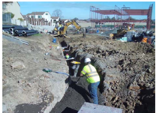
Installing Underground Domestic Water Line
