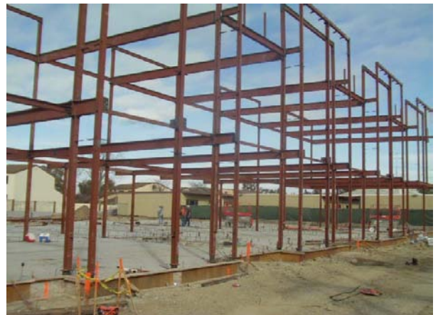
Structural Steel Erection at Building A
