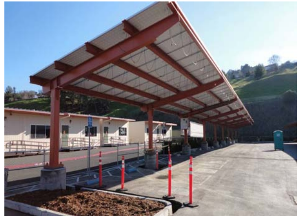
Parking Lot B = Array #2
