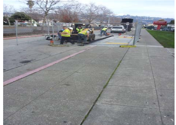
ADA Asphalt Patching
