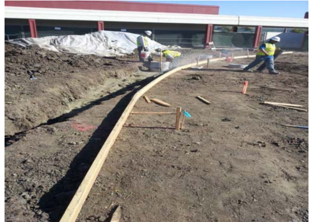
Quads Upgrade - Trench Drain Forming
