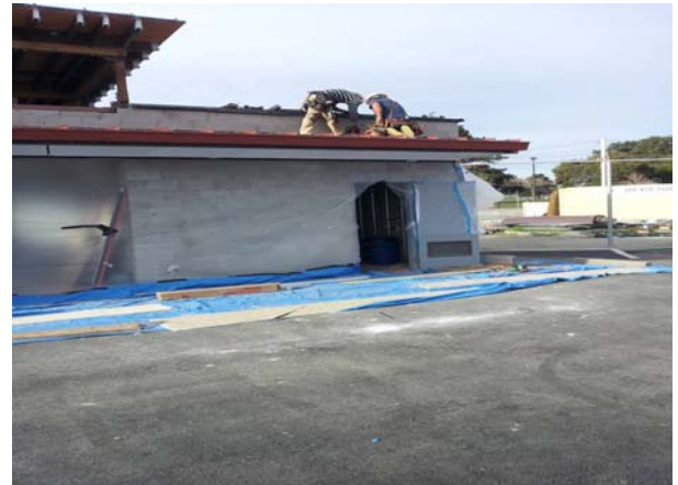
Concession Stand- Install Canopy Roofing
