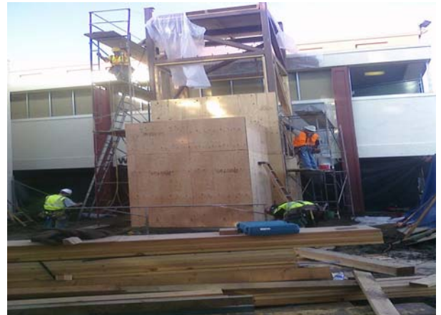
Elevator Framing
